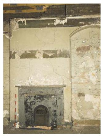
Plate 3: Chimney breast in west wall of Room CFO1F3 and stepping of flue above arched recess
