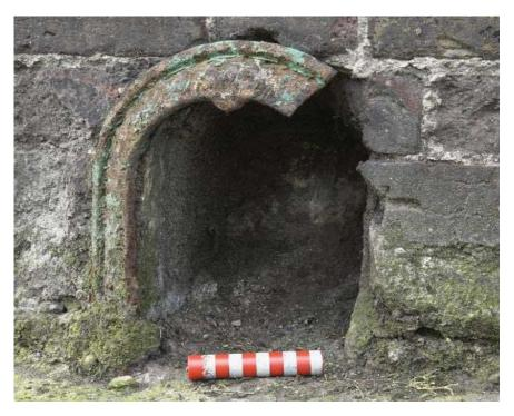
Plate 8: Remains of cast iron boot scraper inserted into the base of the north wall of Block 2 (Figures 11 and 31)
