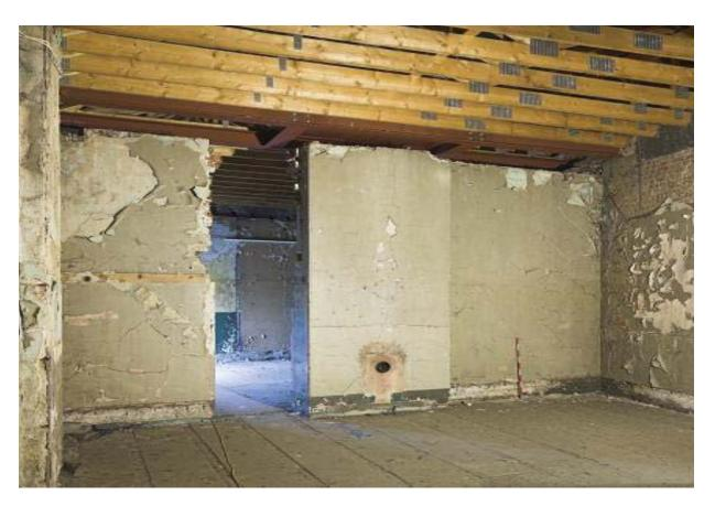
Plate 20: Chimney breast in Room CFO4G2 with steel beams supporting chimney stack above
