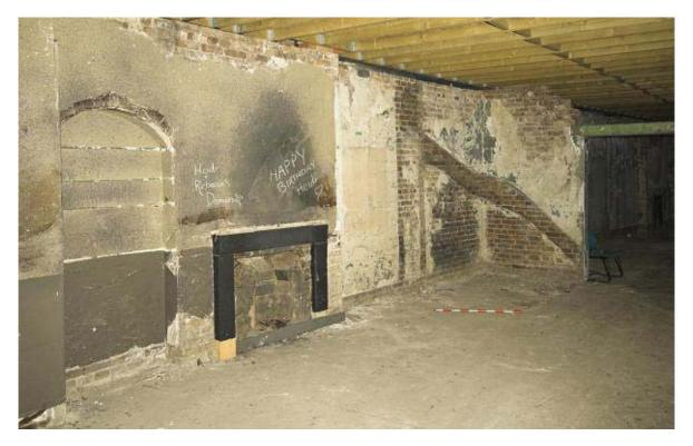
Plate 23: Arched recess, fireplace and stairwell scar in south wall of Room CFO5G1
