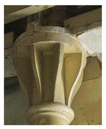
Plate 16: Column head and detail of joint with column above (Figure 28)
