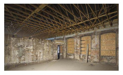
Plate 11: Timber battened and gangnailed roof trusses above Room CFO2S1
