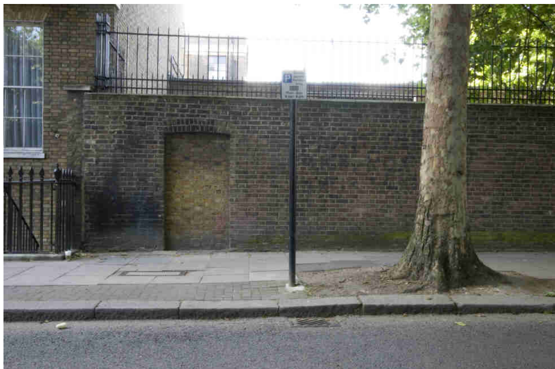
Plate 2 Infilled doorway in north elevation of boundary wall
