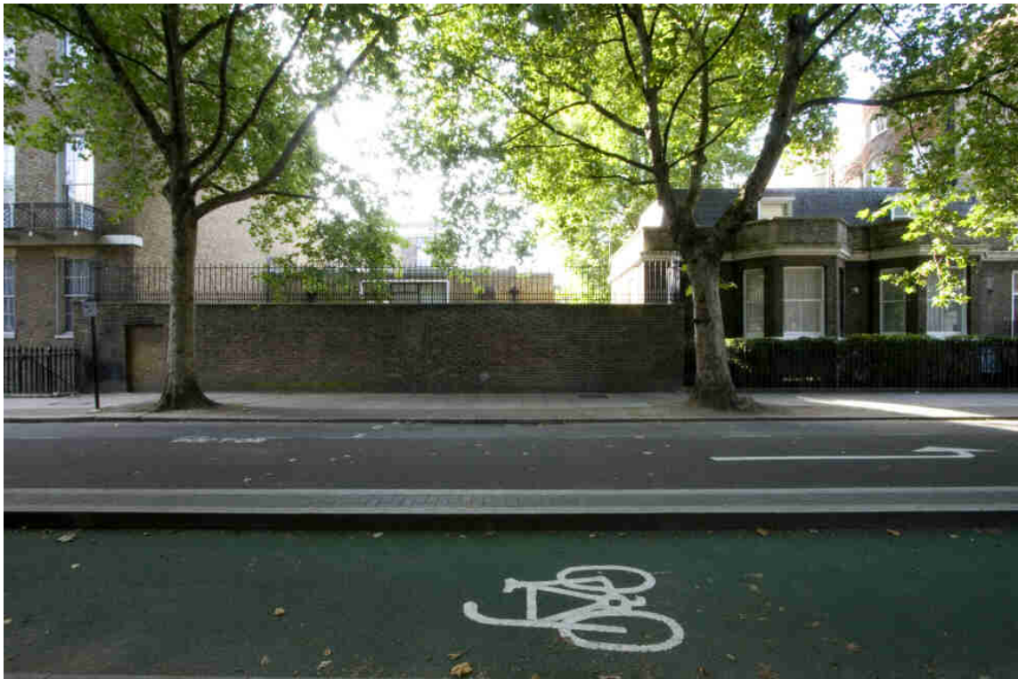
Plate 1 North elevation of boundary wall
