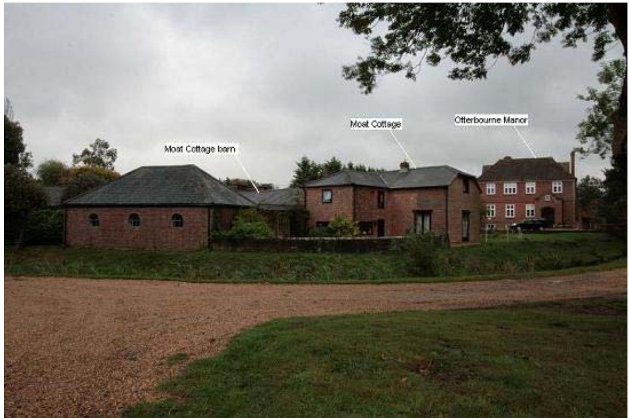
Plate 1: Moat Cottage barn, Moat Cottage and Otterbourne Manor viewed from the southwest (PCA)
