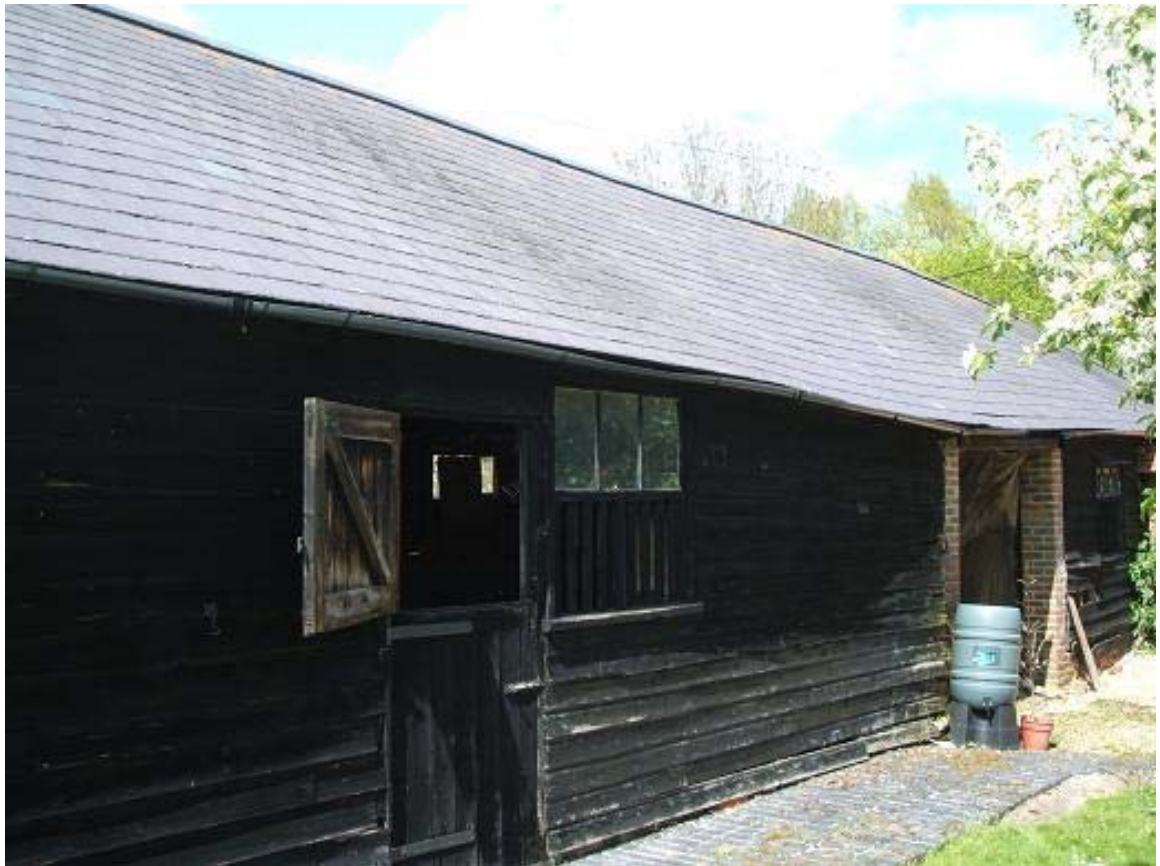
Plate 14: South-east elevation (RG)
