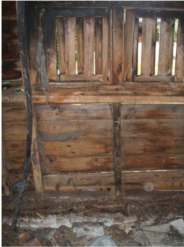
Plate 11: Studwork and window in south-east elevation (RG)
