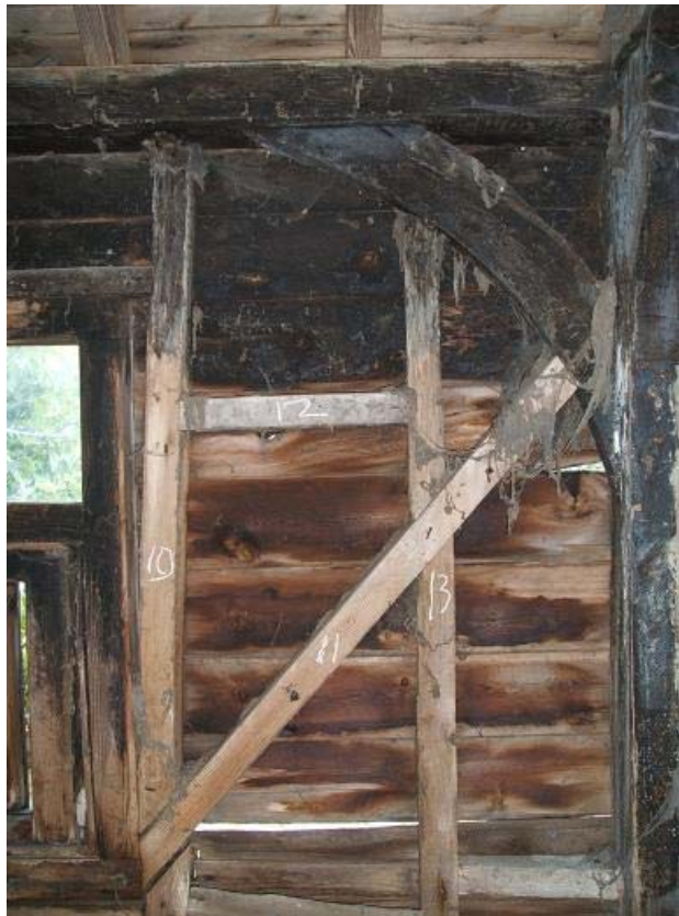
Plate 12: Studwork in south-east elevation (RG)
