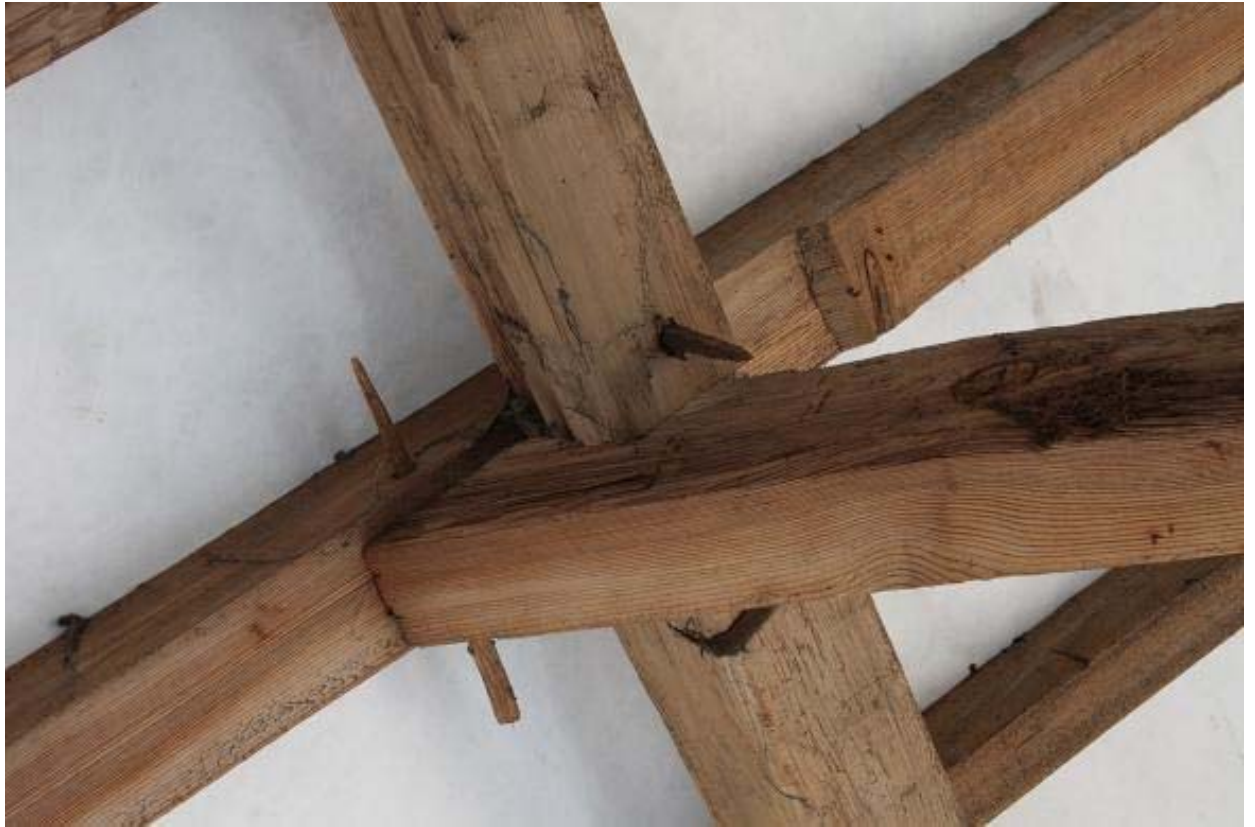
Plate 5: Trenched purlin viewed from the north-east (PCA)
