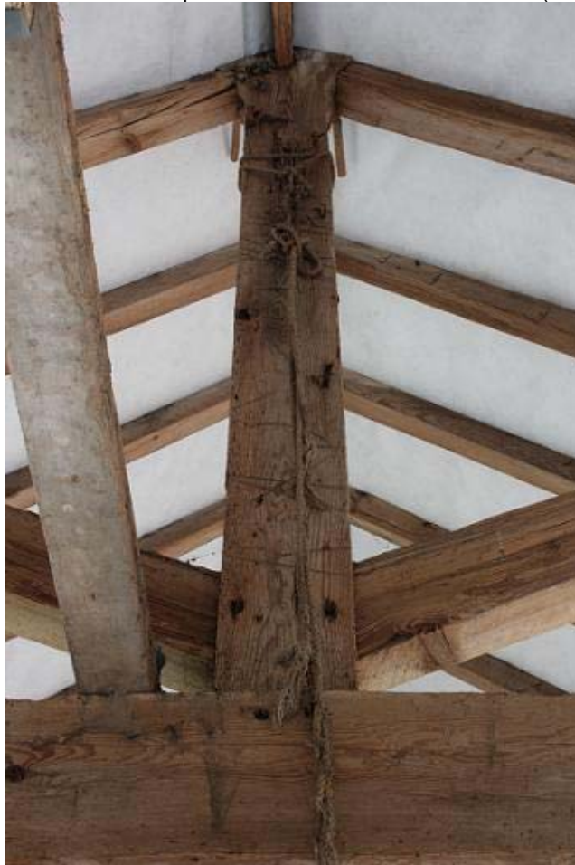
Plate 6: Carpentry marks on central king post viewed from the north-east (PCA)
