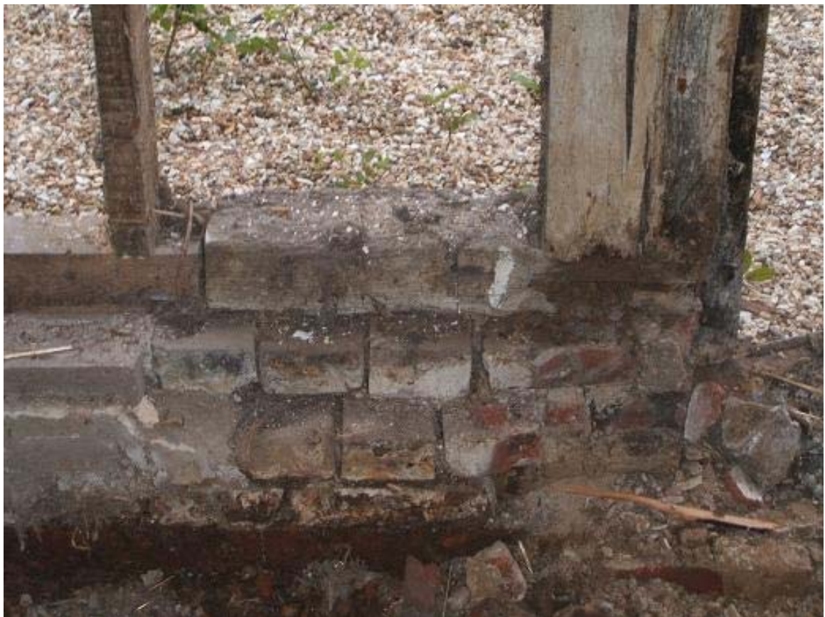
Plate 10: Brick sill and timber sole plate viewed from the north-west (RG)
