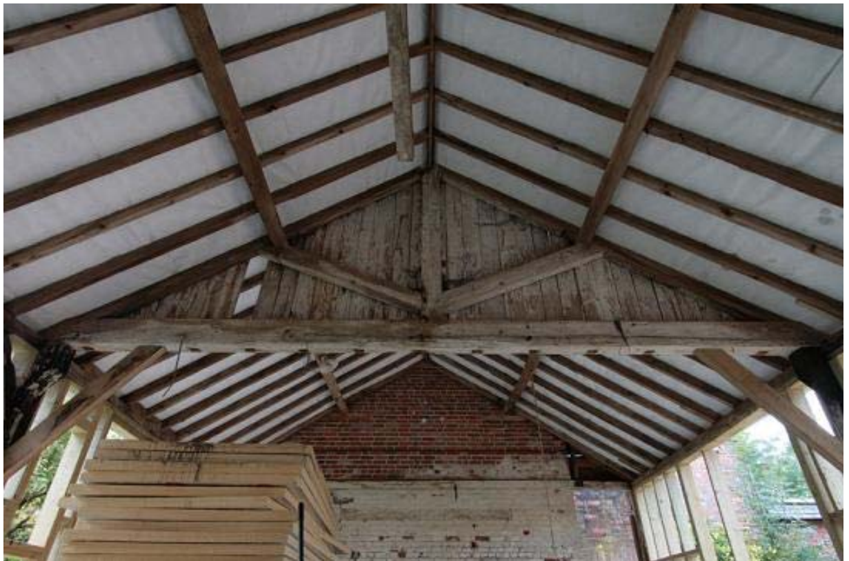
Plate 4: King post truss with wood cladding, viewed from the north-east (PCA)
