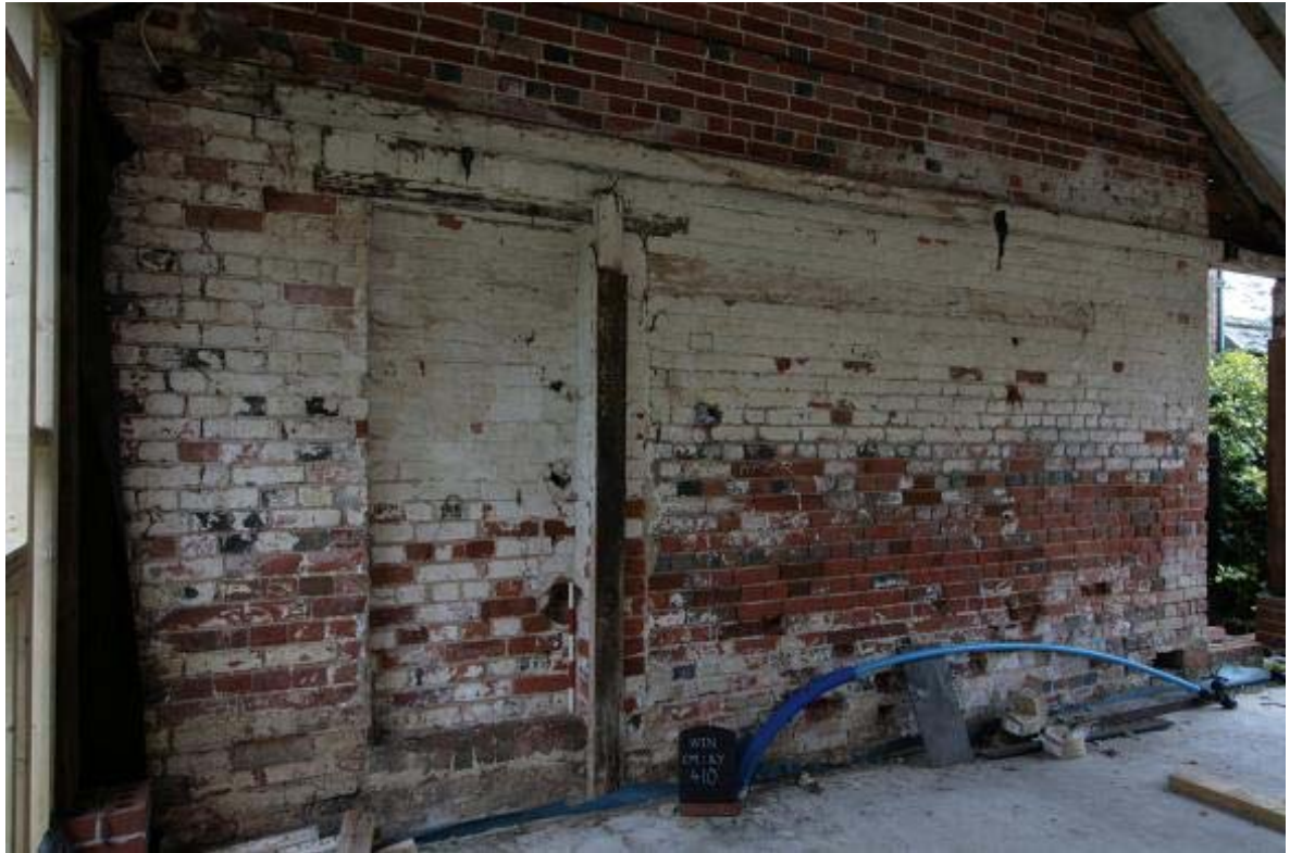
Plate 3: North-east wall of Moat Cottage (PCA)
