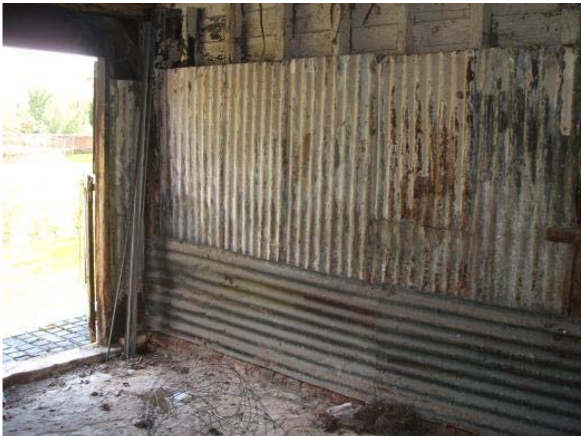
Plate 18: Corrugated metal sheets covering internal partition wall (RG)
