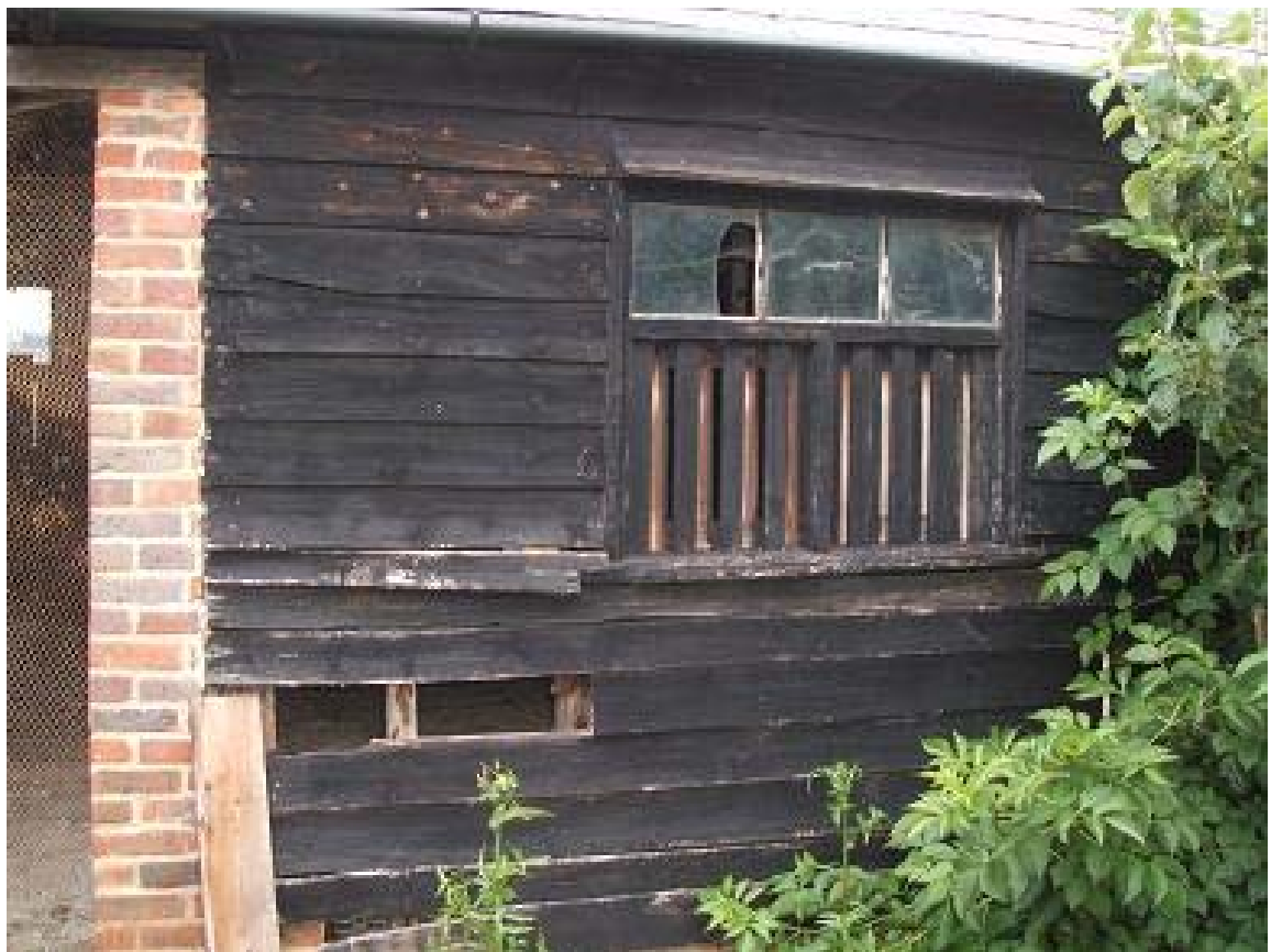
Plate 16: North-east end of the south-east elevation (RG)
