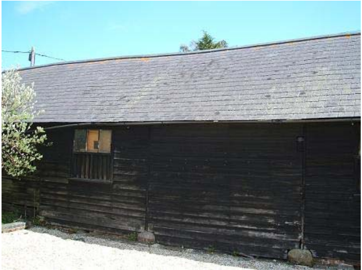
Plate 9: North-west elevation (RG)
