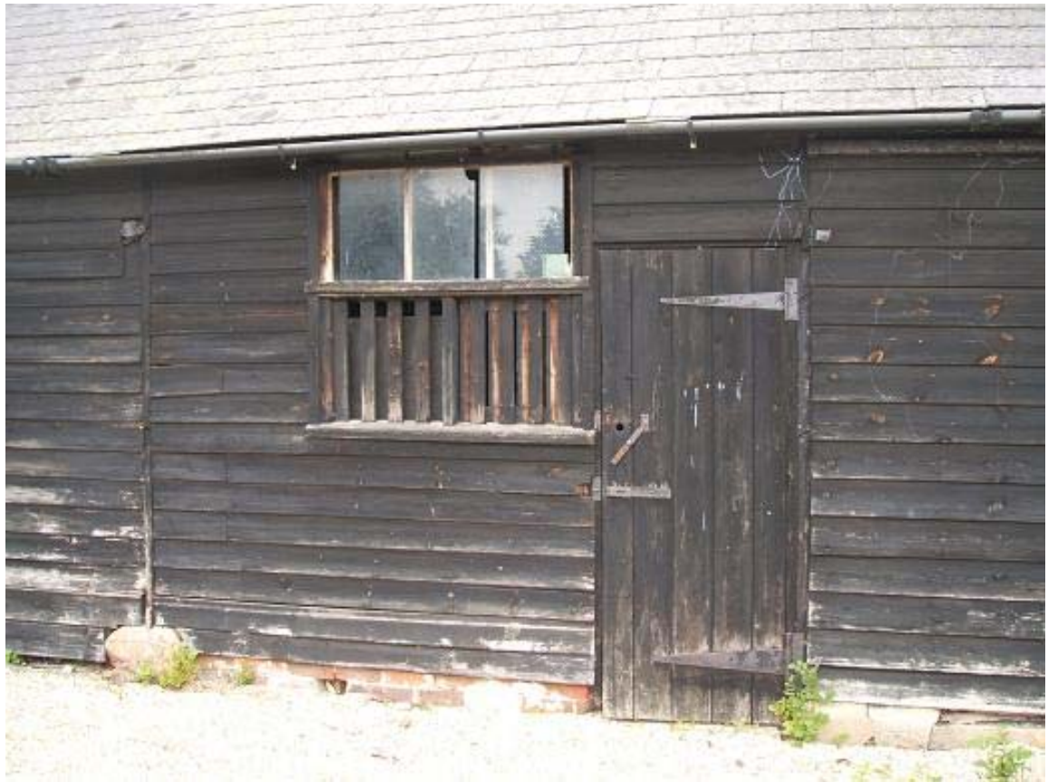
Plate 15: North-west elevation (RG)
