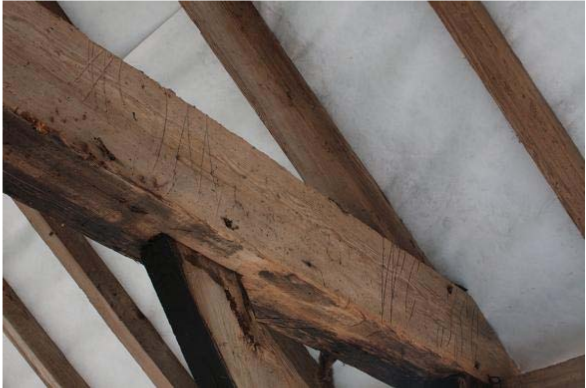
Plate 7: Carpentry marks on tie beam viewed from the north-east (PCA)
