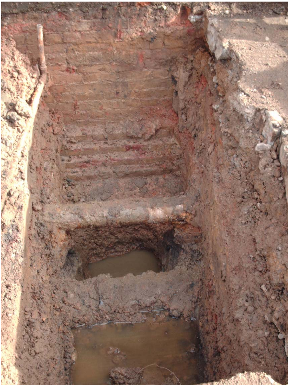
Plate 2: Test Pit 2 view from the west showing stepped foundation of the Midland Goods Shed
