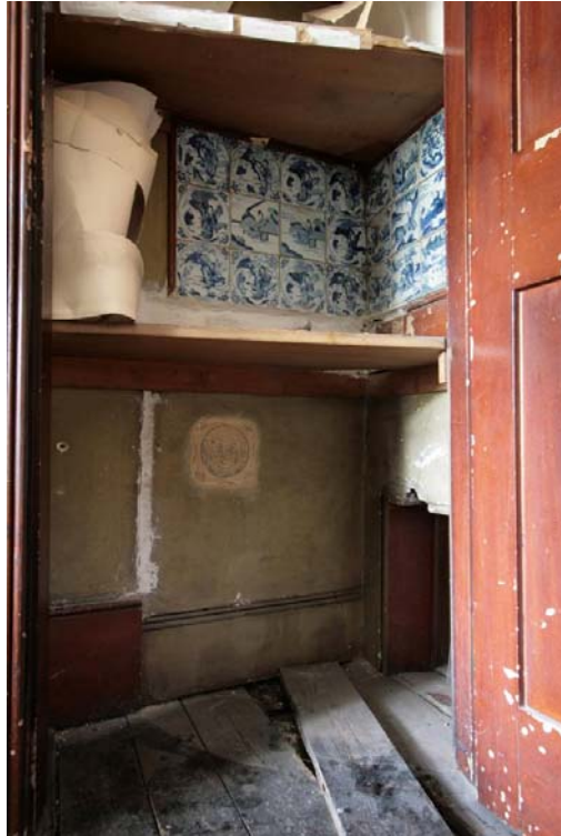
Plate 10 Second Floor, cupboard in north-west corner of Mrs Soane's Morning Room, west wall (PCA)
