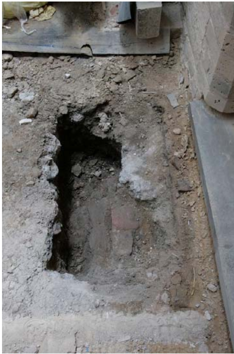
Plate 1 Basement New Court Trial Pit NC/OU1, view from the east (PCA)
