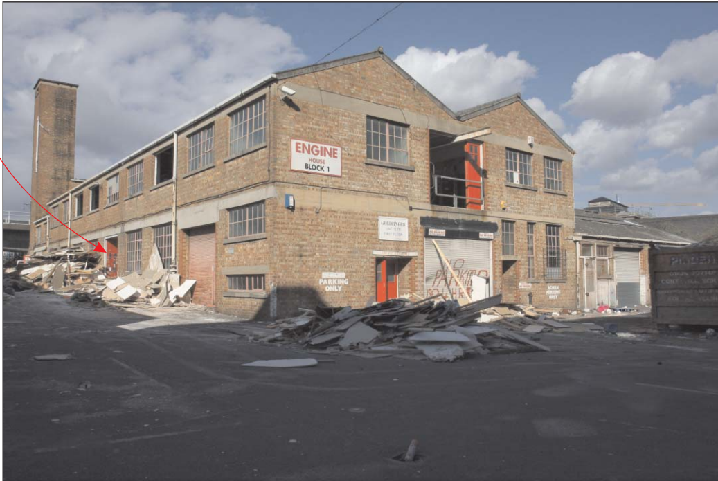
Plate 1: South and west elevation of the Engine House
