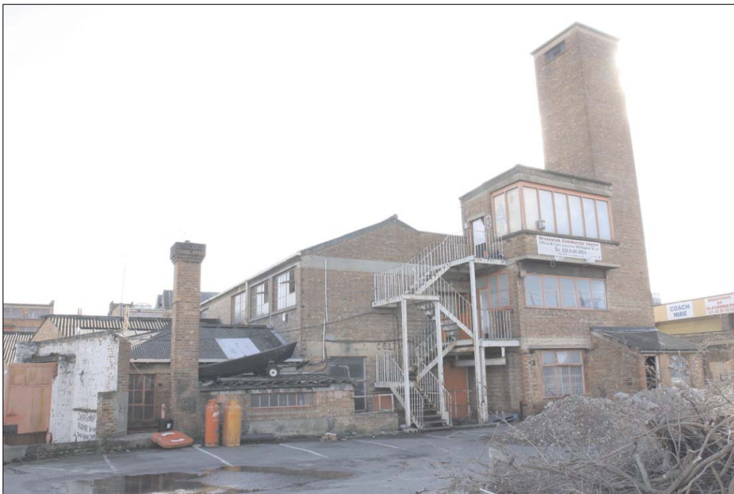
Plate 2: North elevation of the Engine House
