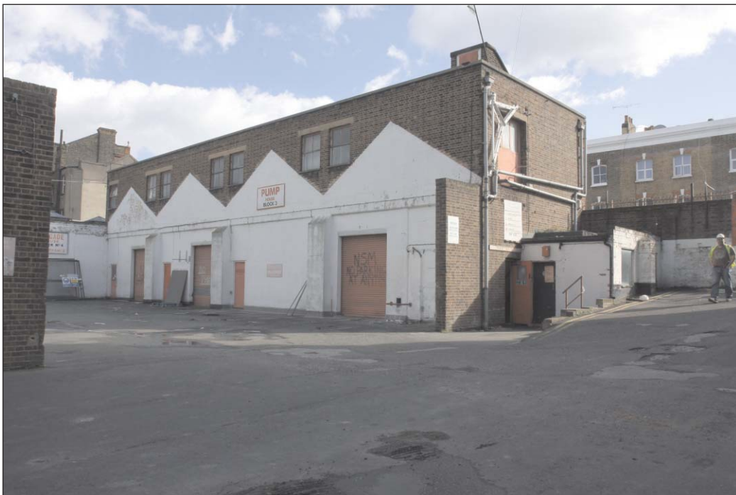
Plate 10: North and west elevations of the Pump House
