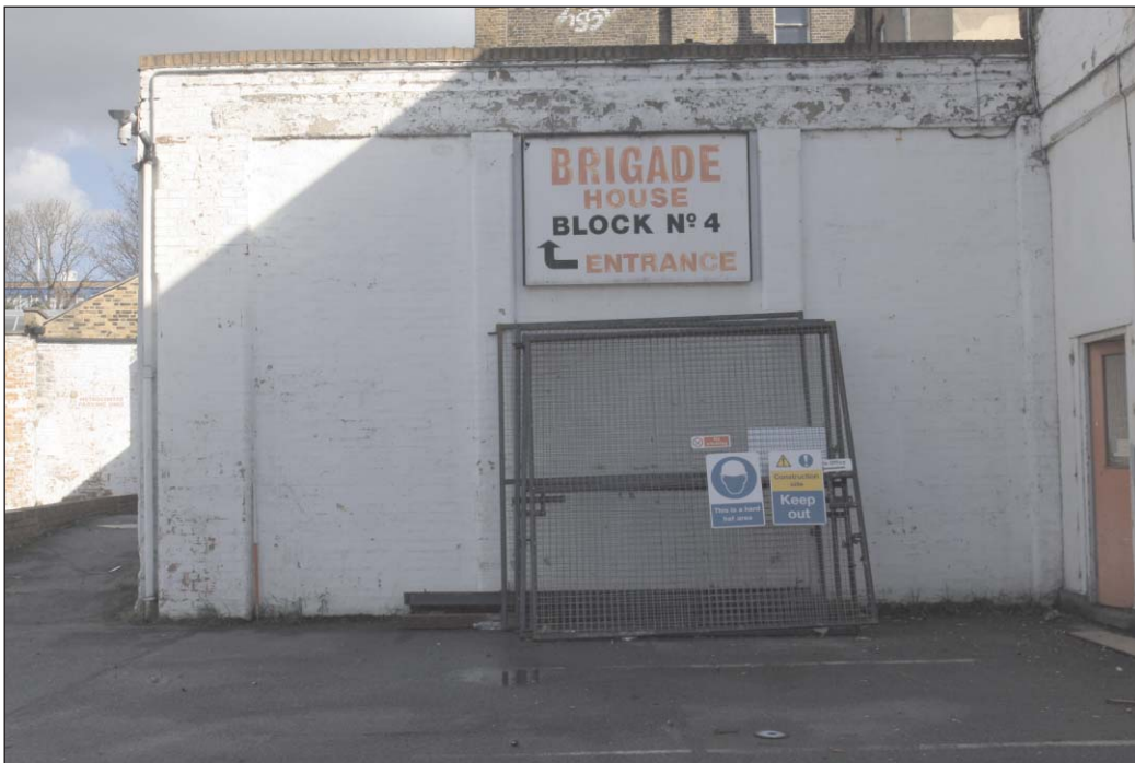
Plate 14: West wall of Brigade House
