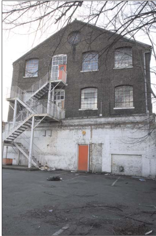
Plate 7: East elevation of the Station House
