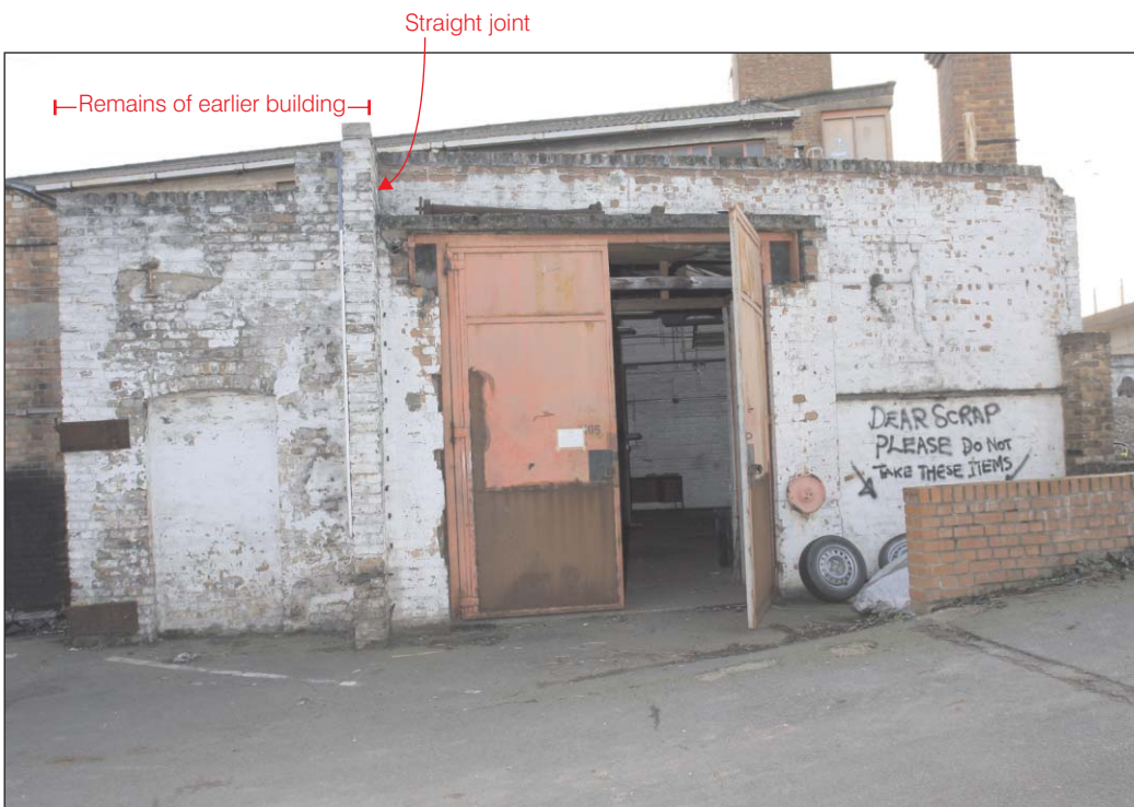
Plate 4: Remains of 19th century building incorporated within the Engine House
