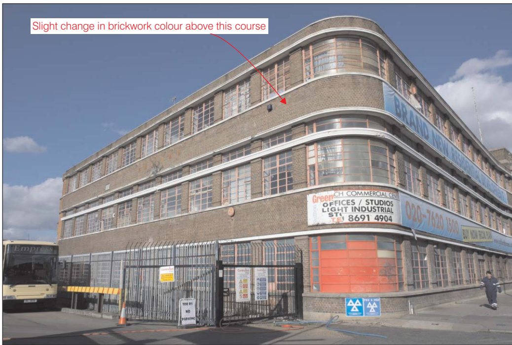
Plate 18: West elevation of Bell House
