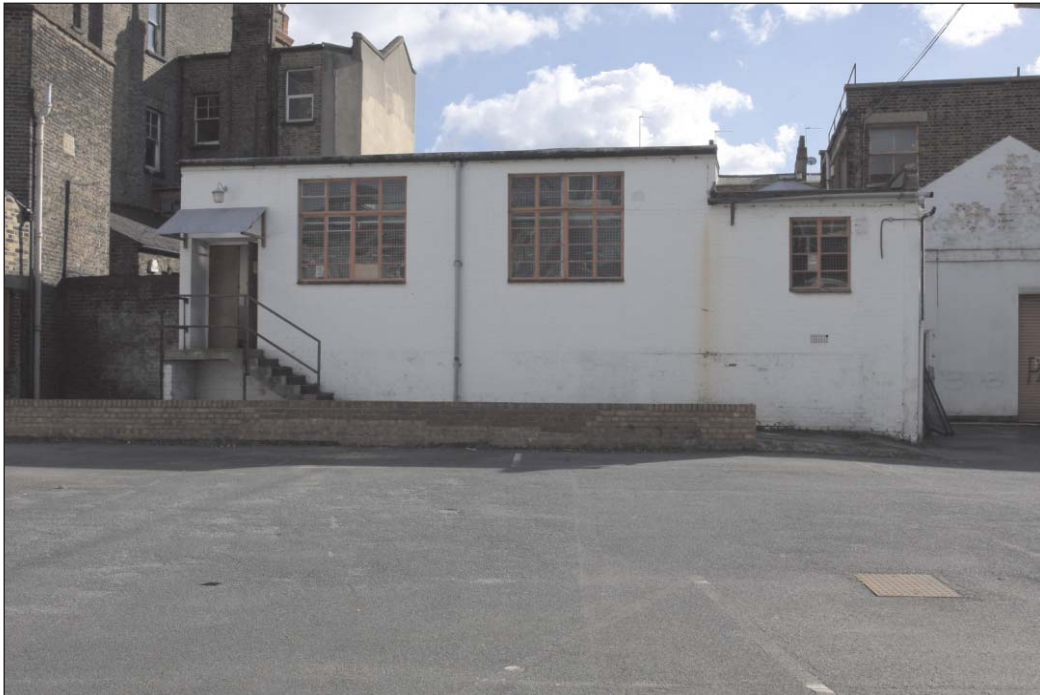
Plate 12: North elevation of Brigade House
