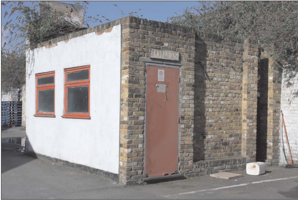
Plate 23: West and south wall of Toilet Block 8
