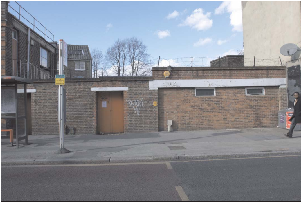
Plate 13: South wall of Brigade House
