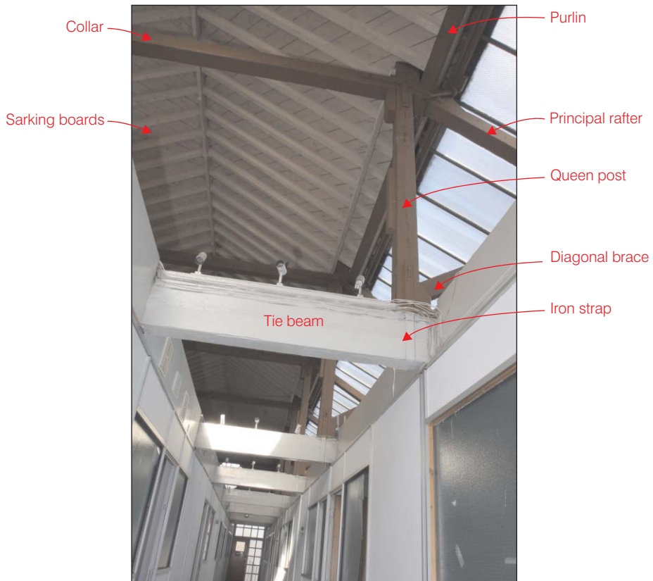
Plate 8: Queen post truss roof in the Station House
