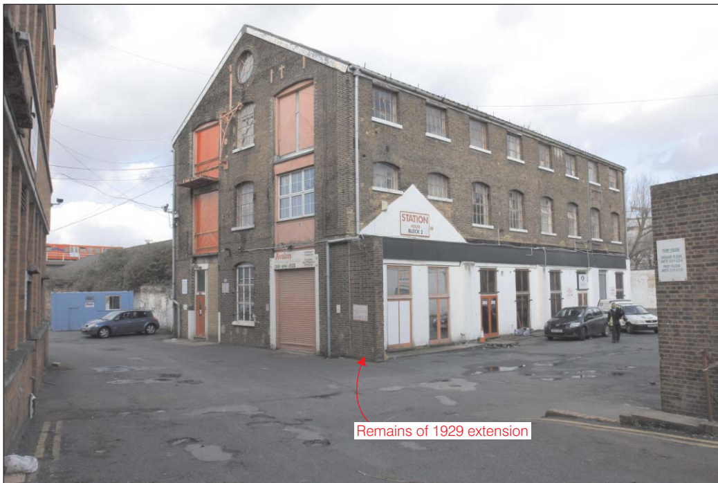
Plate 6: West and south elevations of the Station House
