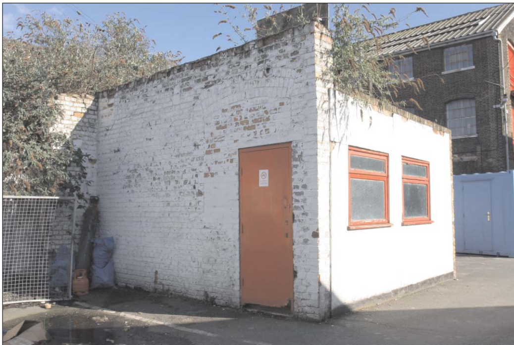
Plate 22: North and west wall of Toilet Block 8
