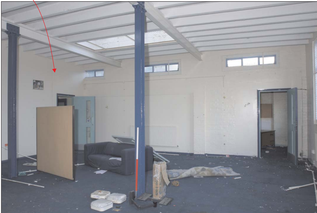
Plate 15: Interior of the canteen in the Brigade House
