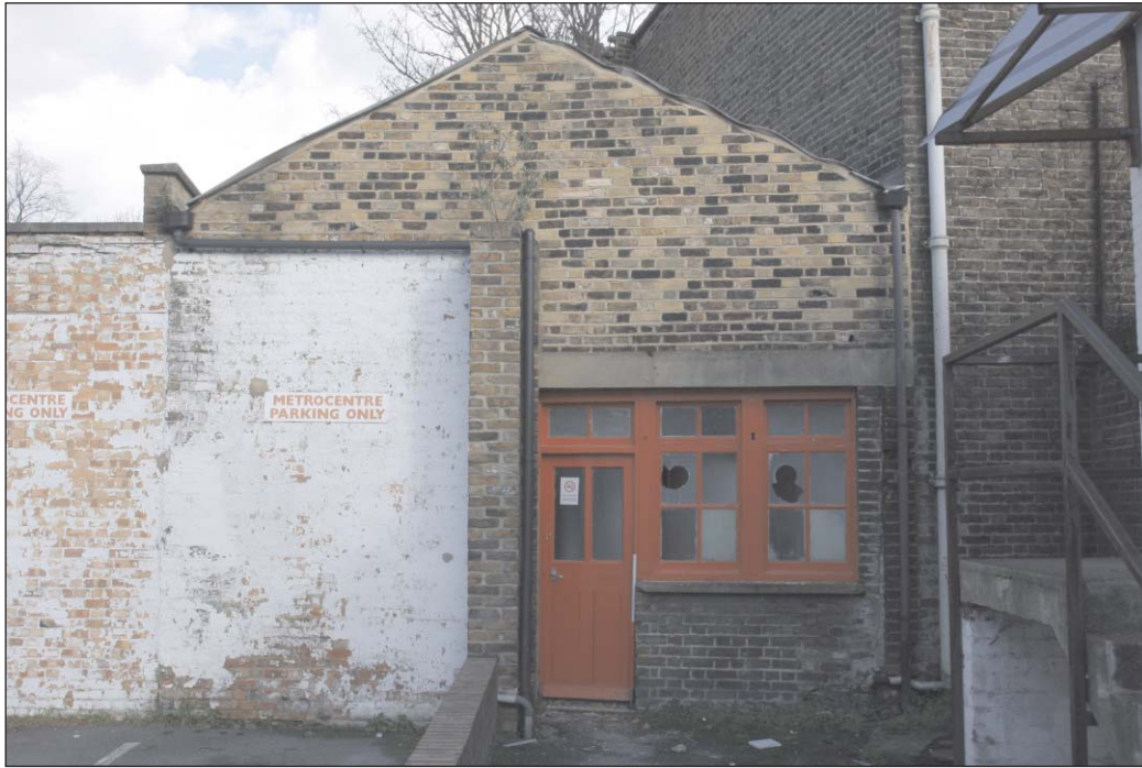
Plate 21: West wall of Toilet Block 7
