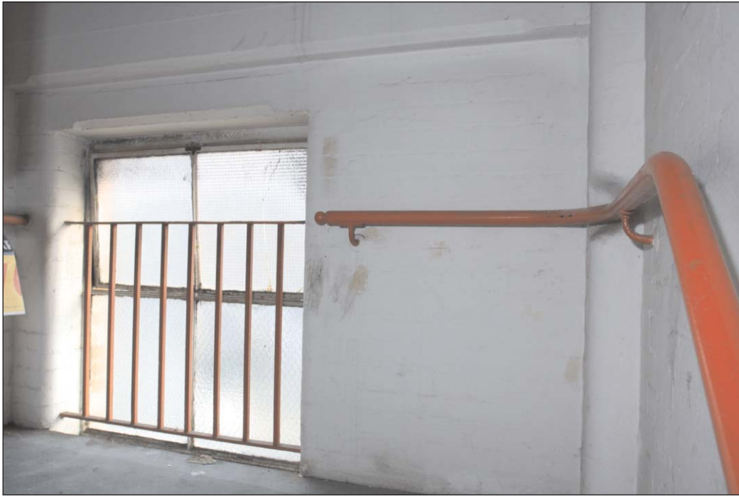
Plate 11: Metal staircase rail in the Pump House
