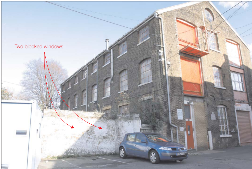
Plate 5: North and west elevations of the Station House
