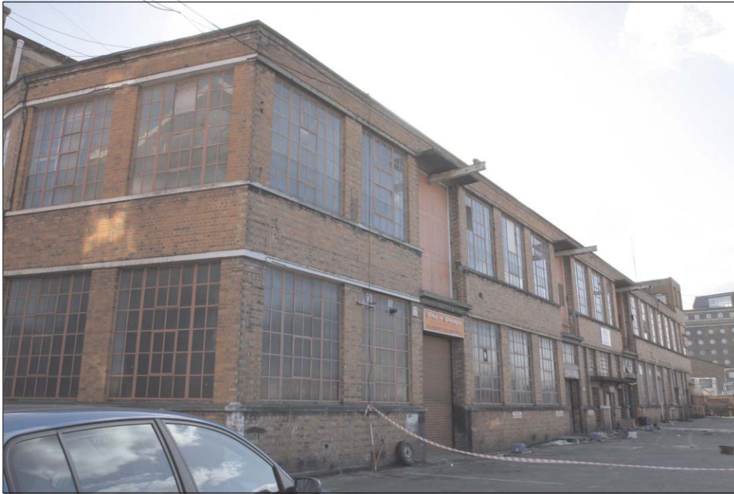
Plate 19: East and north elevation of Bell House and Siren House
