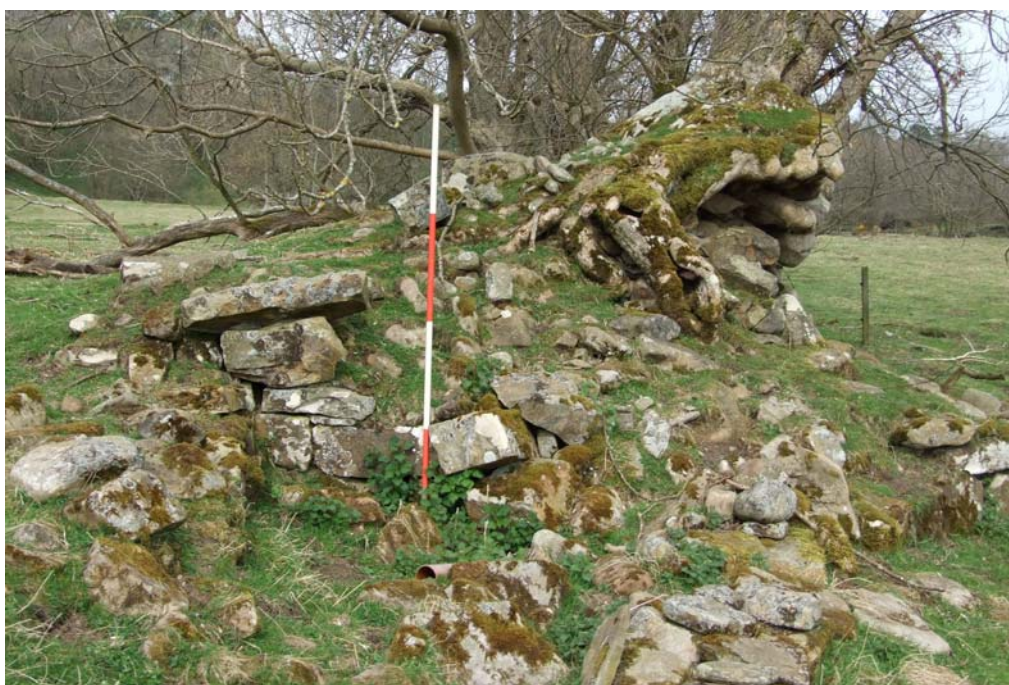
Figure 4: Roman bridge abutment, south side, looking north-west ( scale 2m ).
