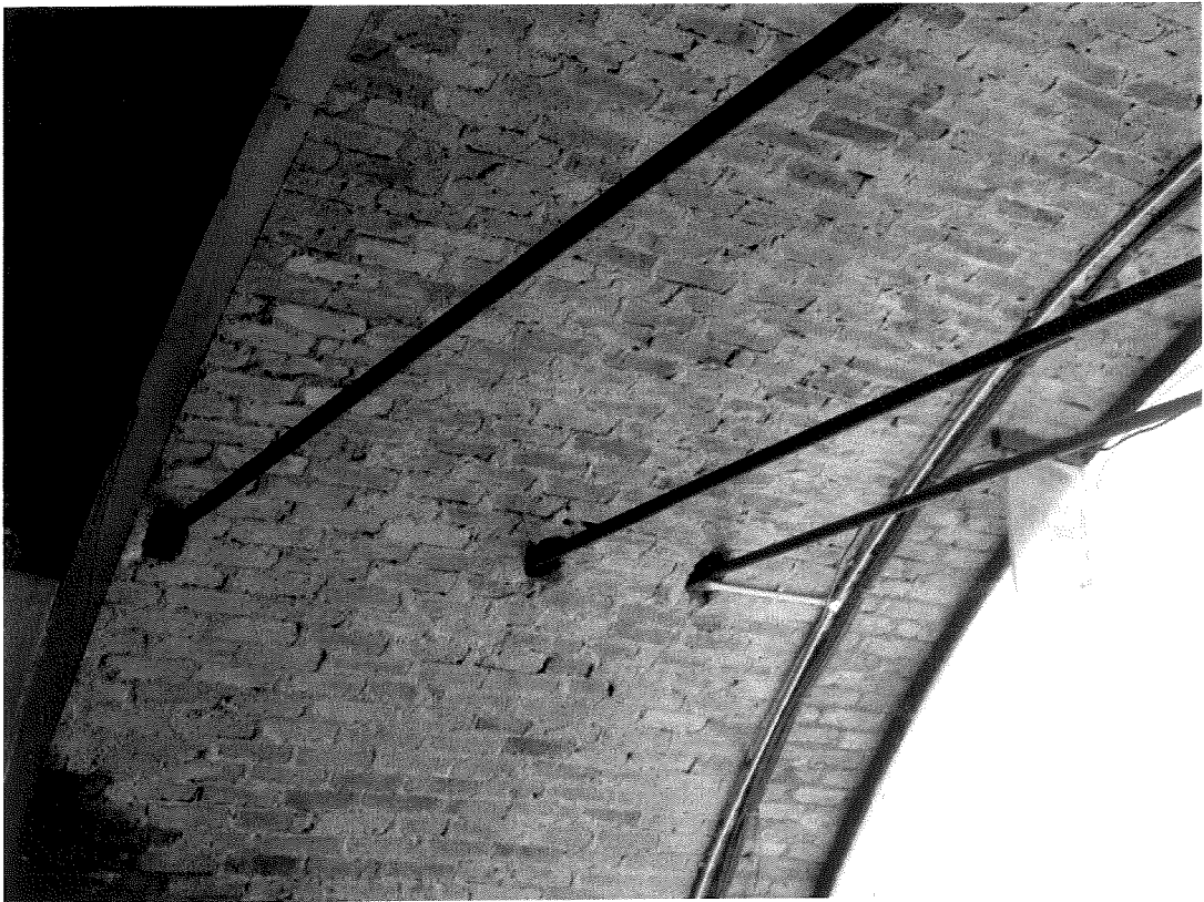
Plate 5: The system of steel tie rods
