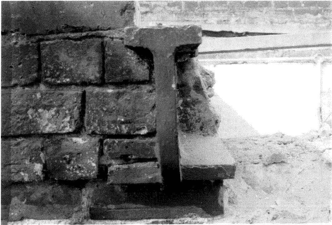
Plate 4: One of the ends of the cast iron beams
