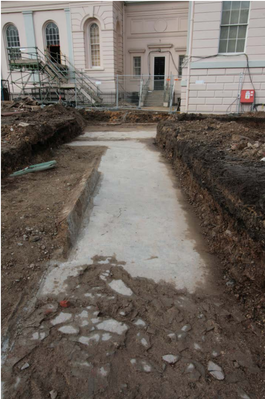
PLATE 7: THE POOL BASE WITH THE NORTHERN WALL (JUST UNDER THE FENCING IN THE BACKGROUND). NOTICE TO THE LEFT THE AREA OF THE ISLAND AND THE BASE OF THE BRIDGE, LOOKING NORTH
