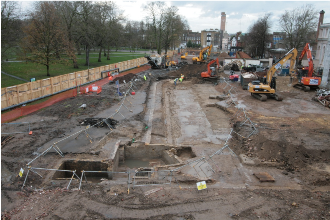
PLATE 3: OVERVIEW OF THE SOUTHERN PART OF THE POOL, LOOKING WEST
