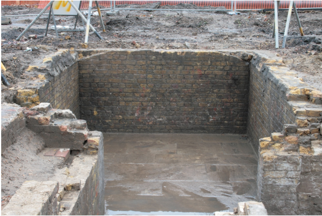
PLATE 5: DETAILED OF VAULTING OF SUBTERRANEAN ROOM ADJACENT TO PUMP ROOM, LOOKING SOUTH
