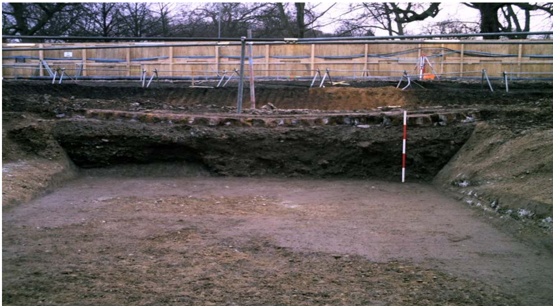
PLATE 6: THE DEEP END OF THE ORIGINAL 1833 POOL, BACKFILLED AND CAPPED WITH BRICKWORK AND RENDER IN 1839, LOOKING SOUTH
