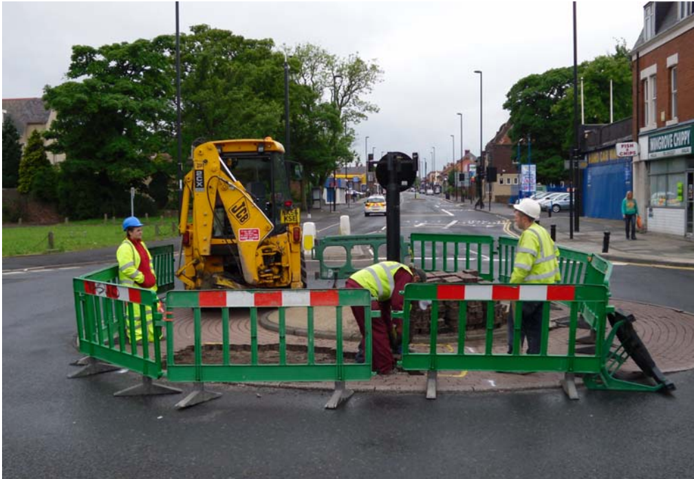
Plate 3: Trench 2, Trench Preparation
