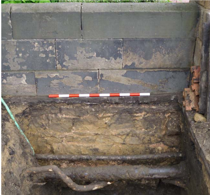
Plate 5: Trench 3, Wall Foundation [325] (scale 1m)
