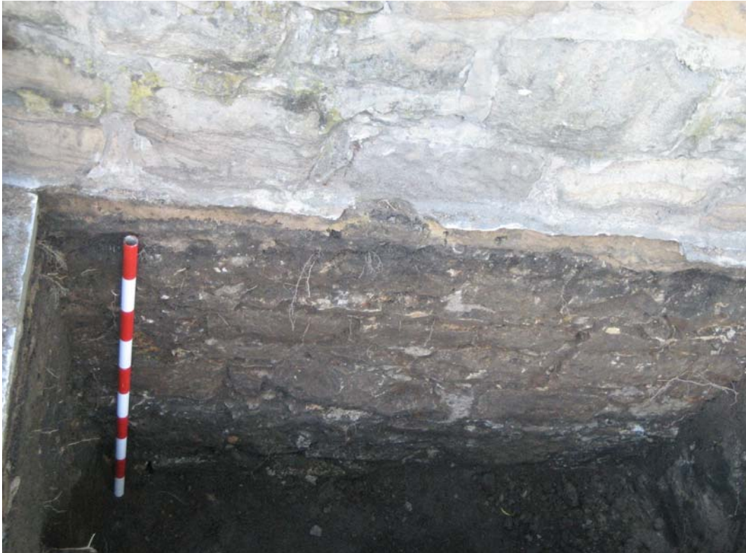
Plate 15: Trench 7, Wall Foundation [729] ( scale 1m )
