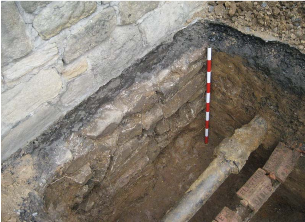
Plate 7: Trench 4, Wall Foundation [411] (scale 1m)
