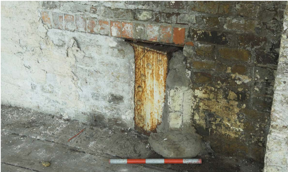
Plate 12: West Handyside Canopy girder visible in the interior of the of the MGS at first floor level in Bay 7 of the west wall
