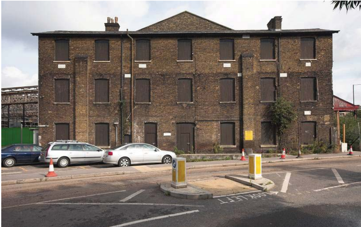
Plate 27: Front (south) elevation of the MGS Offices with the apex of the south gable of the MGS behind
