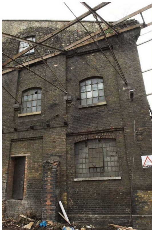
Plate 16: West end of the north elevation of the MGS
