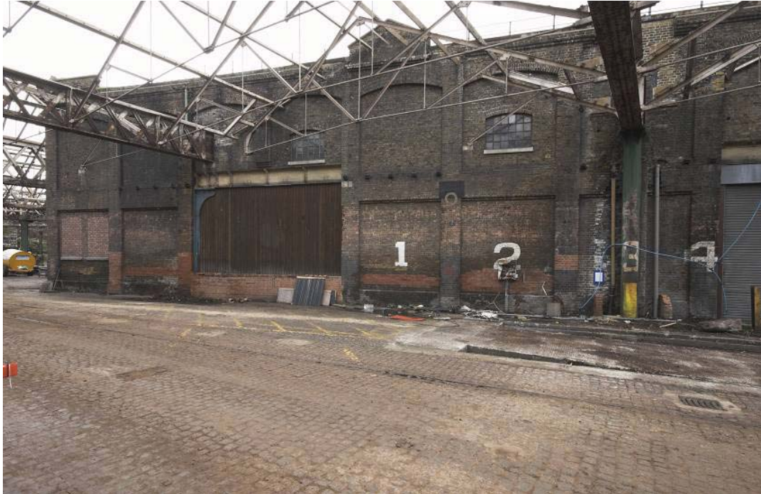
Plate 1: North end (Bays 1 to 7) of the west elevation of the MGS
