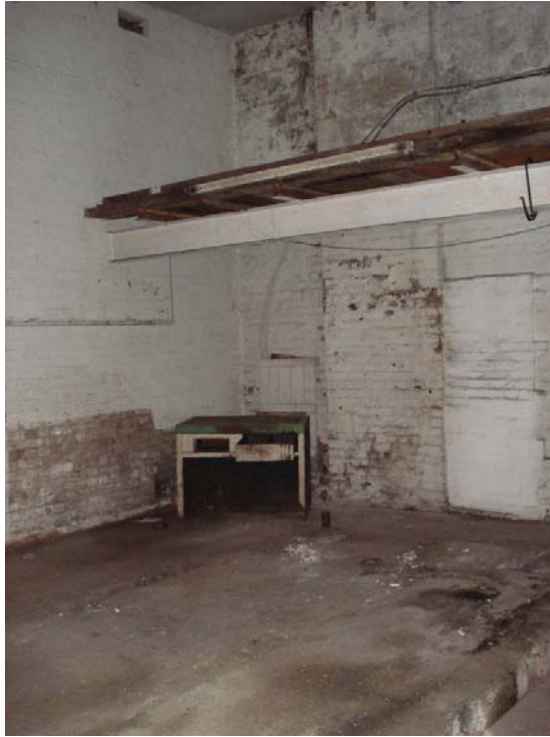
Plate 43c: North-west corner of Pump House MGSG2 in the MGS
