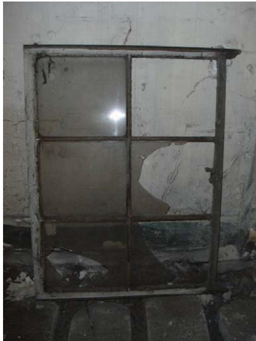
Plate 48: Ex situ upper sash window found in ground floor MGS Office Room MGSOG7 (see Plate 54)
