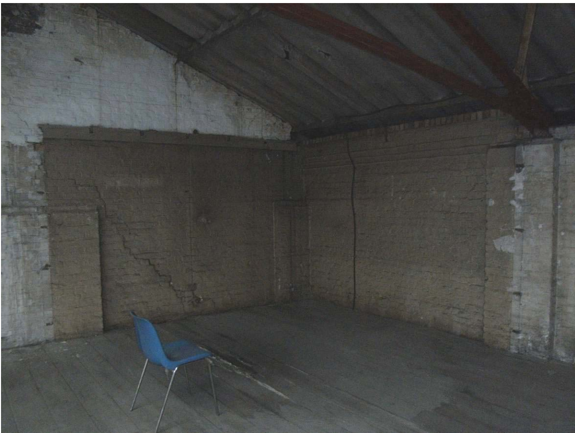
Plate 34: North-east corner of the first floor of the MGS
