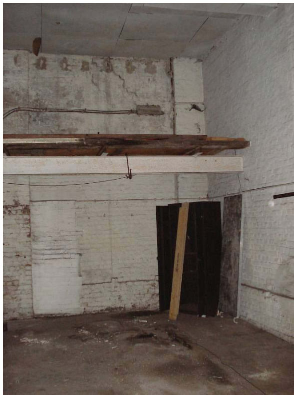
Plate 43b: North-east corner of Pump House MGSG2 in the MGS
