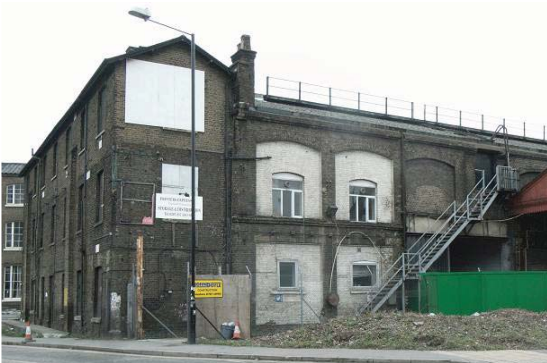
Plate 20: MGS Offices (left) and east elevation of MGS (Bays 21 to 24)
