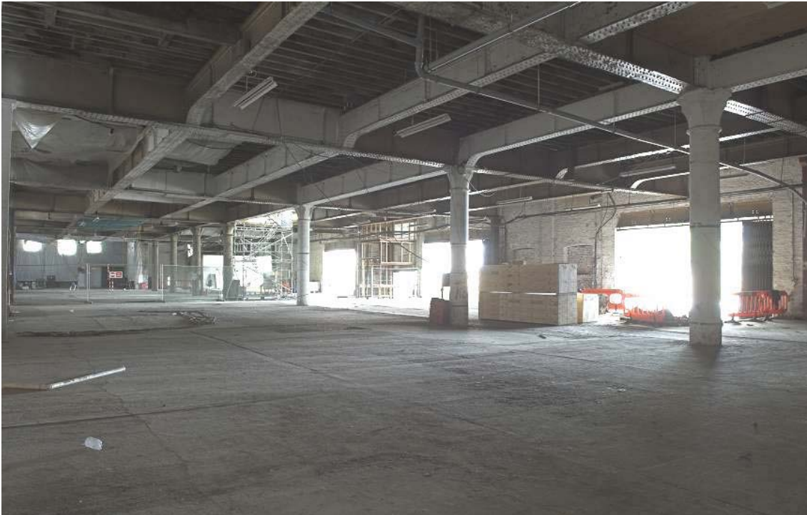
Plate 36: Ground floor of the MGS, view from the south-west
