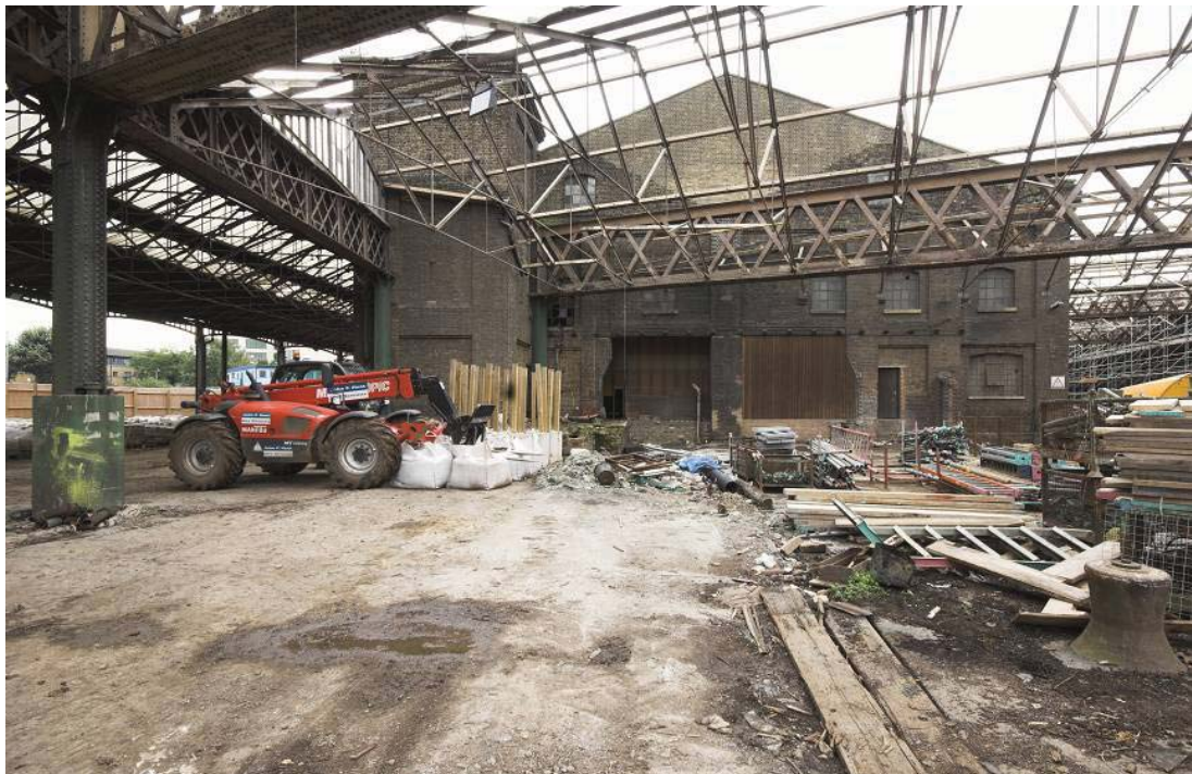
Plate 14: North elevation of the accumulator tower (left) and MGS (right) with capstan in the right (west) foreground
