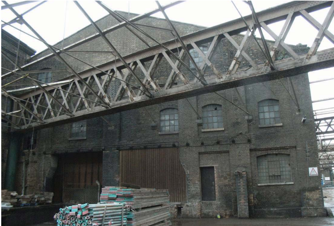
Plate 15: North elevation of the MGS
