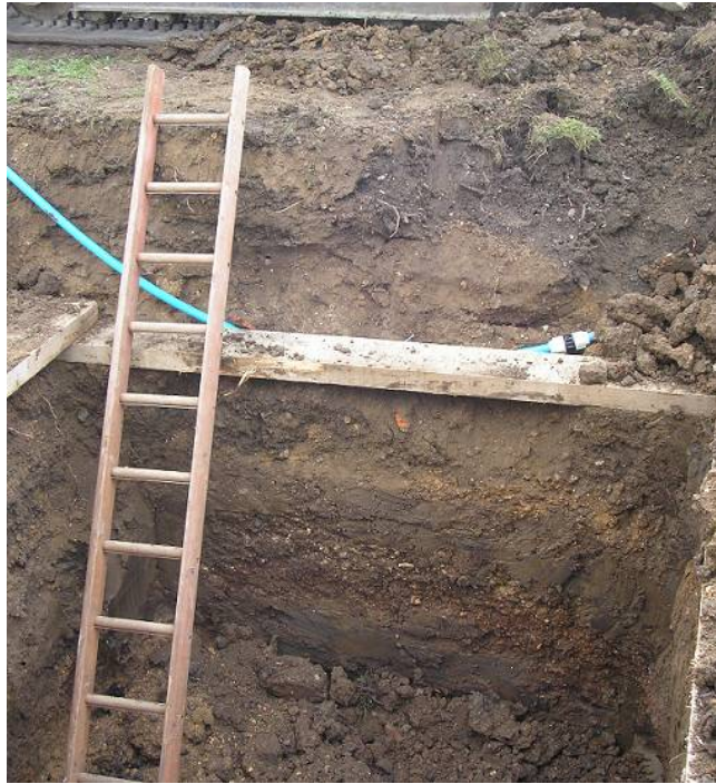
Plate 1: Pipeline A north of Forest Road, looking west, section 28
