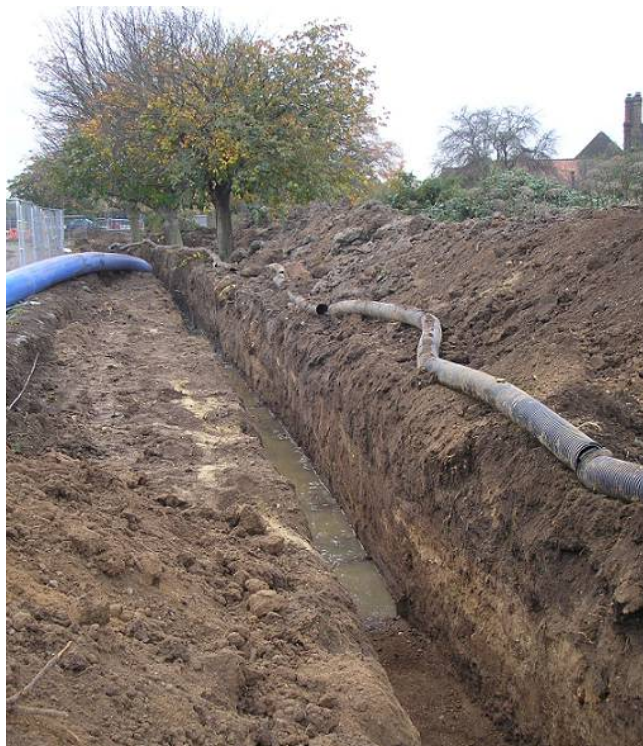
Plate 2: Pipeline A north of Forest Road, looking south, section 30
