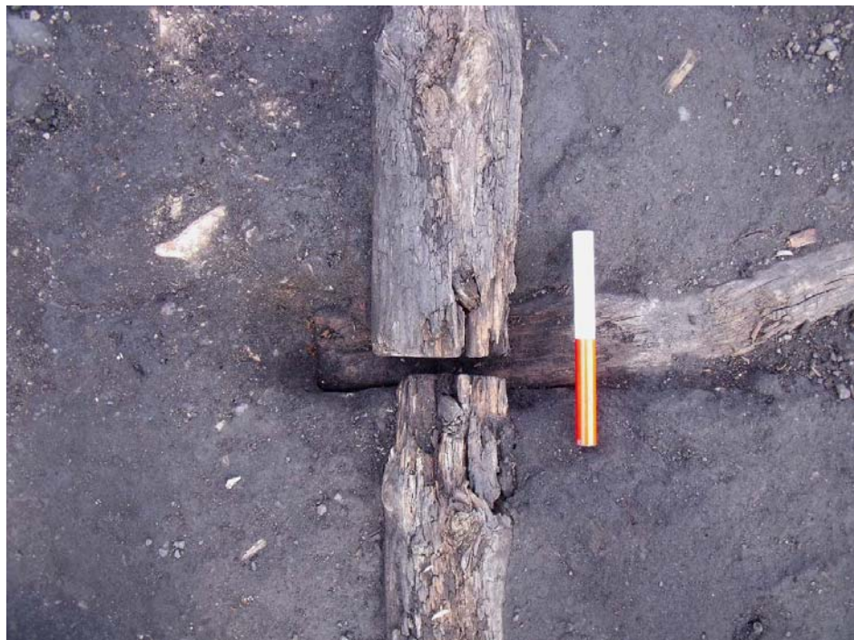
Plate 12. Area A: Rails [216] and [217] on sleeper [191] in waggonway [180] (20cm scale).
