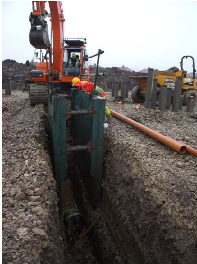
Figure 5. Excavation of Trench 1, looking south
