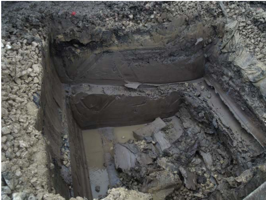
Figure 6. Trench 1, southern inspection chamber excavation, looking south
