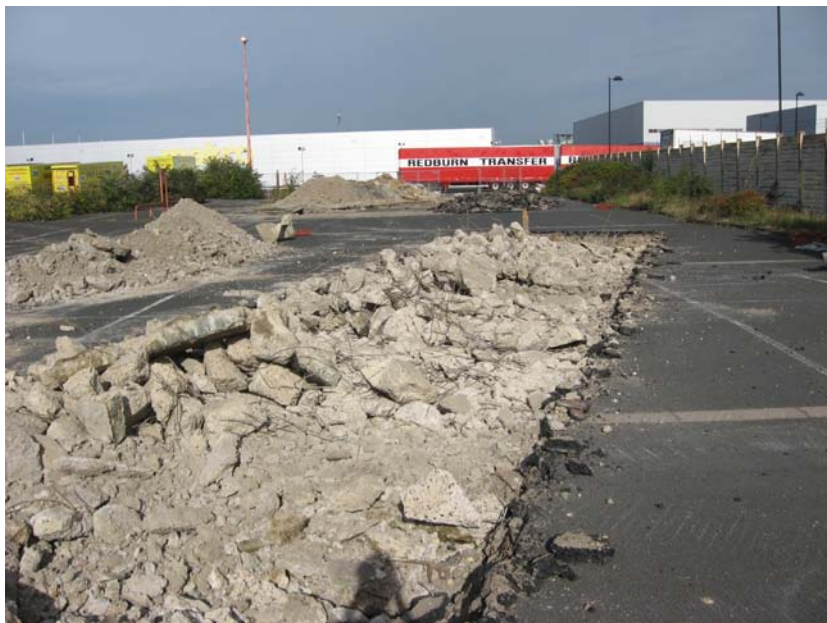
Plate 2: Concrete breaking in progress in Trench 3
