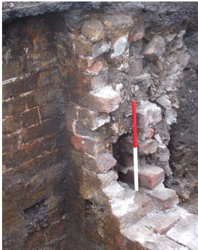
Plate 8. Trench 2: Wall [220], detail, looking south ( 0.5m scale )
