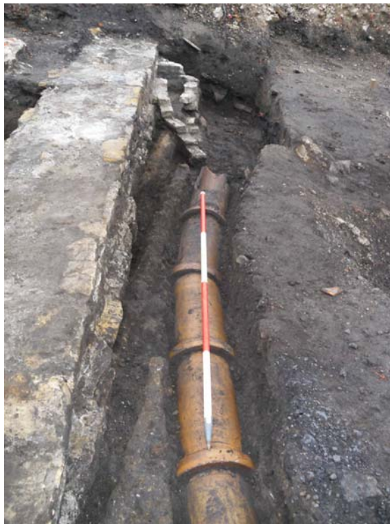
Plate 14: Phase 5c, brick drain [1077] and ceramic drain [1002], looking north-east ( scale 2m )
