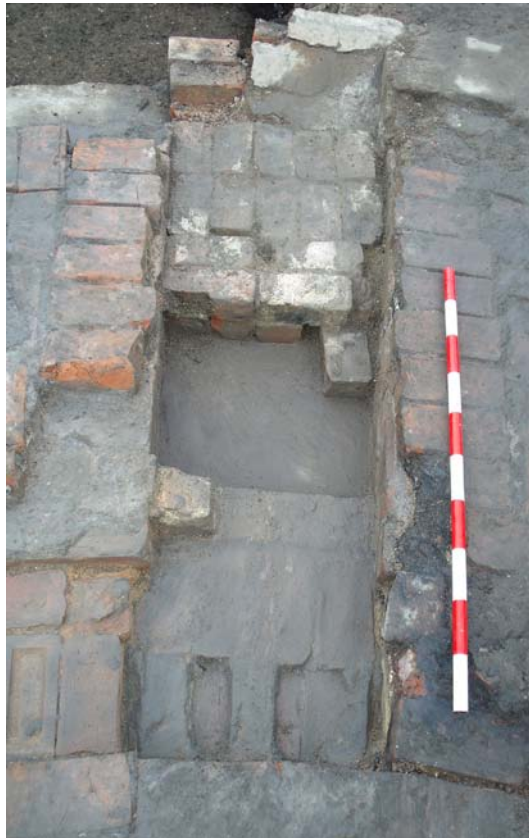
Plate 6: Detail of brick infill [219], within kiln [205], in Trench 2, looking north-east ( scale 1m )
