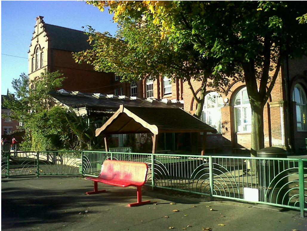
Figure 13 Plate 1 - Westgate Hill Primary School, main building, looking north-west
