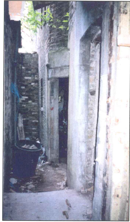
View of the extension looking east
