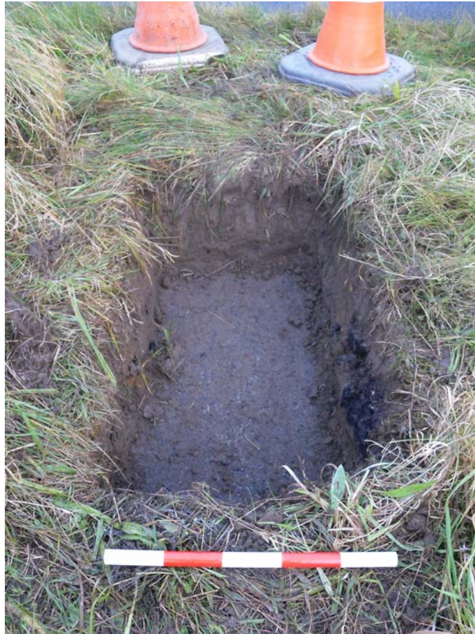
Figure 5. Foundation Pit 25, tarmac surface [4], looking north-east (scale 0.5m)
