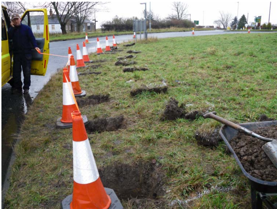
Figure 4. Overview of FPs18-10, looking south.
