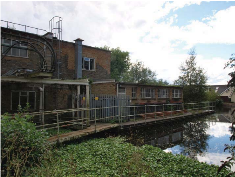
Western extension of the Mill (see Figure 2 for location), view to south-west.
