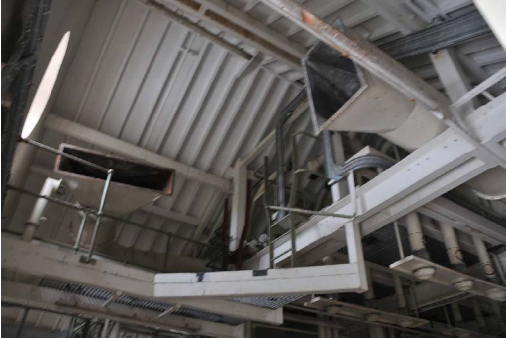
Detail of rafters from third floor of Mill (see Figure 15 for location). View to north-east.
