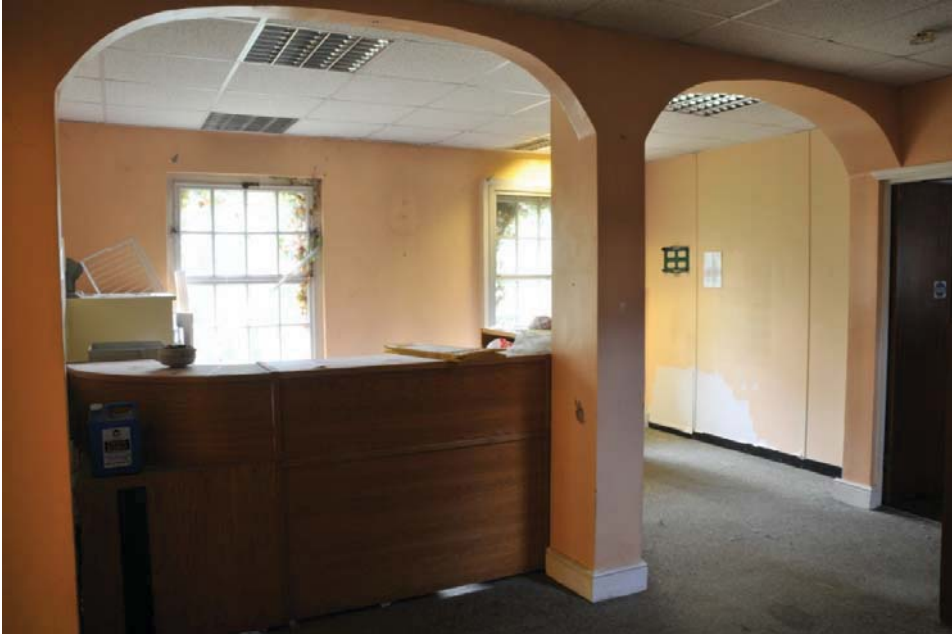
Ground floor reception area, Administration Block. View to south-west.
