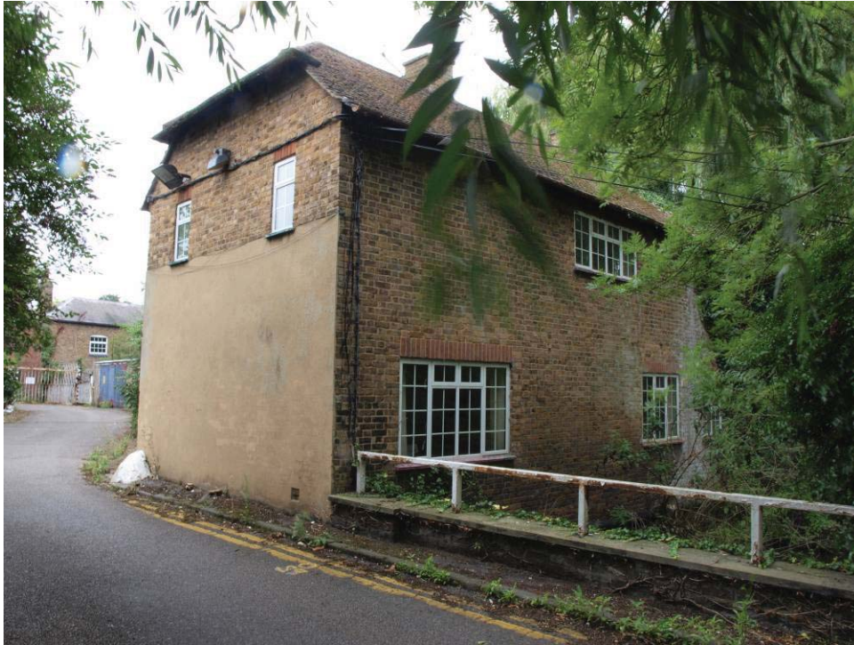
Side (south) and rear (east) elevation of Midway Cottage (see Figure 2 for location), view to north-west
