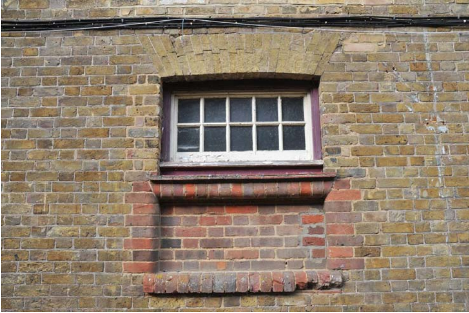
Detail of reduced ground floor window in Bay 6 south elevation of Mill (see Figure 2 for location). View to north.
