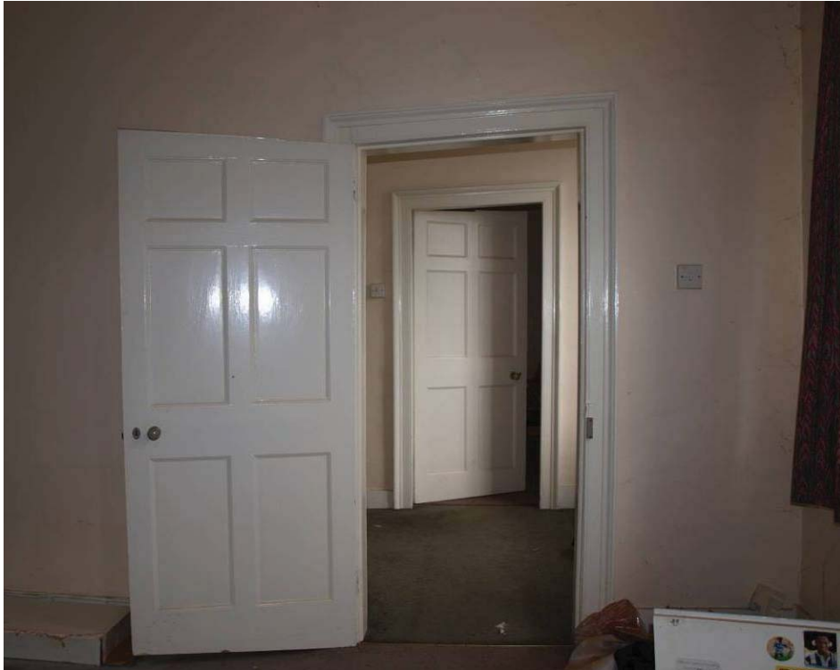
First floor, Kingsmill Cottage, illustrating original door fixtures and warping (see Figure 24 for location). View to south.
