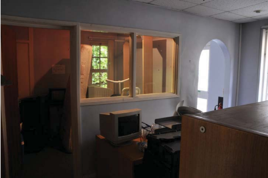
Ground floor Administration Block illustrating earlier part of building. View to north-west.
