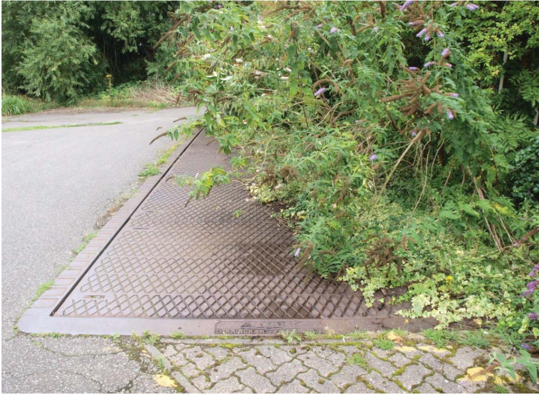
Southern most 'Avery' weighbridge. View to south-west.
