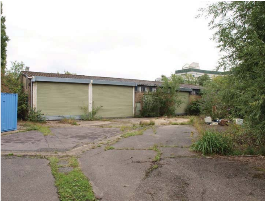
West Elevation of Vehicle Workshop (see Figure 2 for location). View to south-south-east.
