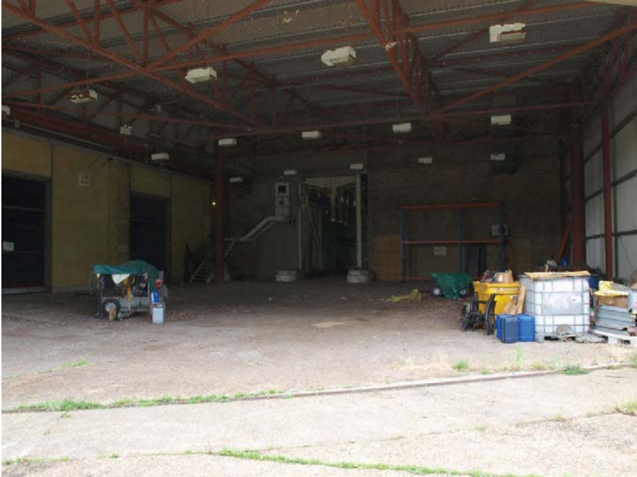
Flour chutes to rear (west) and vehicle loading bay in the northern extension of the Mill (see Figure 2 for location), view to south-west.
