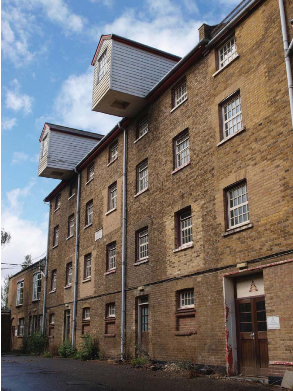
South elevation of Mill (see Figure 2 for location). View to north-west.
