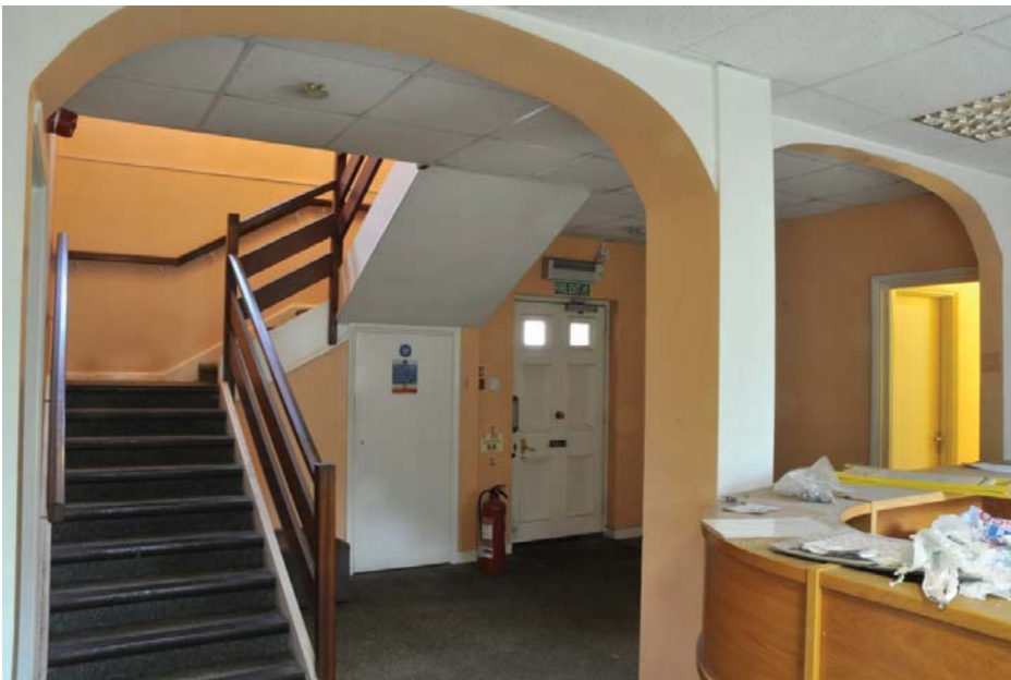
View to north-east of staircase from reception area, ground floor, Administration Block.
