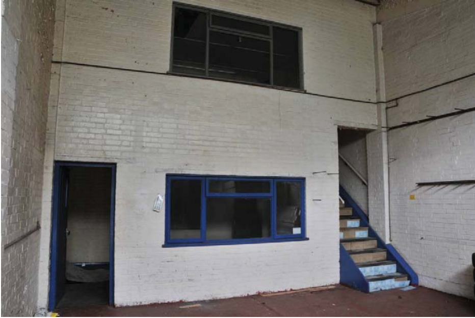
Offices of Vehicle Workshop (see Figure 2 for location). View to east-south-east.
