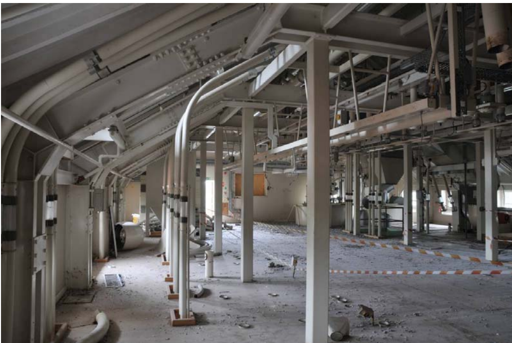
Third floor of Mill (see Figure 15 for location). View to west-north-west.
