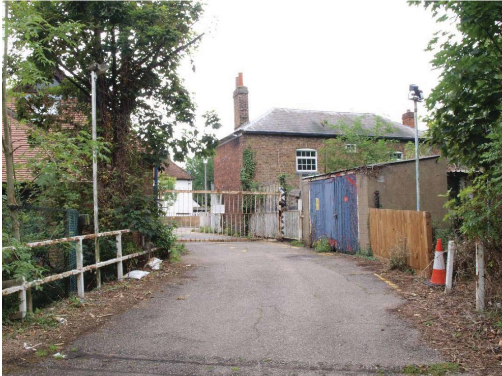
Rear elevation depicting both chimney stacks of Kingsmill Cottage (see Figure 2 for location). View to west.
