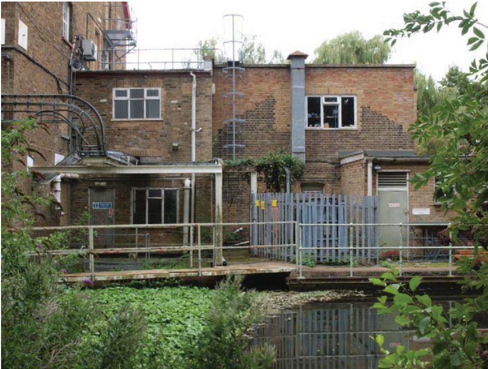
Western extension of the Mill, showing scar of former gable (see Figure 2 for location), view to south
