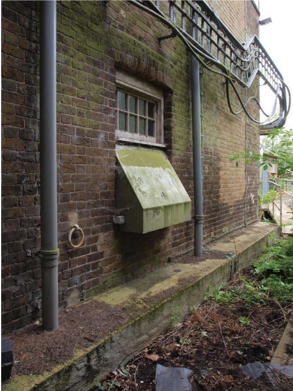
Detail of mooring rings along Mill's north elevation and in-filled dock (see Figure 2 for location). View to south-west.
