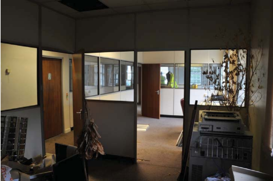
Office partitions of first floor, Administration Block. View to east-north-east.
