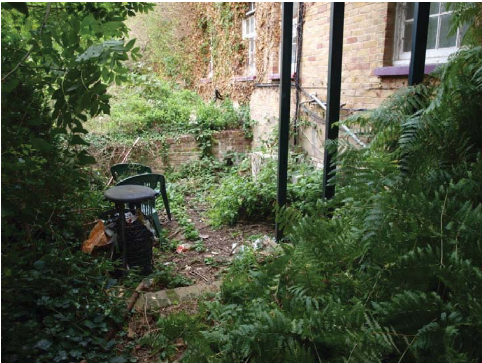
South Elevation of Administration Block to east illustrating former in-filled channel (see Figure 2 for location). View to west-north-west.
