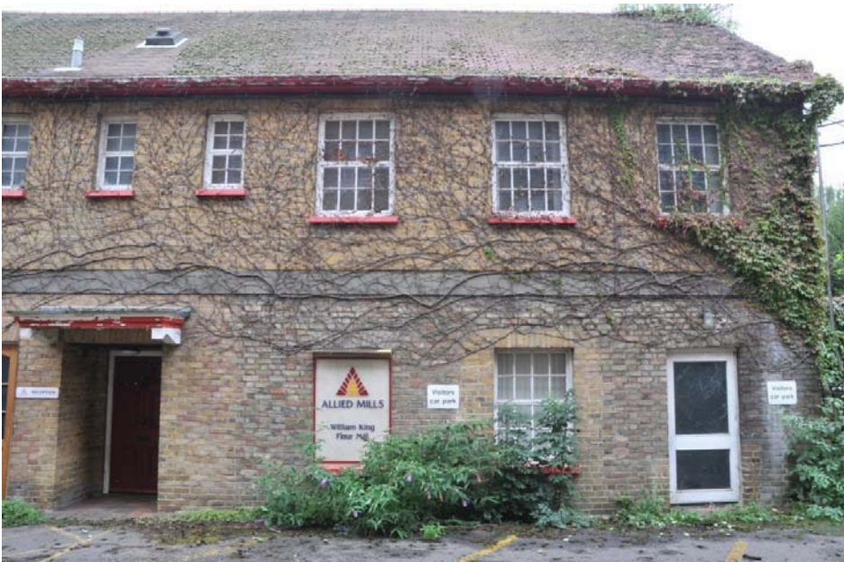
North Elevation of Administration Block to west (see Figure 2 for location), illustrating original building. View to south.
