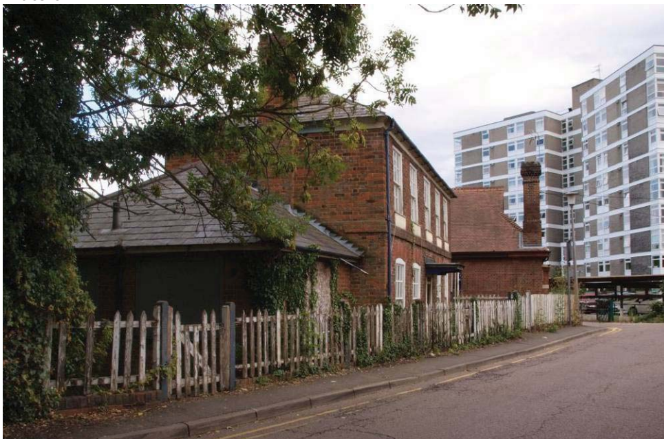
North elevation and extension, Kingsmill Cottage (see Figure 2 for location). View to south-east.
