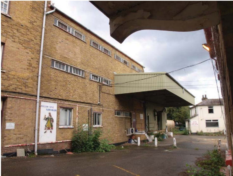
South elevation of Mill's early 1960's eastern extension (see Figure 2 for location), view to north-east
