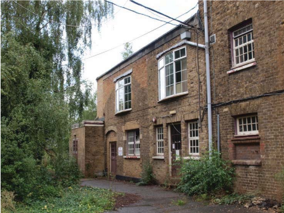
South elevation of the western extension of the Mill (see Figure 2 for location), view to north-west
