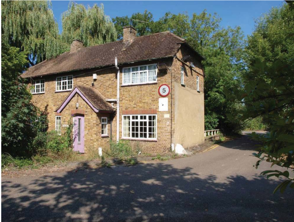
West (front) elevation of Midway Cottage (see Figure 2 for location), view to north-east
