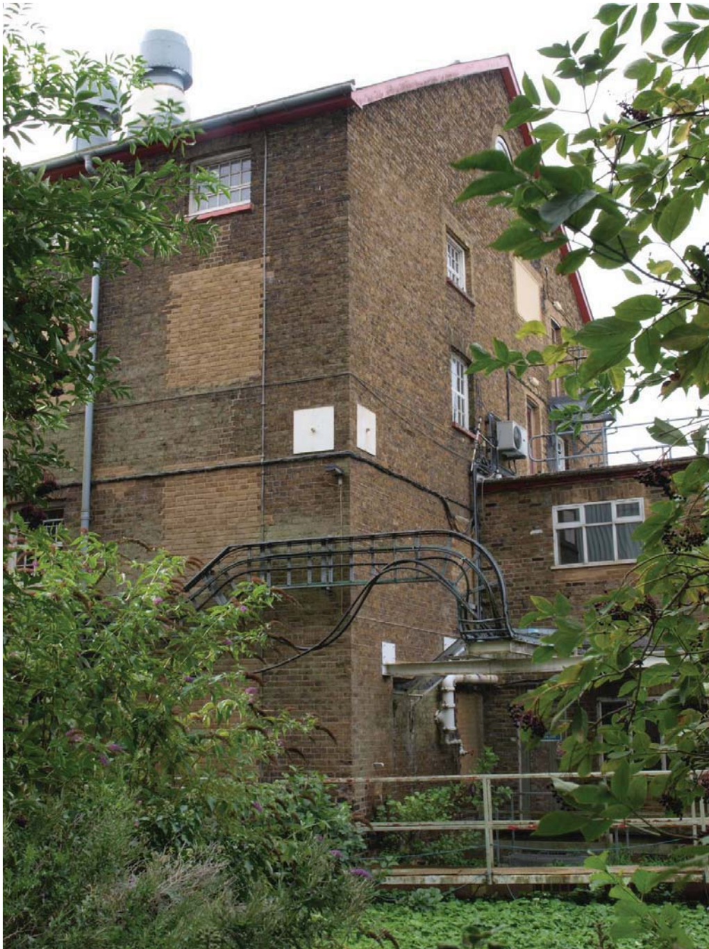
North (left) and west (right) elevation of Mill (see Figure 2 for location). View to south-east.
