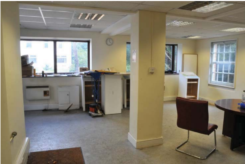
Ground Floor Administration Block to east. View to south-east.
