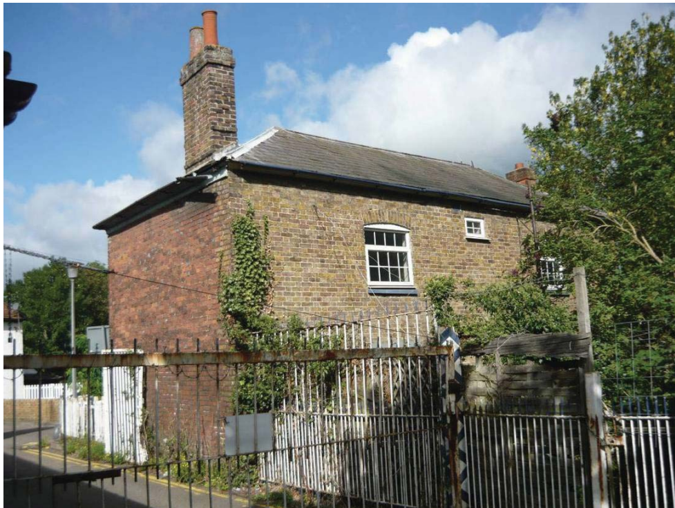
West Elevation, Kingsmill Cottage (see Figure 2 for location). View to north-west.
