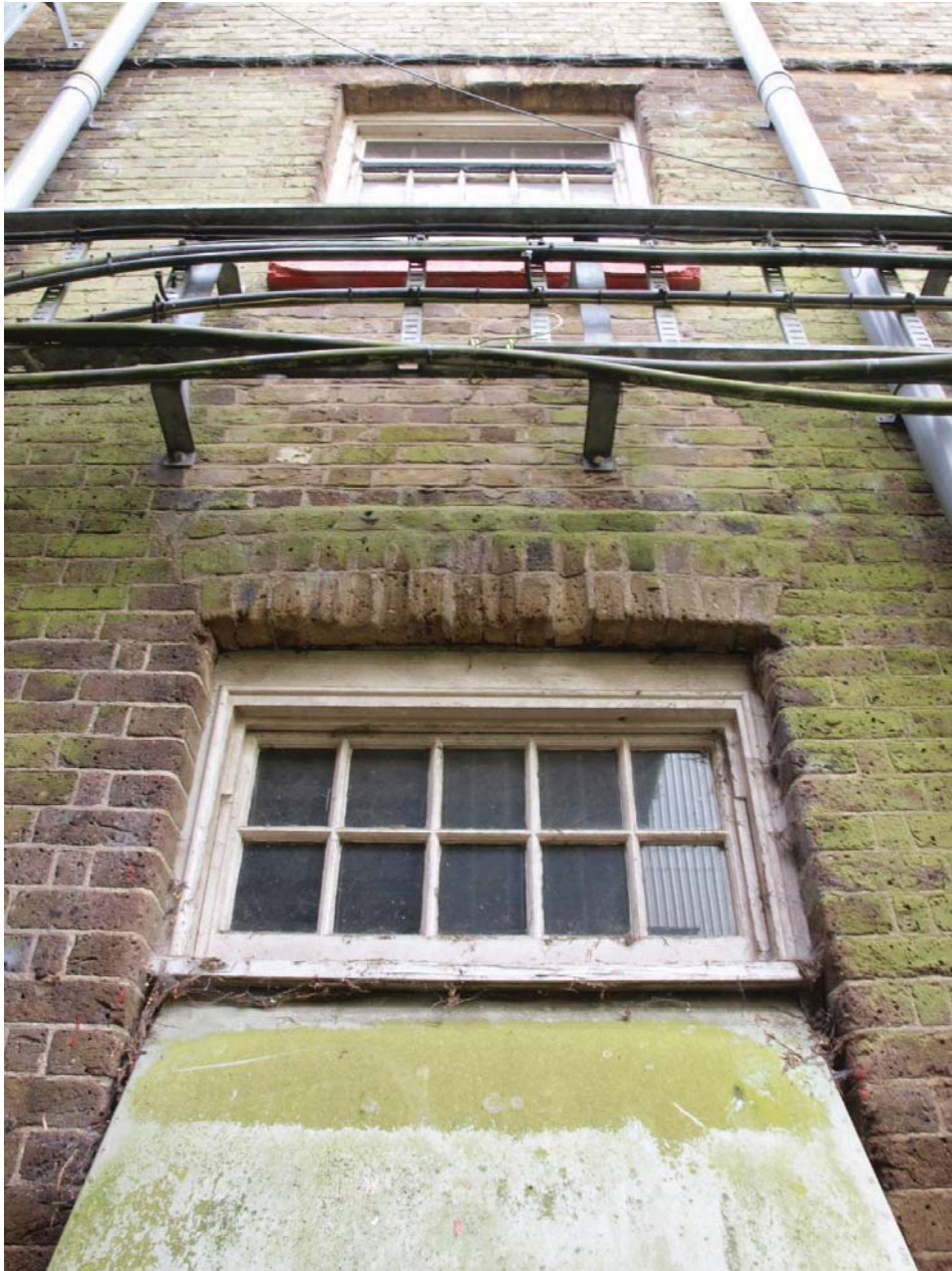
Detail of wear patterns on ground floor window arch in Bay2, north elevation of Mill (see Figure 2 for location). View to south.
