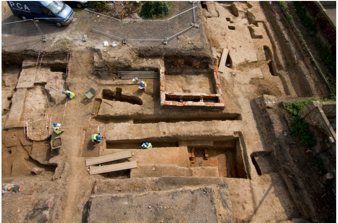
Plate 1: Site view looking south
