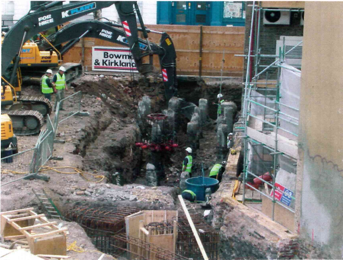
Plate 1: View of the northeast corner of the site.
