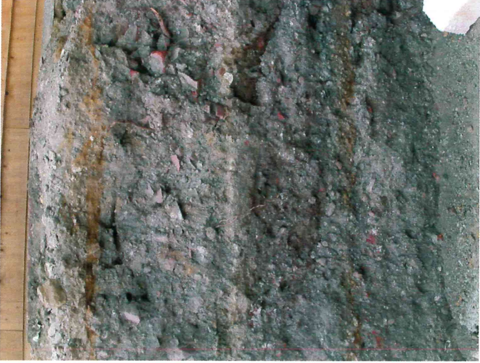
Plate 5: South facing section at the northeast corner of the site (2m depth).
