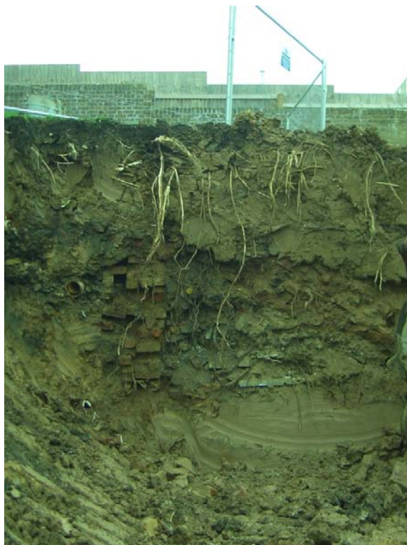
Plate 1: View NE of modern wall and associated truncation, with truncated natural clay visible.
