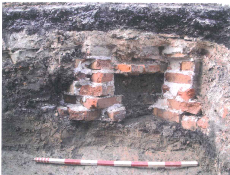
Above: Wall [11] and tile floor [23] in section. Below left: Wall [2] in the foreground (truncated to the west by a machine sondage) and stepped foundation [22] sealed by rebuild [1] in the background. Below right: Detail of stepped foundation [22] sealed by later rebuild [1]. Note the poor quality of the pointing undertaken in the construction of [1], suggesting it may be trench built within a construction cut.
