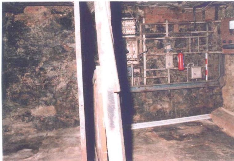
Plate 2 Stone Basement, Room B01
