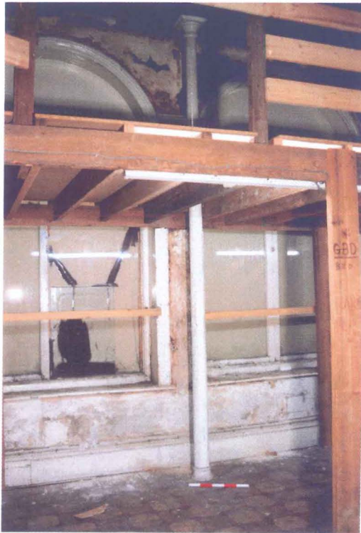
Plate 7 Historic windows, Room 1F02
