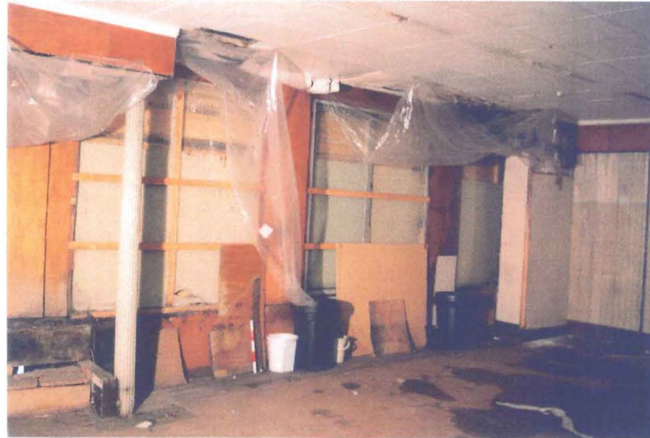
Plate 6 Historic shop front, Room 1F07
