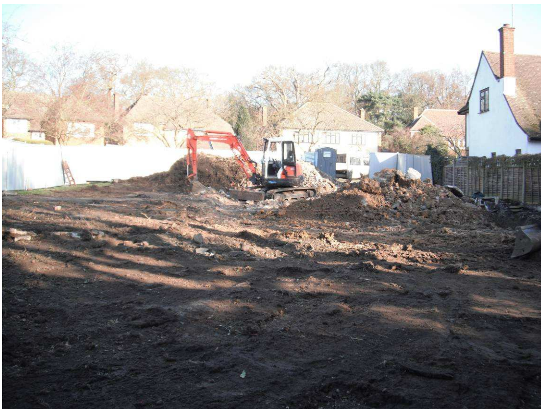
Site view to north
