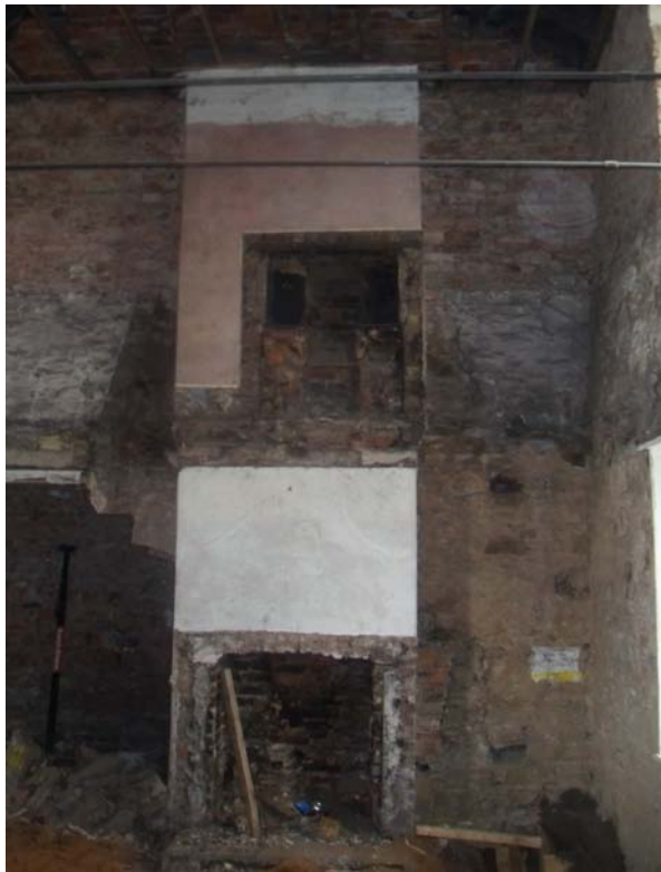
Plate 24. Detail of interior, chimney breast in western gable end of farmhouse. No scale.
