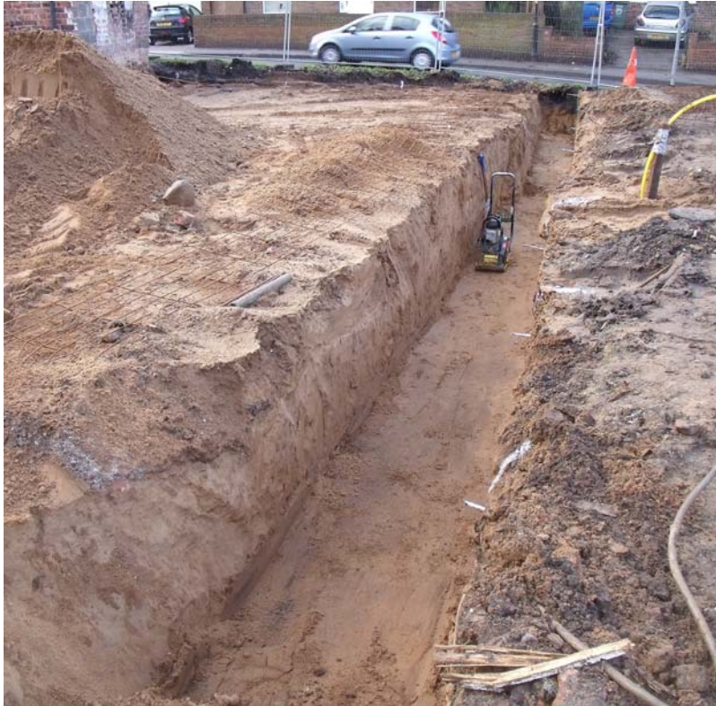
Figure 12 Northernmost element of new build footings, looking WSW
