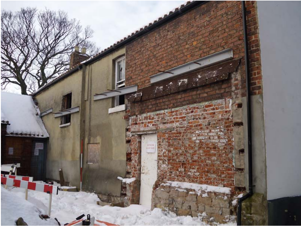
Plate 19. South facing elevation (oblique) of farmhouse. 2m scale.
