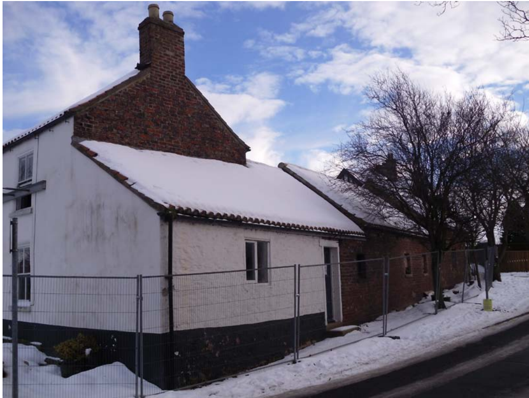
Plate 9. West facing elevation (oblique) of farmhouse and outbuildings. No scale.
