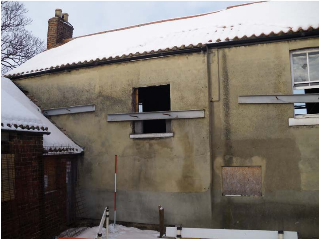
Plate 13. South facing elevation (oblique) of western part of farmhouse. 2m scale.
