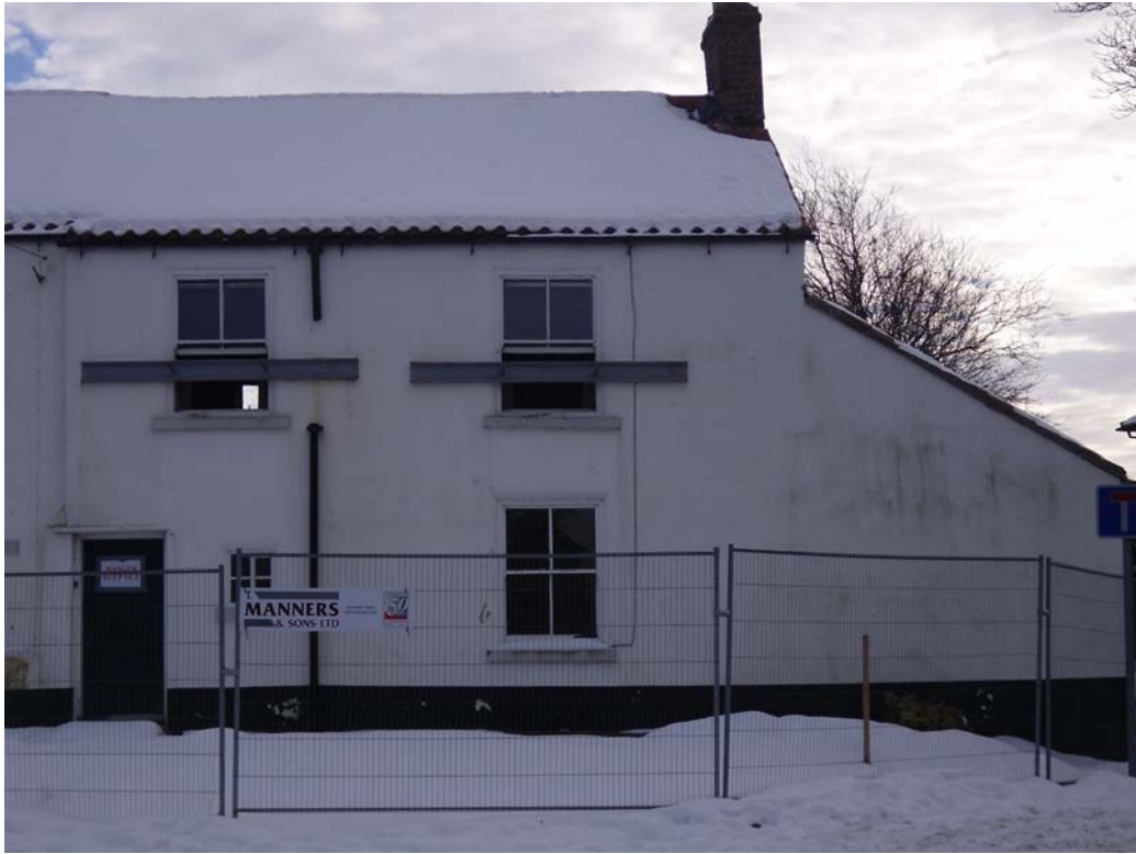
Plate 5. North facing elevation of western part of farmhouse. No scale.
