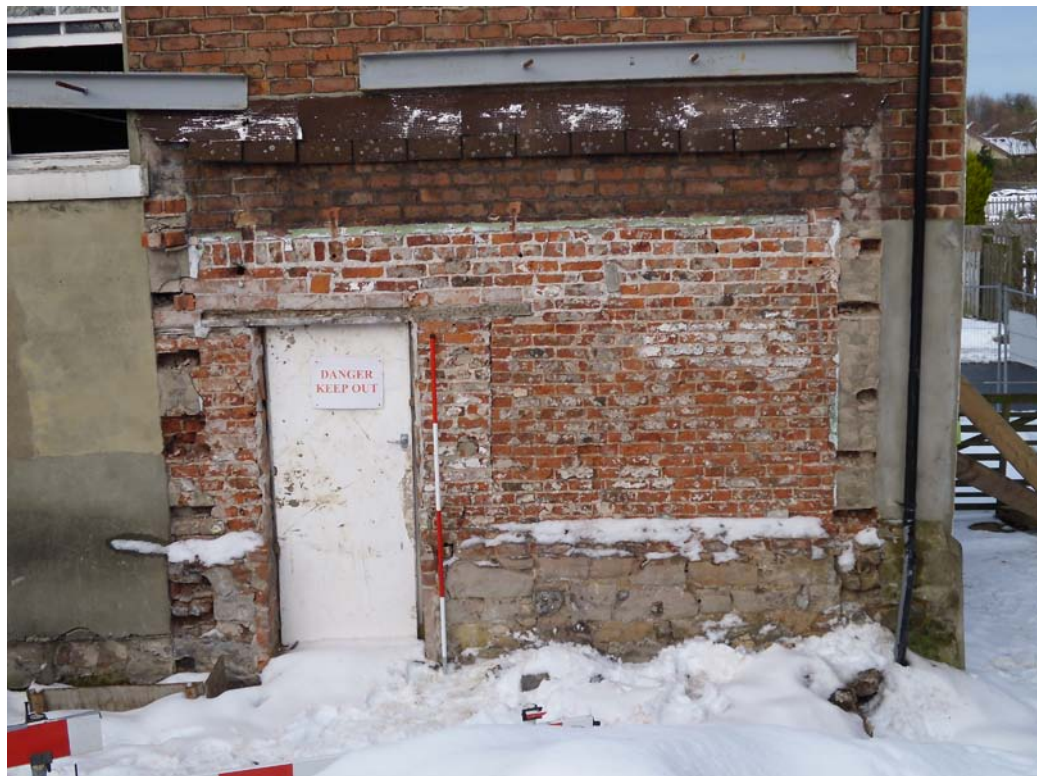
Plate 16. Detail of lower part of south facing elevation of eastern part of farmhouse. 2m scale.
