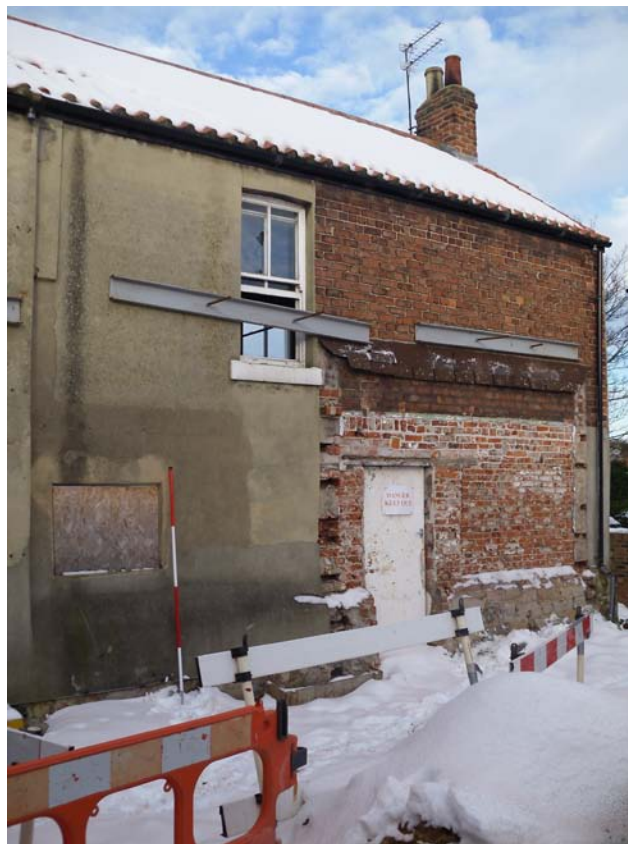
Plate 12. South facing elevation (oblique) of eastern part of farmhouse. 2m scale
