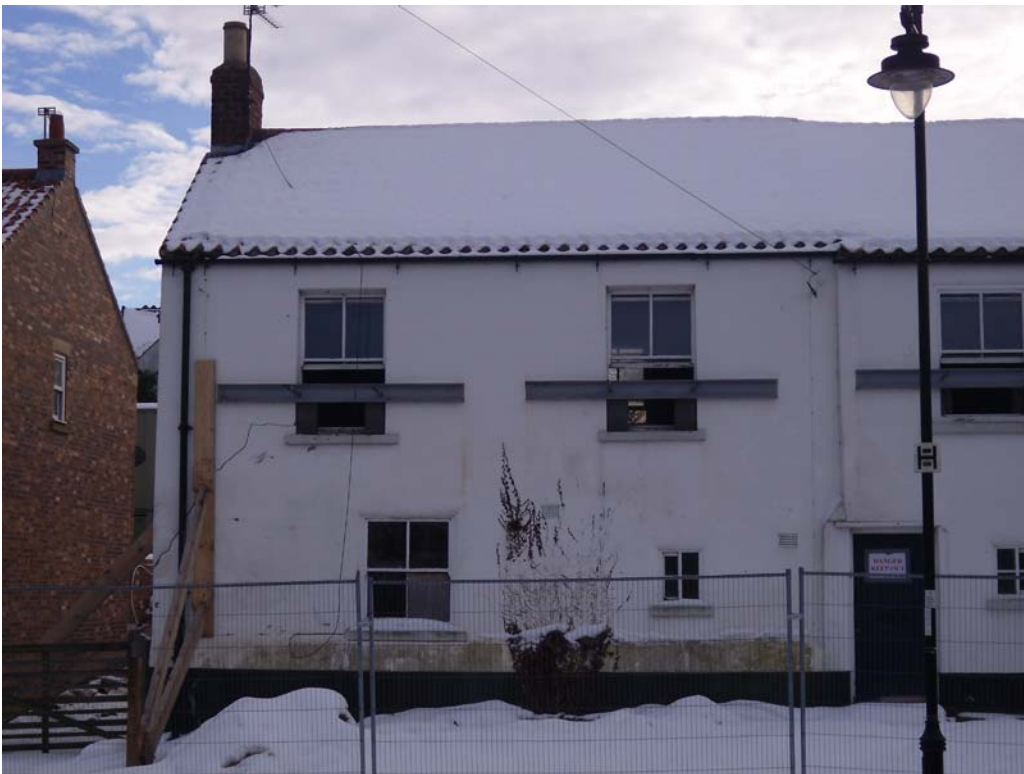
Plate 4. North facing elevation of eastern part of farmhouse. No scale.
