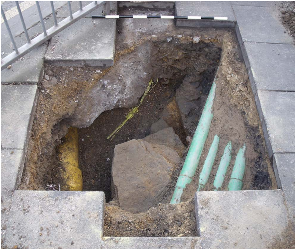
Figure 17: Overview of Trench 2, looking south-west ( scale 1m )
