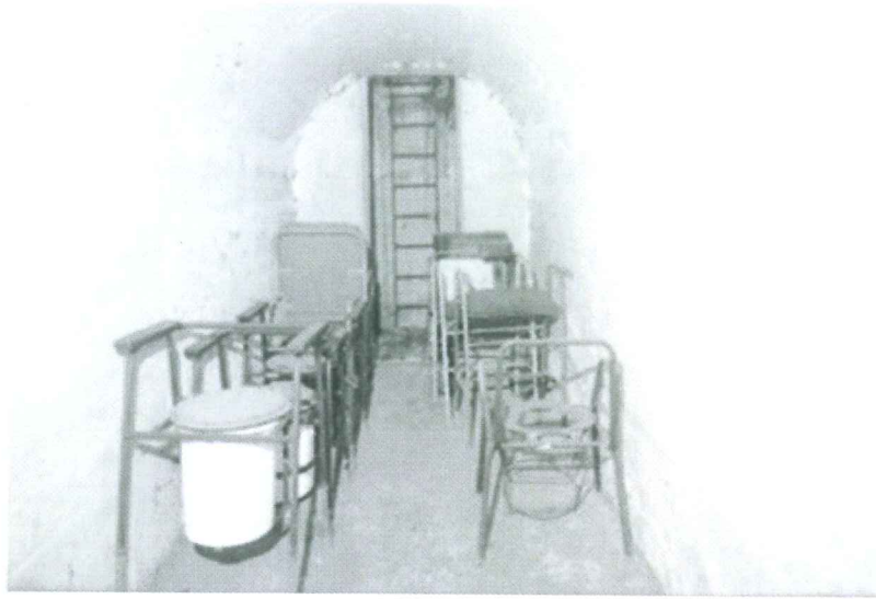
Plate 2 The shelter interior with escape hatch and ladder to the rear
