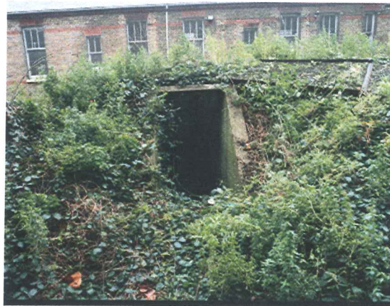
Plate 1 The entrance to the shelter
