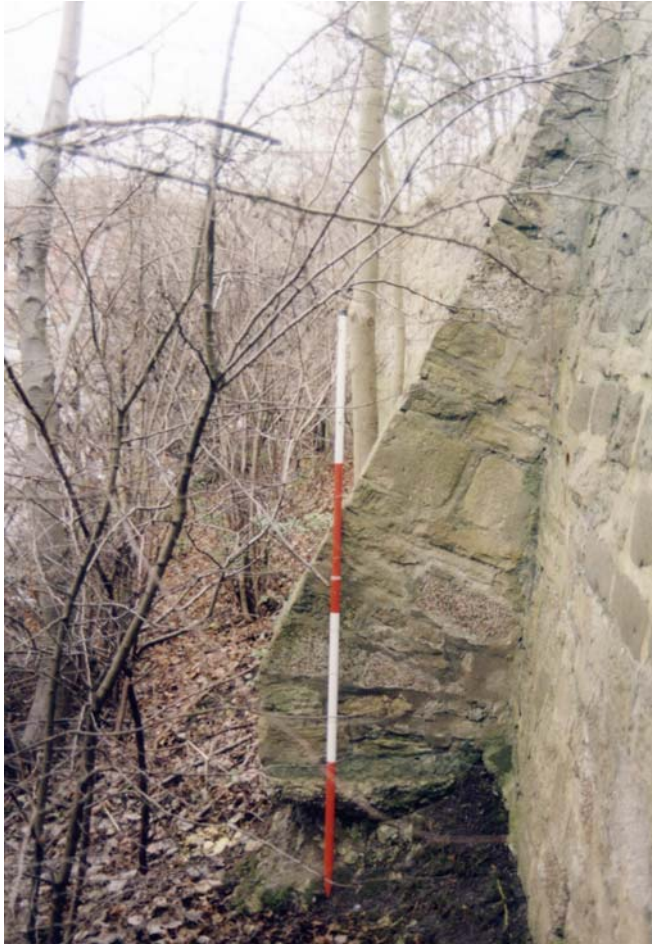
Plate 13. Buttress 3. Section 3 of revetment wall, looking SSW (2m scale).
