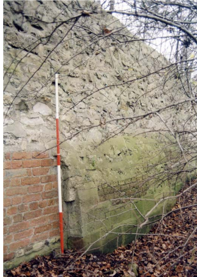
Plate 12. Buttress 2. Section 1 of revetment wall, looking north-west (2m scale).
