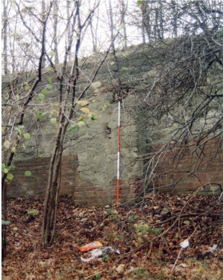
Plate 11. Buttress 1. Section 1 of revetment wall, looking west (2m scale).
