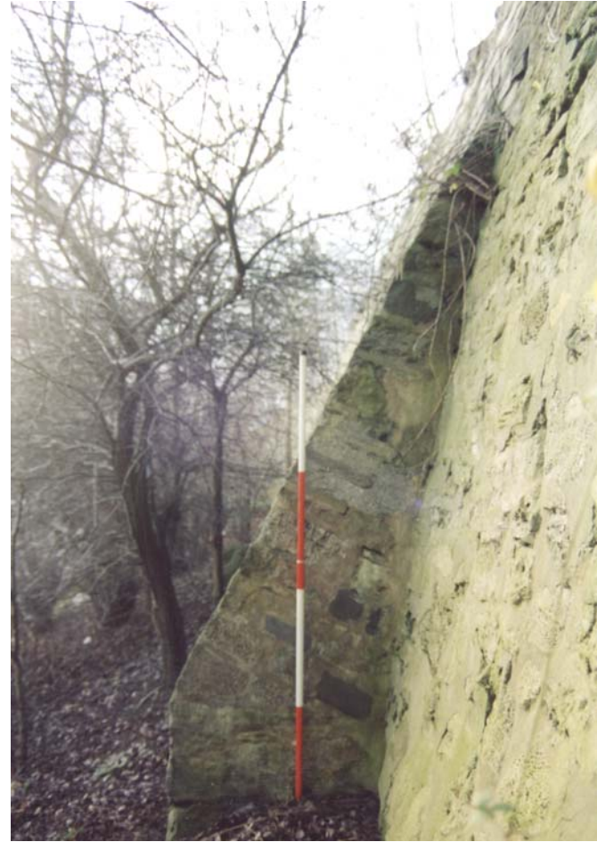
Plate 14. Buttress 4. Section 2 of revetment wall, looking SSW (2m scale).
