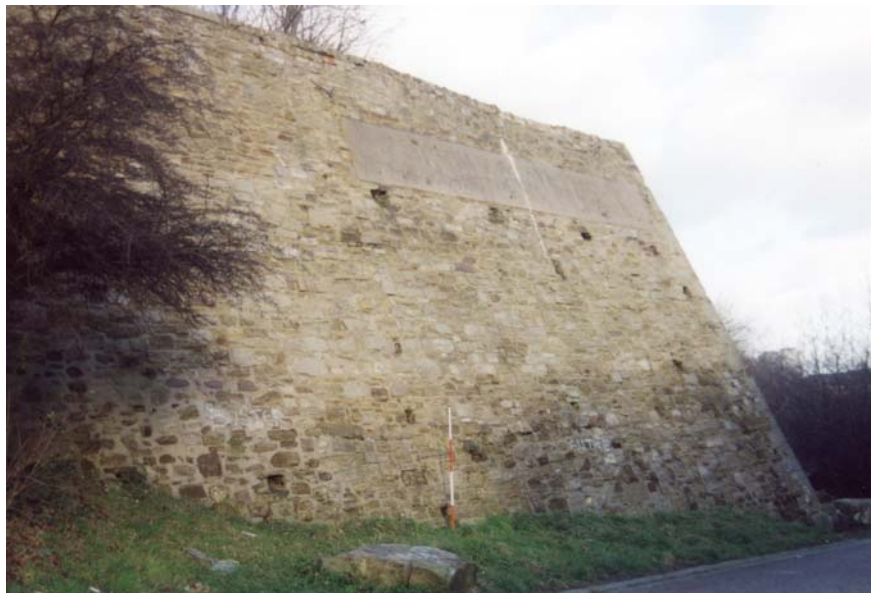
Plate 8. Section 3 of revetment wall, looking north-west (2m scale).
