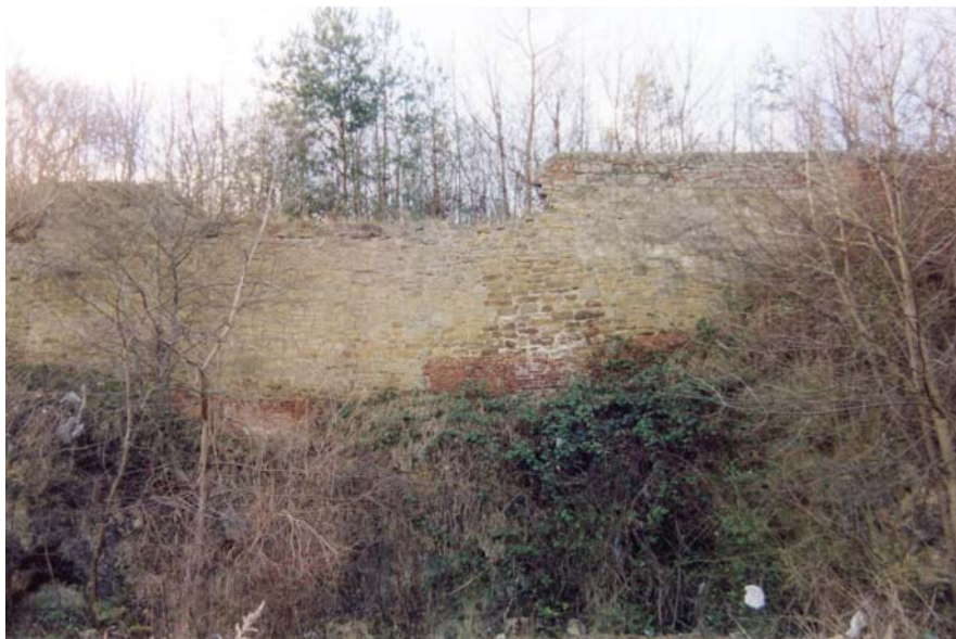
Plate 10. Section 4 of revetment wall, looking south-west ( 2m scale ).
