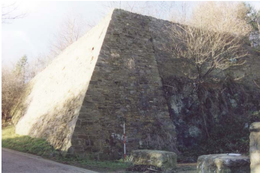
Plate 9. Sections 3 and 4 of revetment wall, looking west ( 2m scale ).
