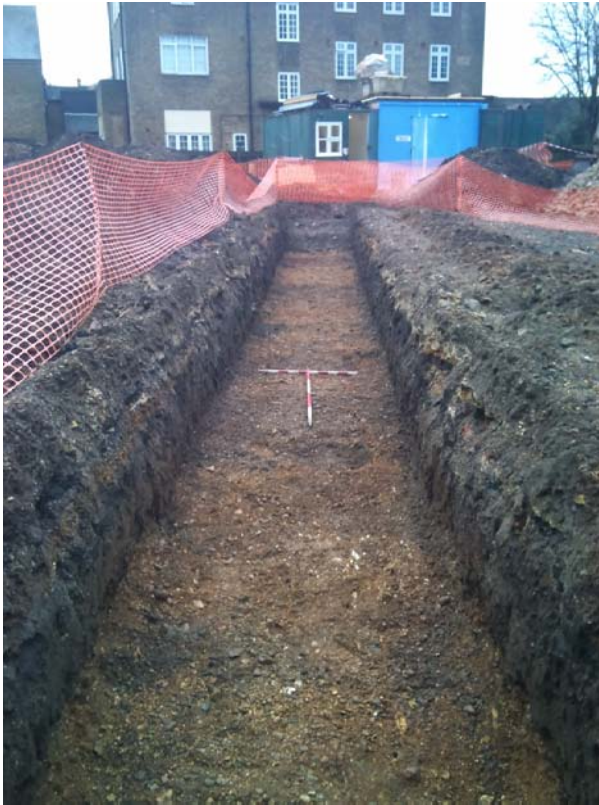
Plate 3: Trench 3, view S, after evaluation machining
