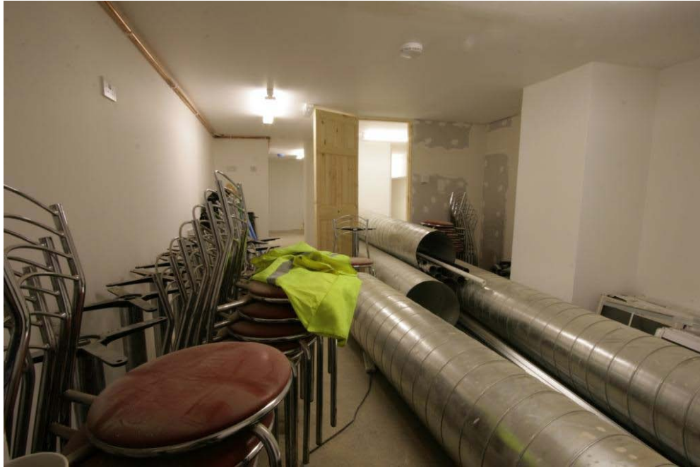
Plate 19. Basement looking west after refurbishment. (PCA)
