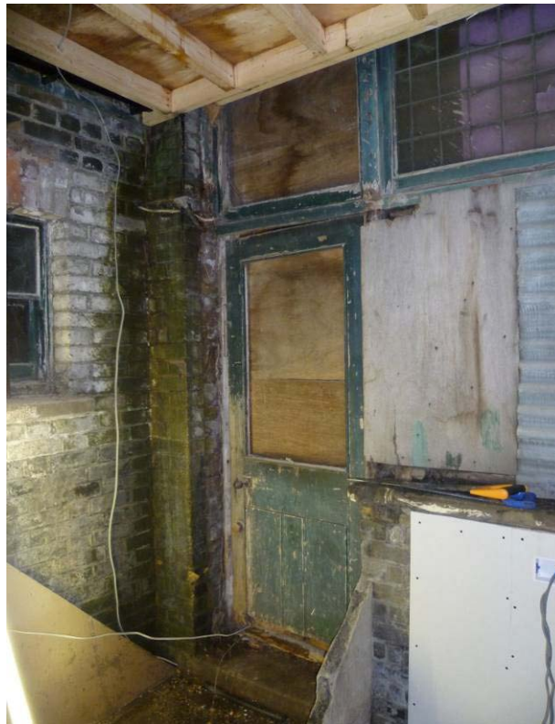
Plate 4. Door and windows on the north side of the yard. (JM)
