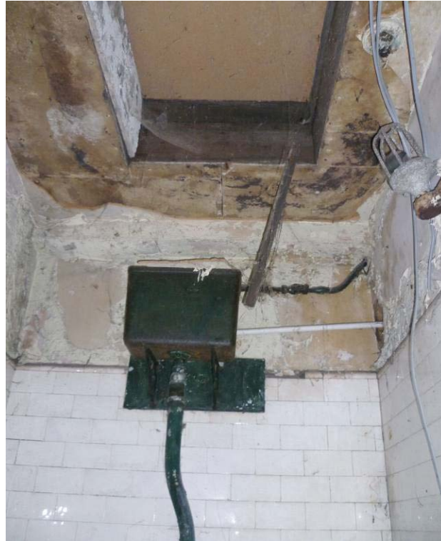
Plate 13. White tiled walls, toilet cistern and skylight of west/yard toilet. (JM)
