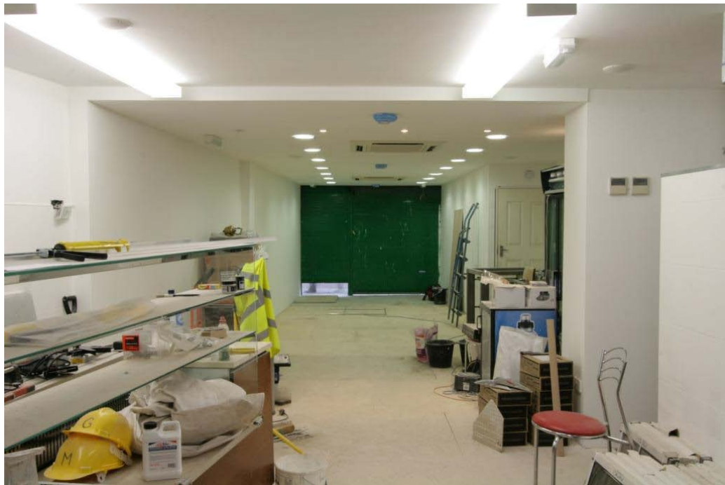
Plate 6. Refurbished ground floor looking east towards the street frontage. (PCA)
