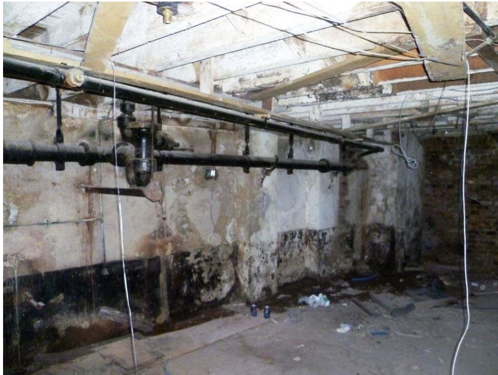
Plate 18. North wall at east end of the basement showing two brick buttresses that would have supported a chimney breast above. (JM)
