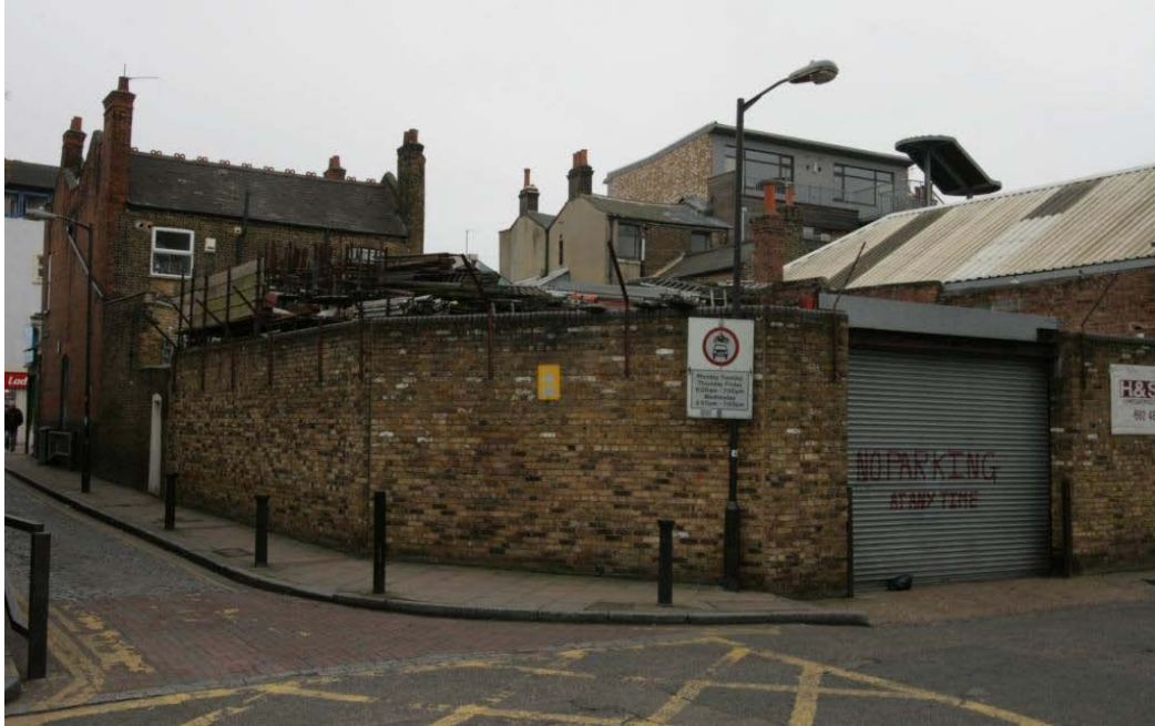
Plate 3. Rear elevation of 45 Deptford High Street looking south-east. The double gable of the north elevation each with a chimney stack at the apex can be seen in the centre of the picture. The construction of buildings on Comet Street in the foreground meant the only access to the property is from Deptford High Street. (PCA)
