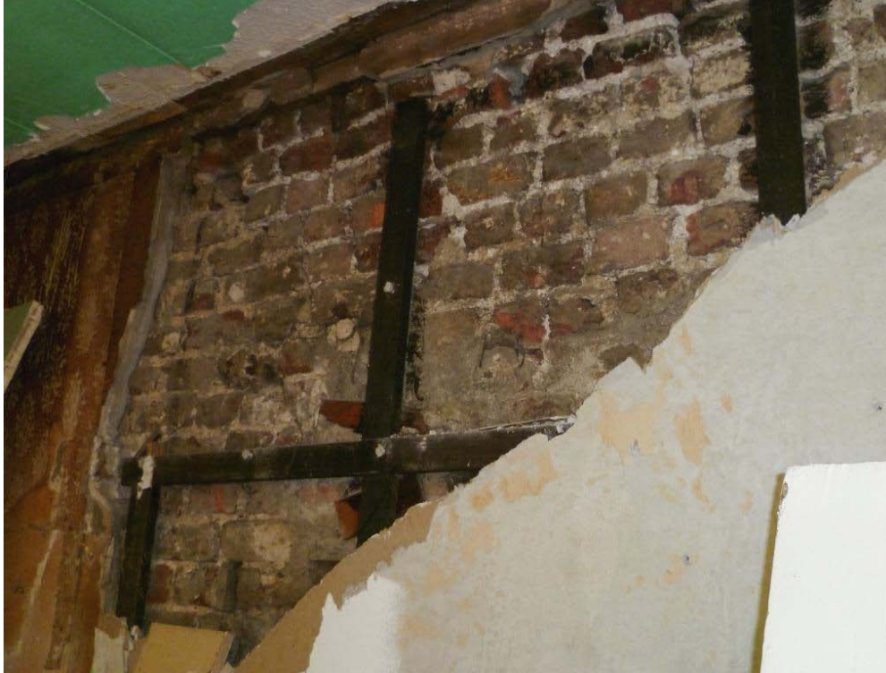
Plate 7. North party wall of 45 Deptford High Street exposed on the ground floor in the shop front area, revealing red brick laid in English bond with a white lime mortar. (JM)
