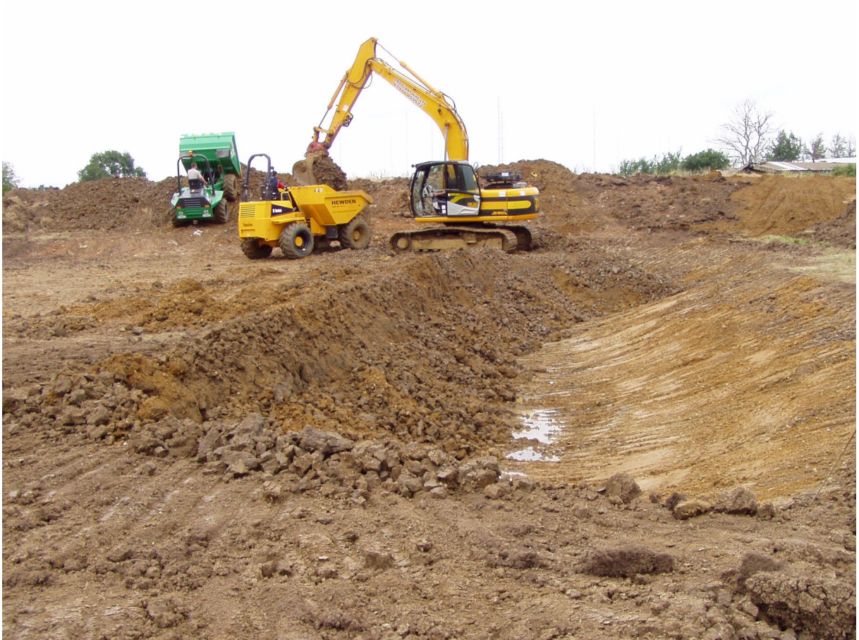
Plate 3: Excavation of Pond 1, viewed from the South.
