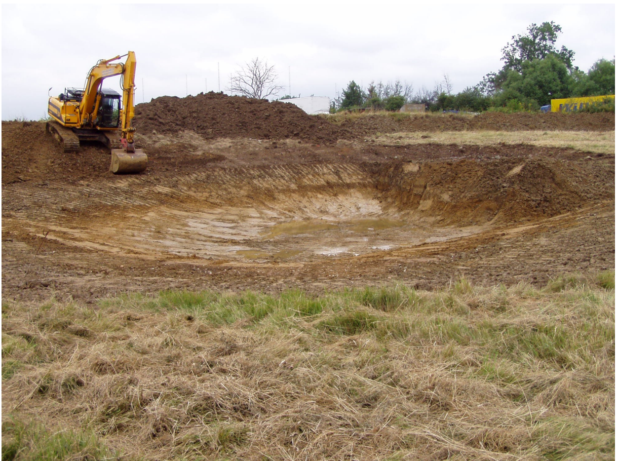
Plate 2: Excavation of Pond 2, viewed from the South-West.
