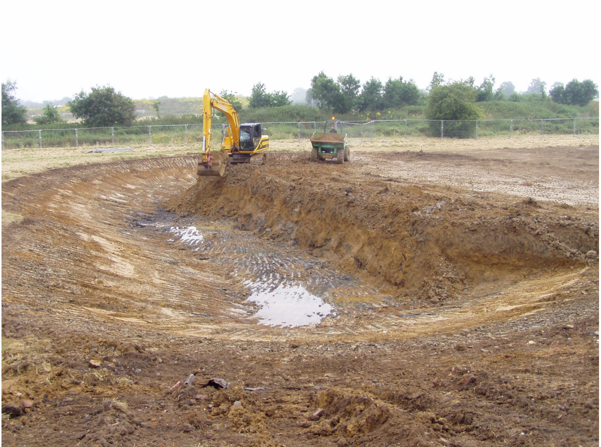
Plate 4: Excavation of Pond 1, viewed from the North-West.
