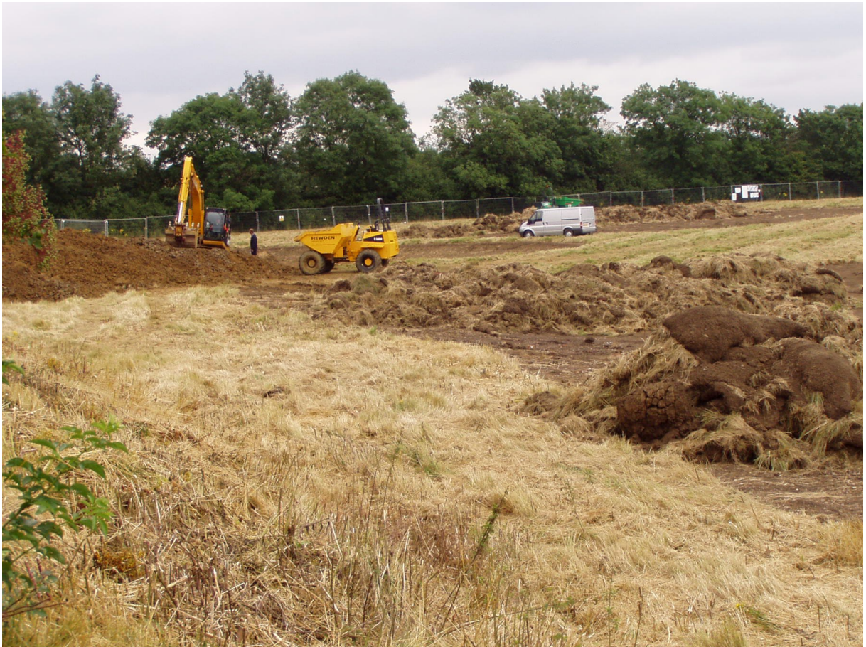
Plate 1: Topsoil Strip of Pond 2, viewed from the North-West.
