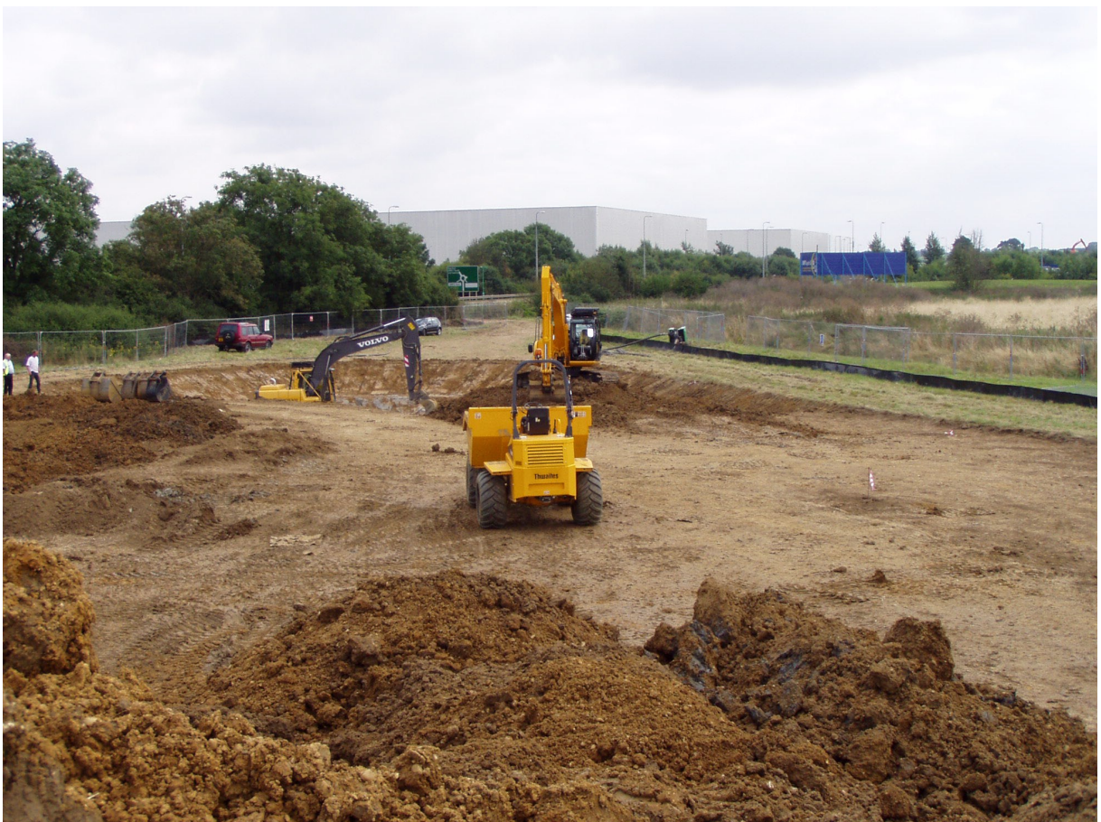
Plate 6: Excavation of Pond 4, viewed from the North-West.
