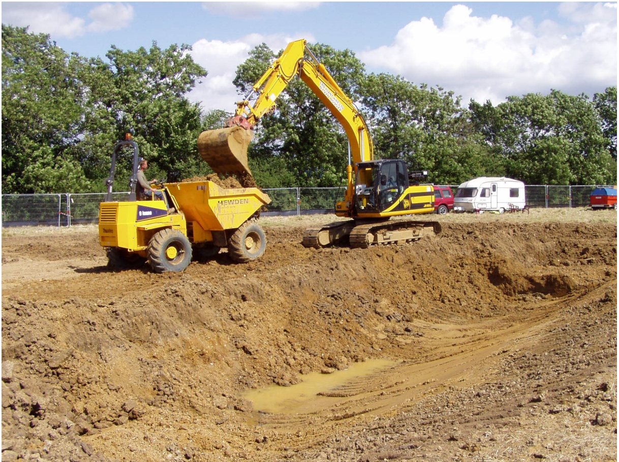
Plate 5: Excavation of Pond 3, viewed from the North-West.
