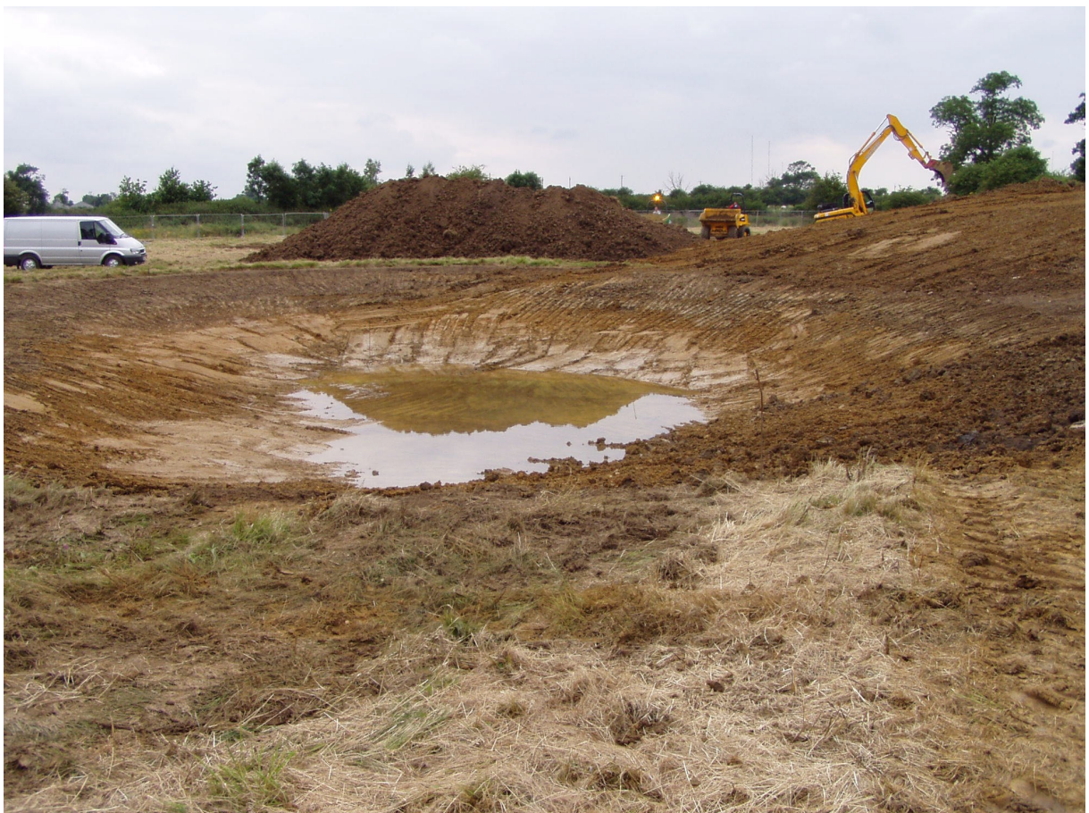
Plate 8: Excavated Pond 2, before laying the liner, viewed from the East.
