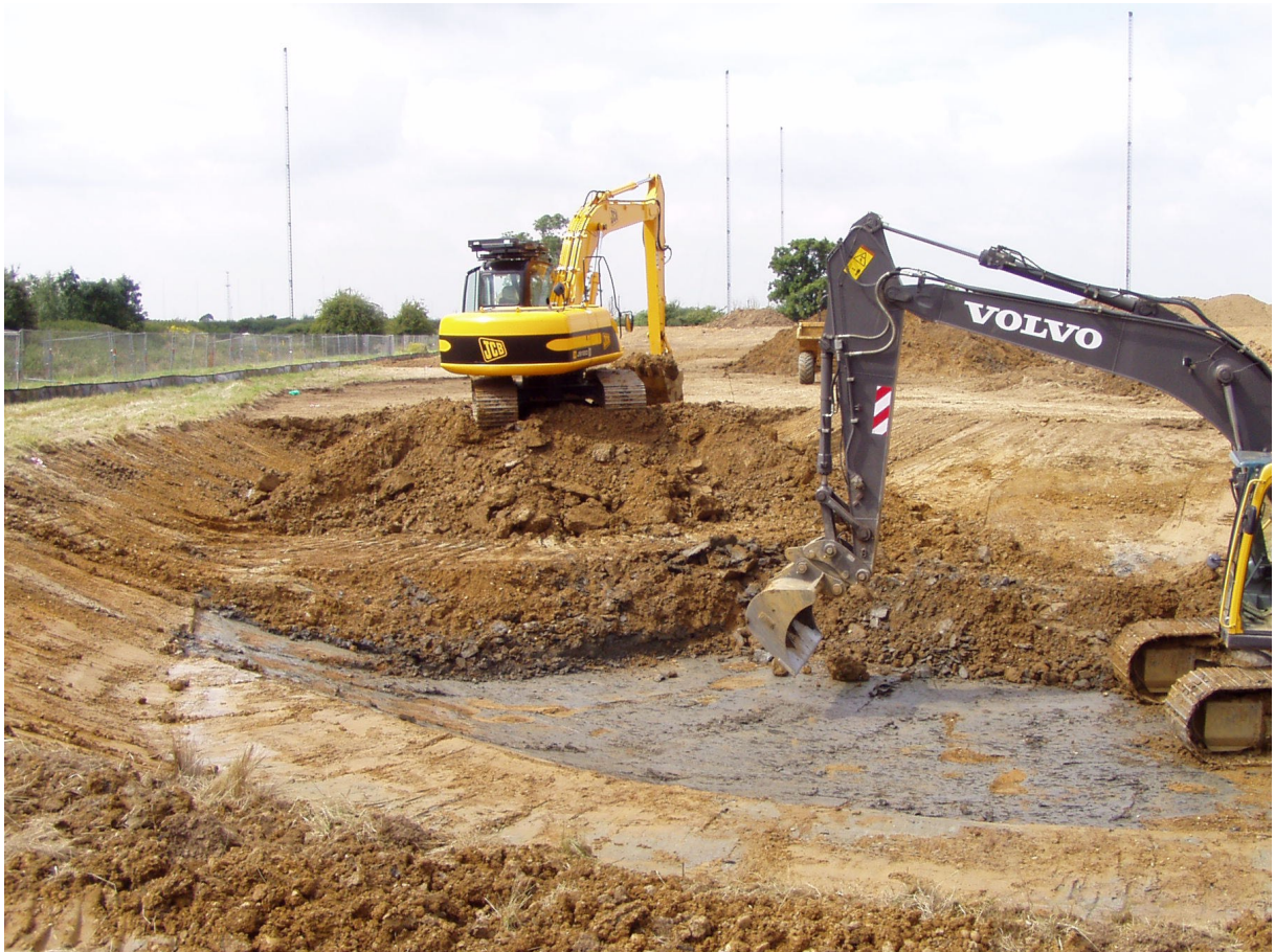
Plate 7: Excavation of Pond 4, viewed from the East.
