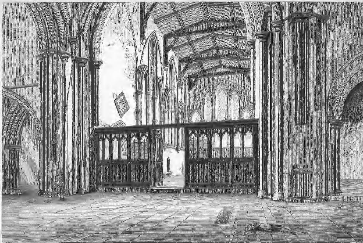
Interior of the Friary of St. John the Evangelist, formerly the Church of the Holywood.
