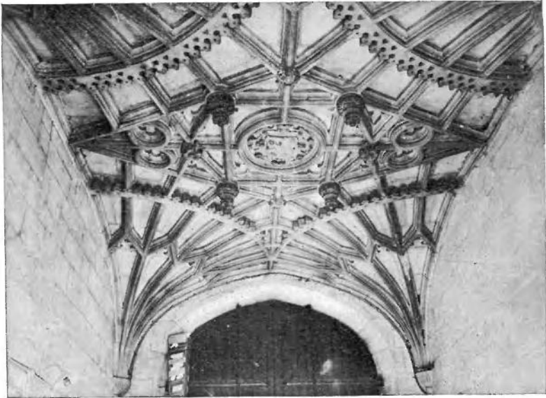
NO. 1. WADHAM COLLEGE, OXFORD. GATEWAY TOWER.
