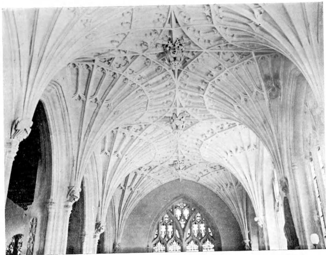
CULLOMPTON CHURCH, DEVON. LANE AISLE.
