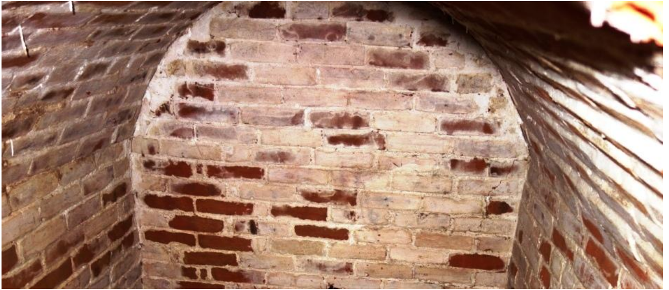
Plate 27. Interior of crypt showing barrel-vaulted ceiling, from the entrance (looking west)
