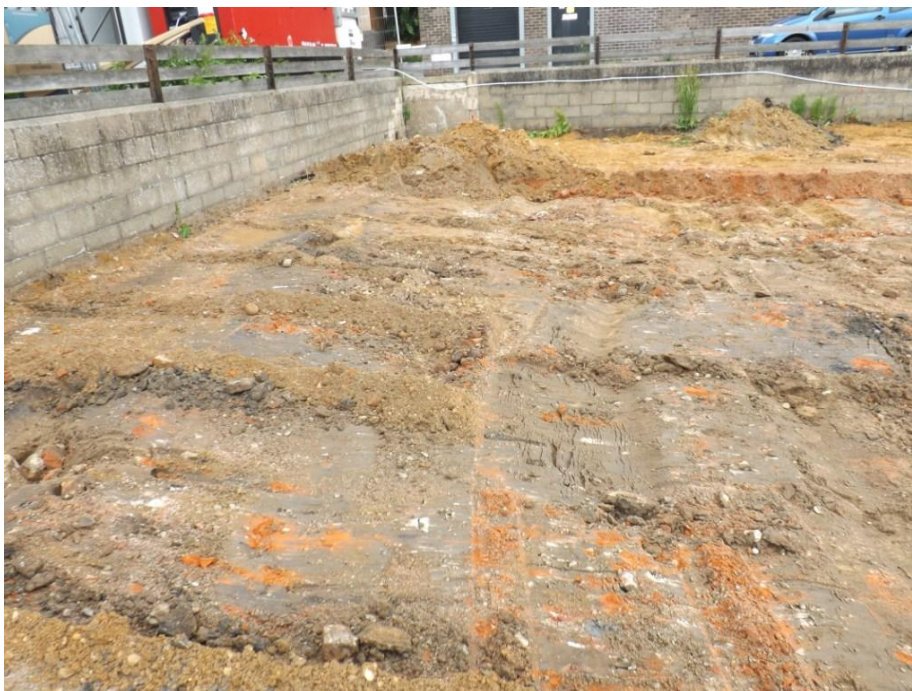
Plate 2. Site view during stripping, looking south-west
