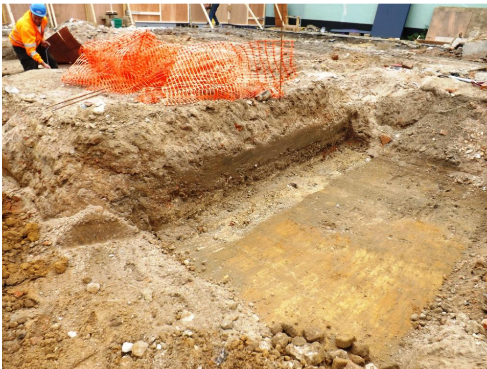
Plate 22. Area stripped to the back of the crypt showing extent
