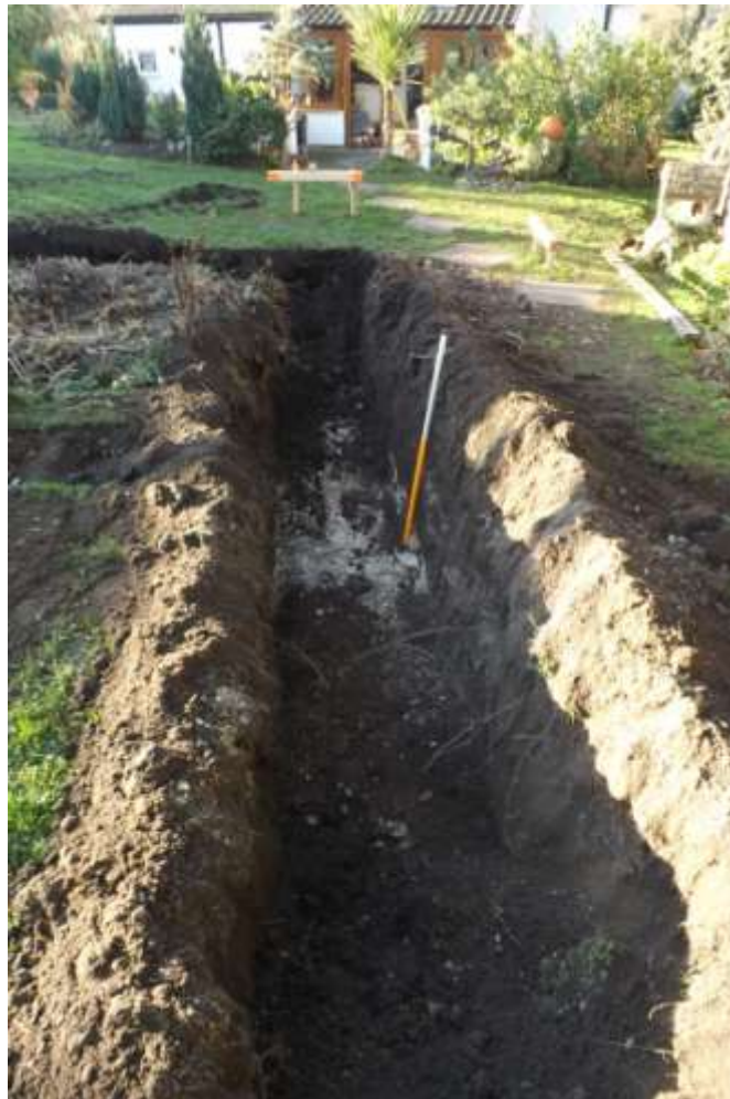
Plate 2. General view of foundation trench showing chalky natural
