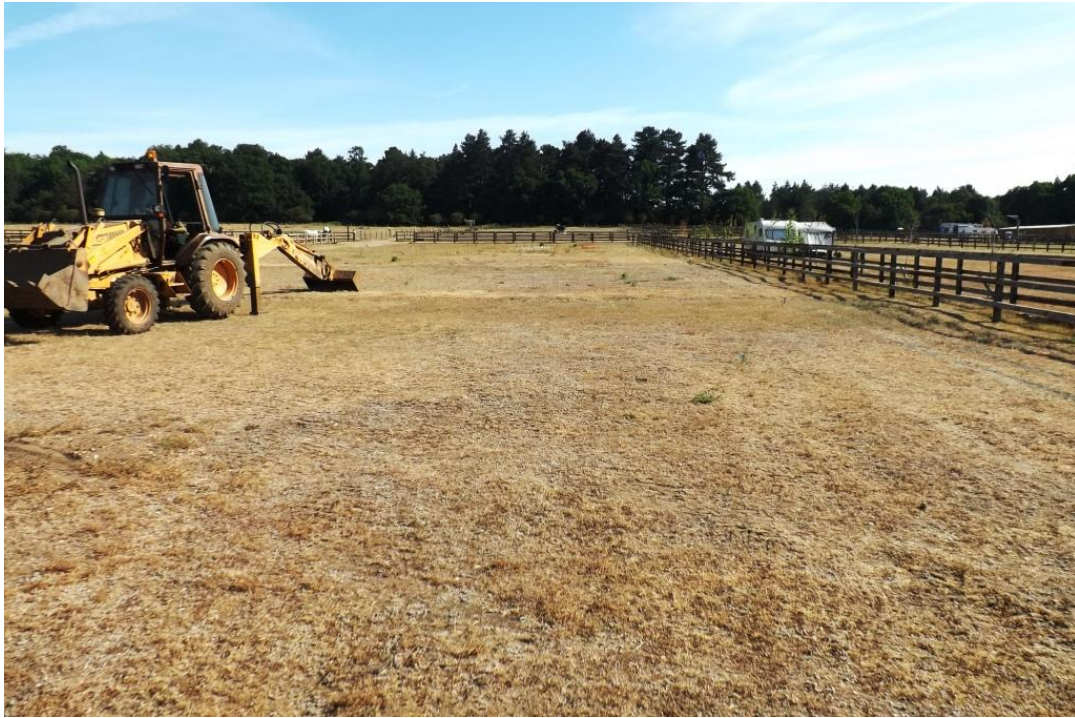
Plate 1. Pre-excavation of the log cabin site
