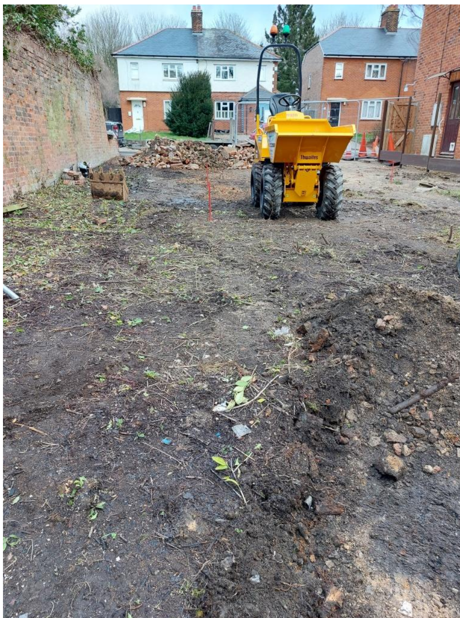
Plate 1. Pre-excavation - general view to the north
