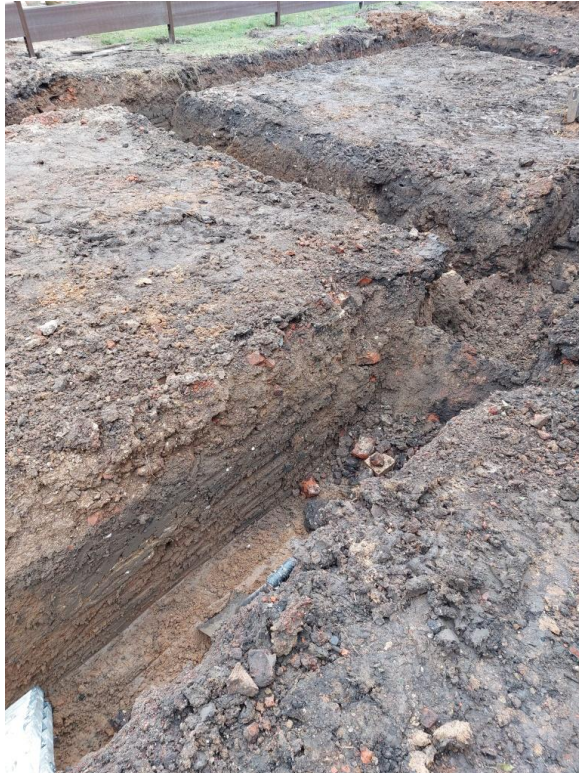
Plate 4. General view to the south-east across footings showing demolition layer (1000)
