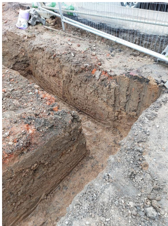
Plate 3. North-east corner of footing where demolition layer (1000) was absent (cbm seen is from last building demolished)
