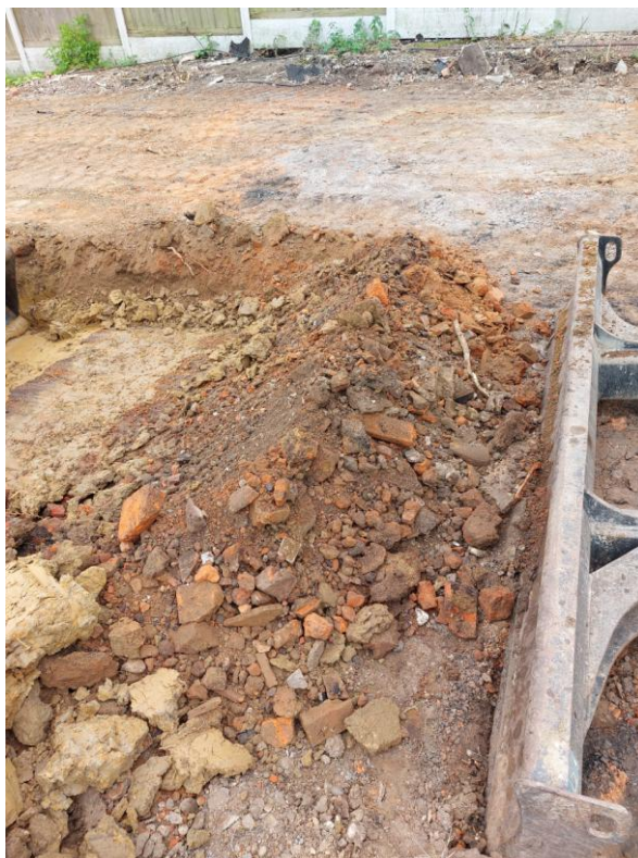
Plate 1. Mid-excavation of trench 4 site; note brick in demolition layer
