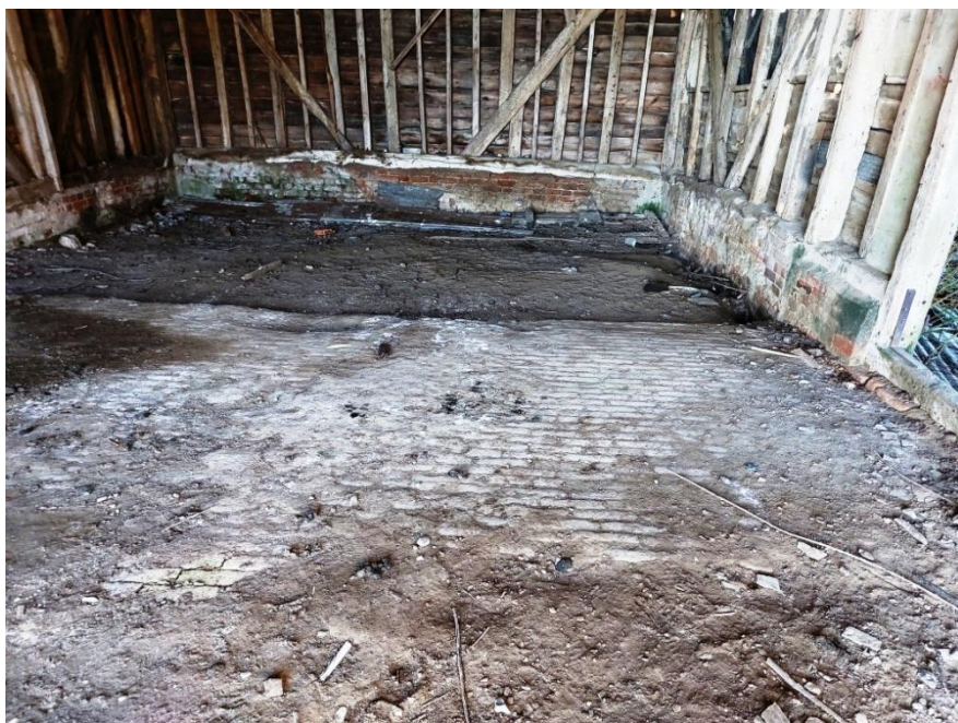
Plate 18. Threshing floor
