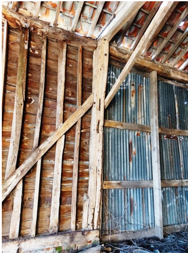
Plate 15. Vacant mortise and tenon joint on storey post of south wall
