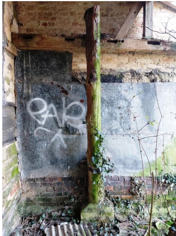
Plate 29. Lean-to support post with iron tie
