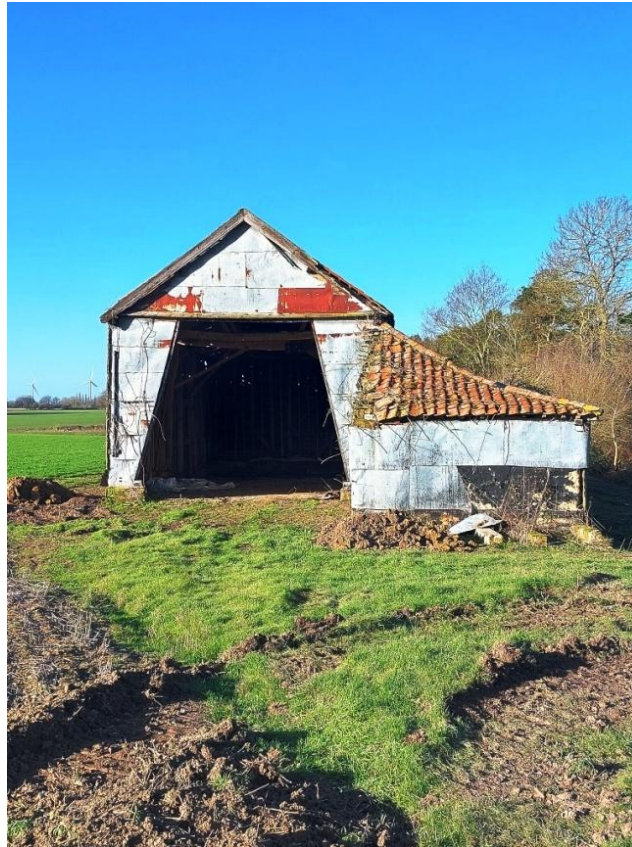
Plate 1. Barn general view from the north-east
