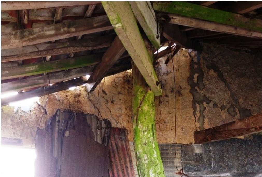
Plate 40. Clay lump wall on east gable end of lean-to (interior)
