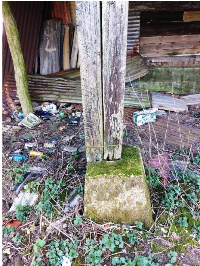
Plate 34. Detail of post base in concrete
