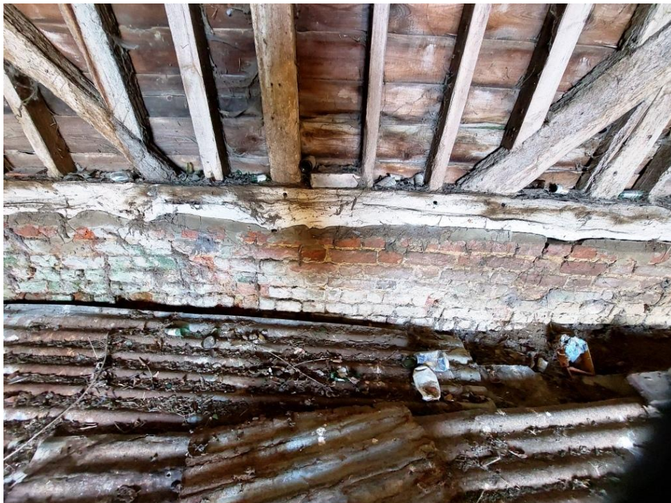
Plate 22. Brick plinth detail
