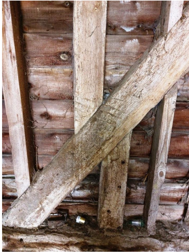
Plate 35. Carpenters marks example throughout barn
