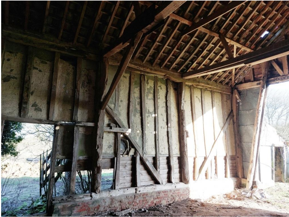
Plate 12. Framing detail in north wall
