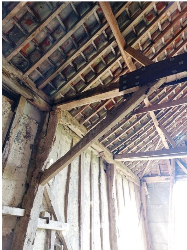
Plate 13. Original post with modern brace and tie beam detail
