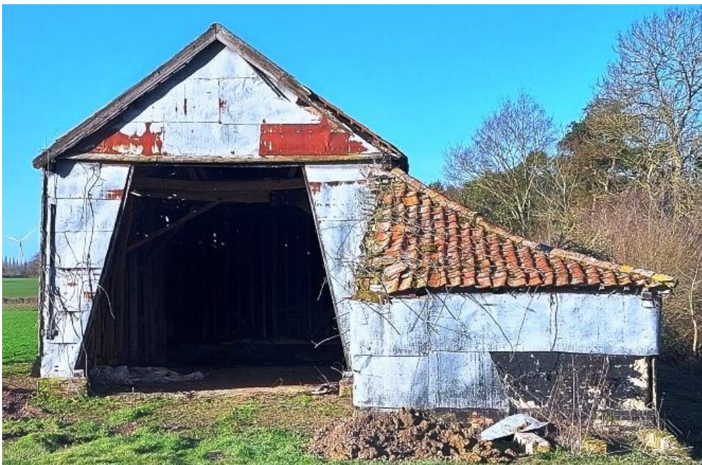
Plate 2. Side elevation view, from the north-east
