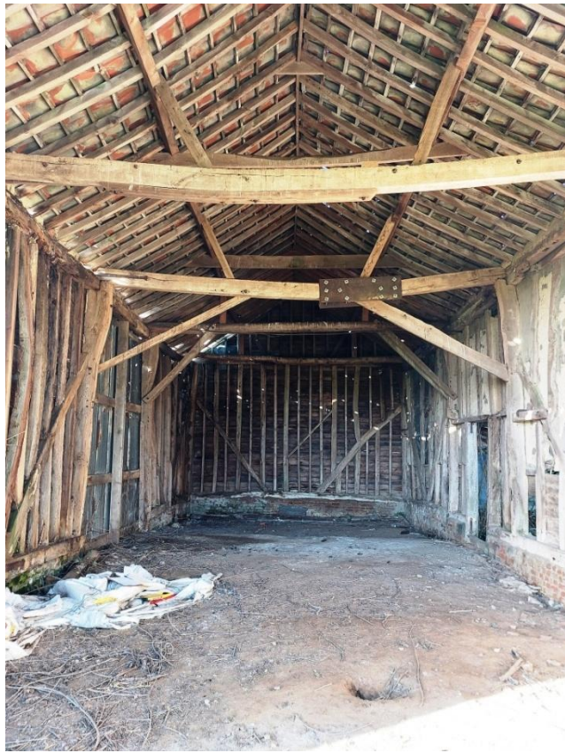
Plate 7. View into barn. from the east
