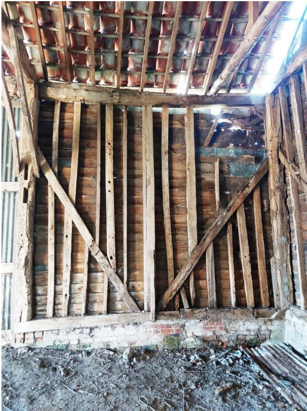
Plate 9. Timber-frame detail on south elevation wall
