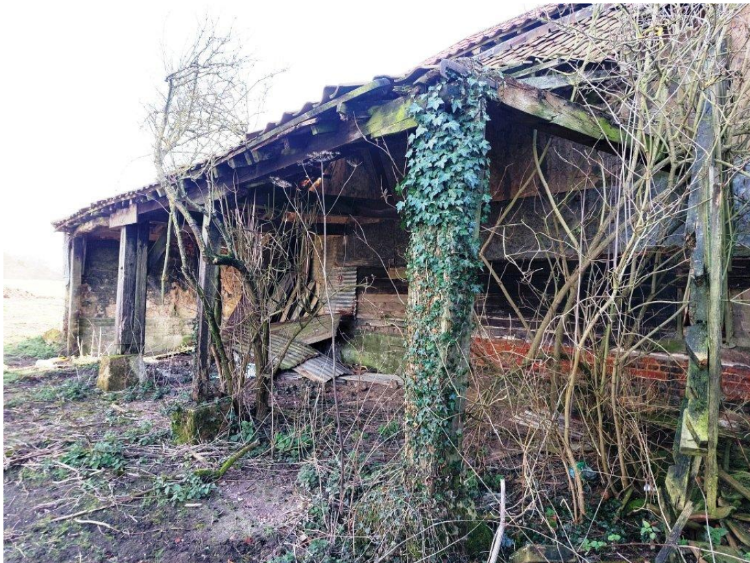
Plate 30. General view of lean-to, from the north-west
