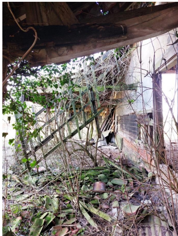
Plate 28. View through lean-to (roof timbers)
