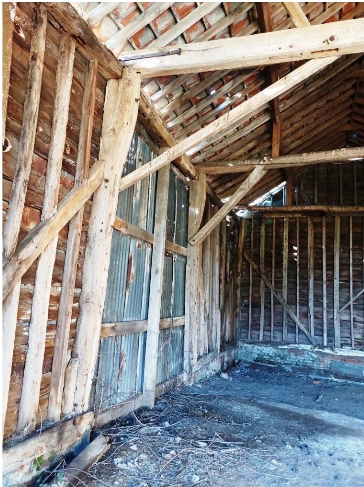
Plate 17 . Splayed post detail
