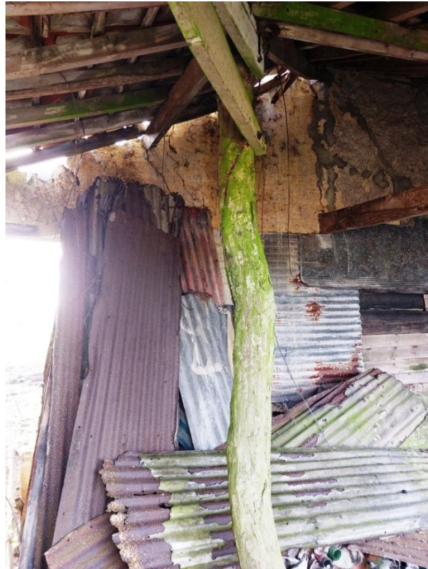
Plate 25. Rustic post supporting lean-to roof
