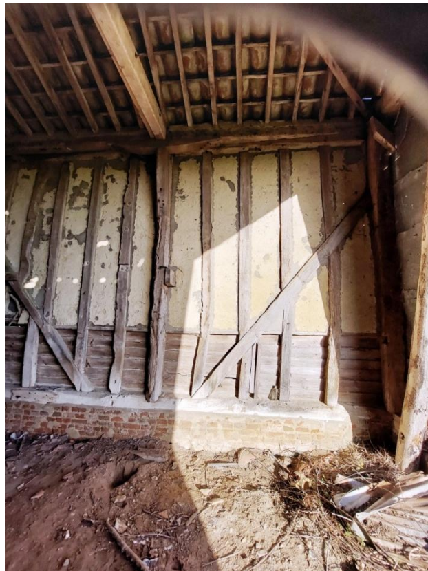
Plate 20 .Wall infill of wattle and daub with weatherboarding below
