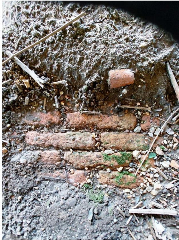
Plate 19. Brick detail in threshing floor
