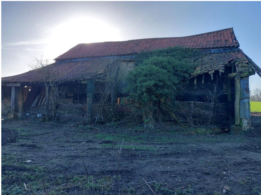
Plate 6. View of lean-to, from the north
