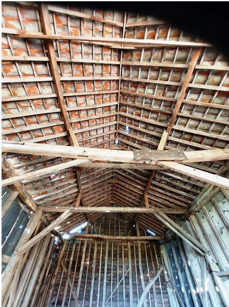
Plate 23. Later roof detail
