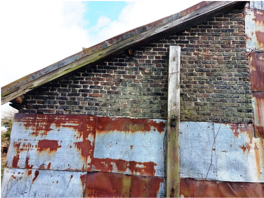
Plate 33. Brick gable (coarse Flemish bond) end wall to lean-to (west-facing)
