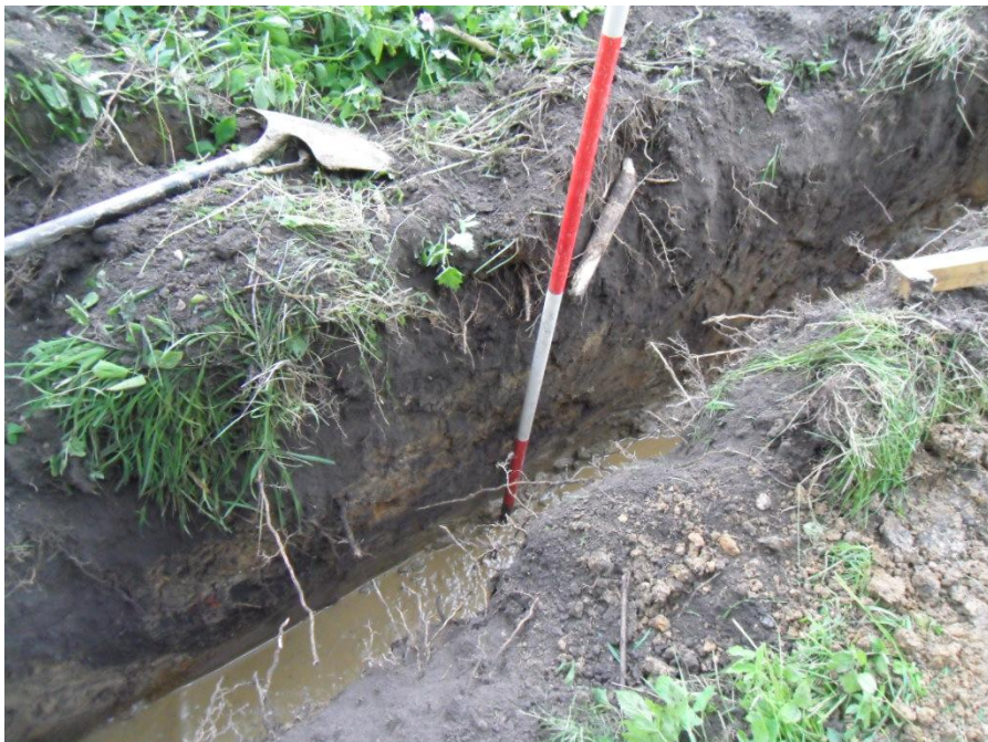
Plate 23. Drainage trench at the rear of the house, looking north
