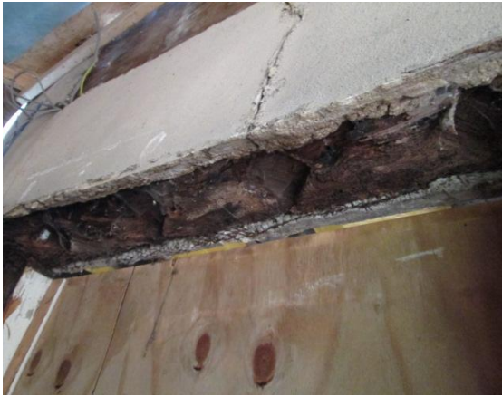
Plate 3. mullioned window sockets in lintel From the rear of the house
