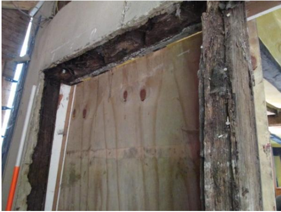
Plate 1. Re-sited window frame with moulding reversed
