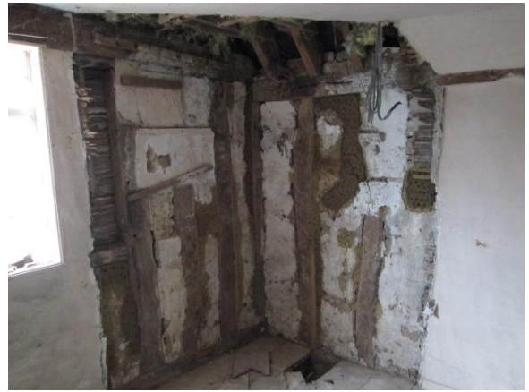
Plate 4. Truncated storey post- possible sites of window apertures
