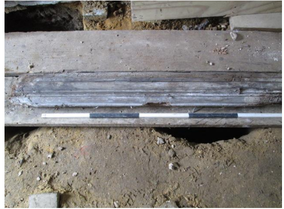
Plate 2. Re-sited window frame removed (showing moulding)
