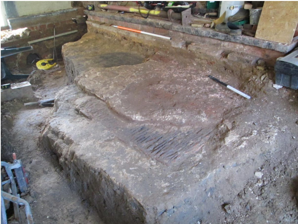
Plate 9. The open hearth (018) with first over-burden removed, showing the tiled hearth with brick and mortar layer (016) and fired earth layer (017) above, with charcoal-stained earth (020) behind; in the background, the much truncated structure (021, all revealed upon the made-up layer (004)
