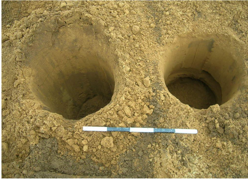
Plate 1. Sample of post holes excavated for the PV system
