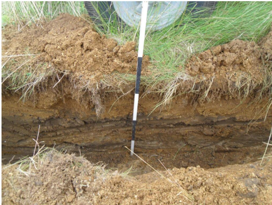
Plate 4. Cable trench showing re-deposited material
