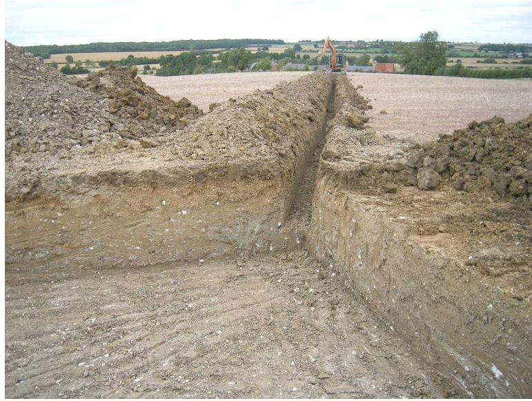
Plate 3. The cable trench running from the turbine base to the farm to the north, viewed from the south
