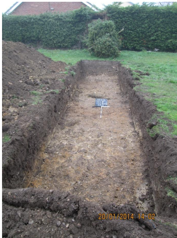
Plate 4. Post Excavation, Trench 3 from the south
