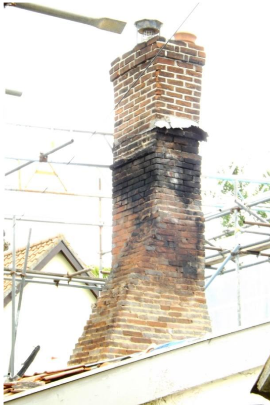
Plate 16. Chimney stack as revealed
