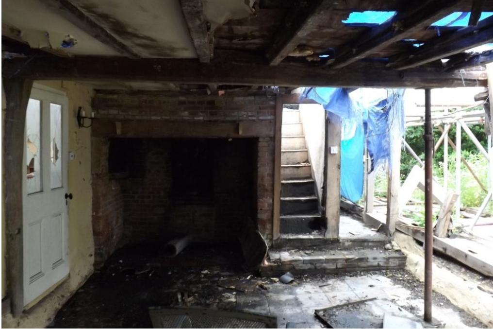
Plate 7. The hall towards the fireplace
