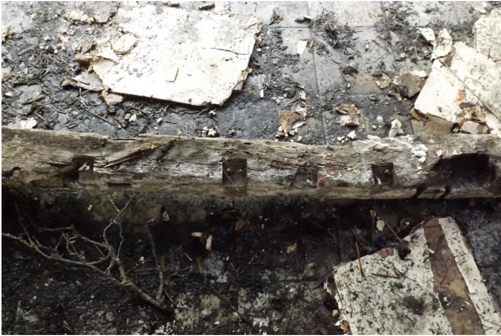
Plate 21. The wall plate (as removed)
