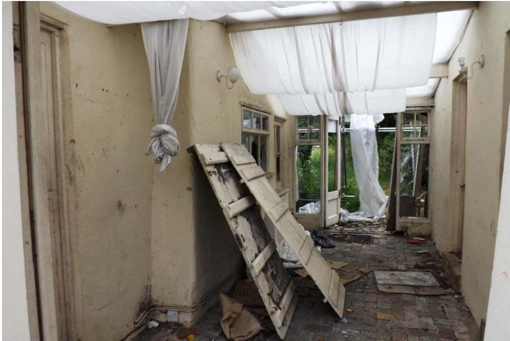
Plate 17. The end gable wall to the left through modern connecting passage
