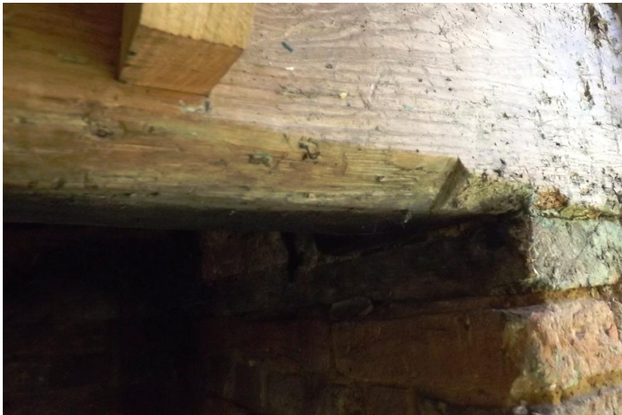
Plate24. Fireplace bressummer beam chamfer and stop detail in the hall
