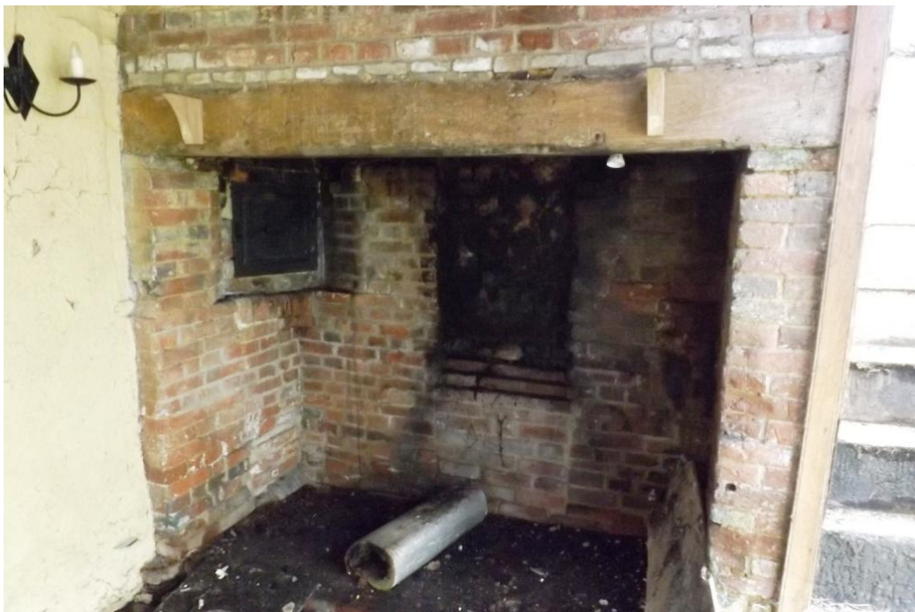
Plate 8. Fireplace in the hall
