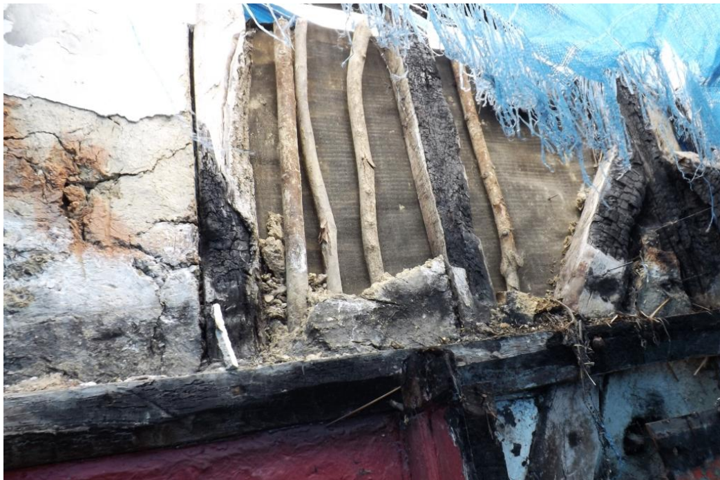
Plate 20. Wattle and daub wall fabric as revealed in the parlour
