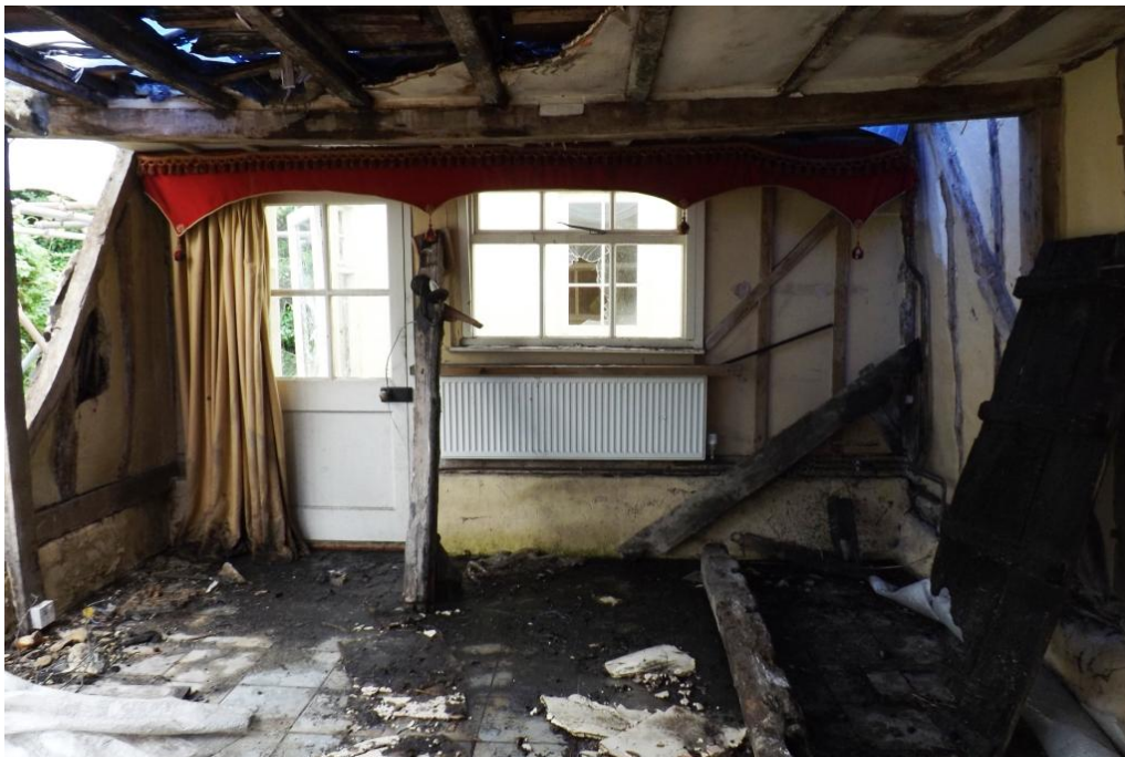
Plate 10. Hall through to open up service room
