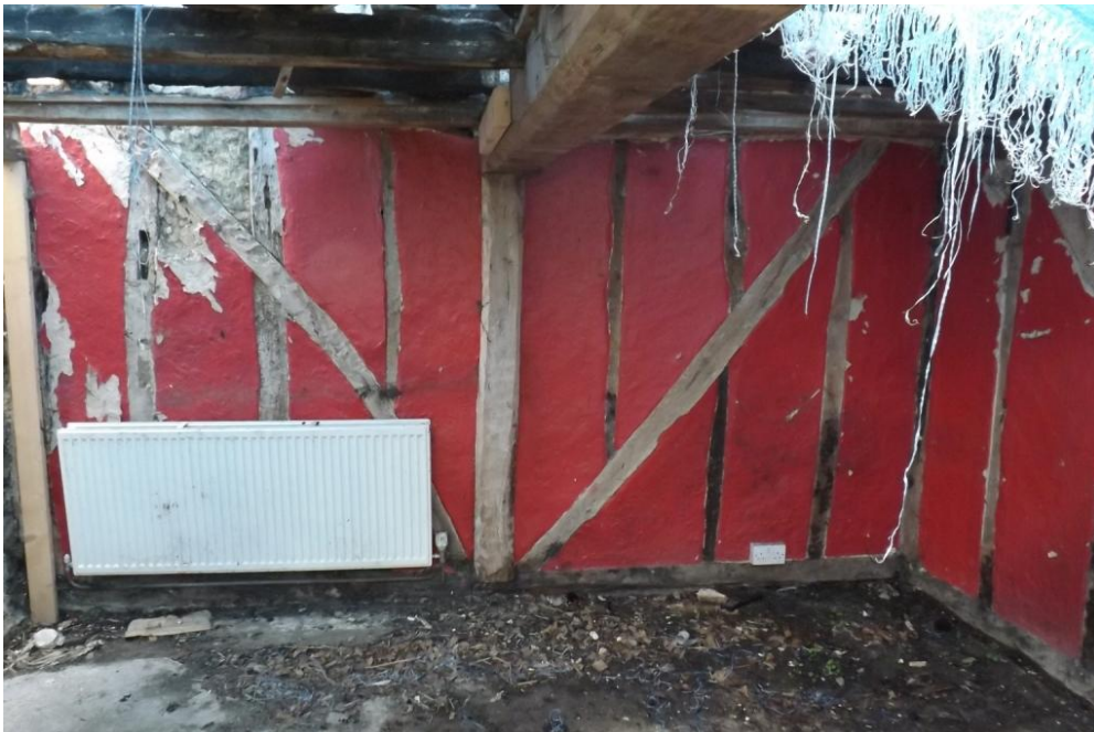
Plate 4 . Parlour wall studwork detail
