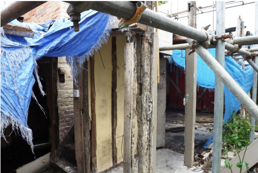
Plate 18. Lobby entrance (front)
