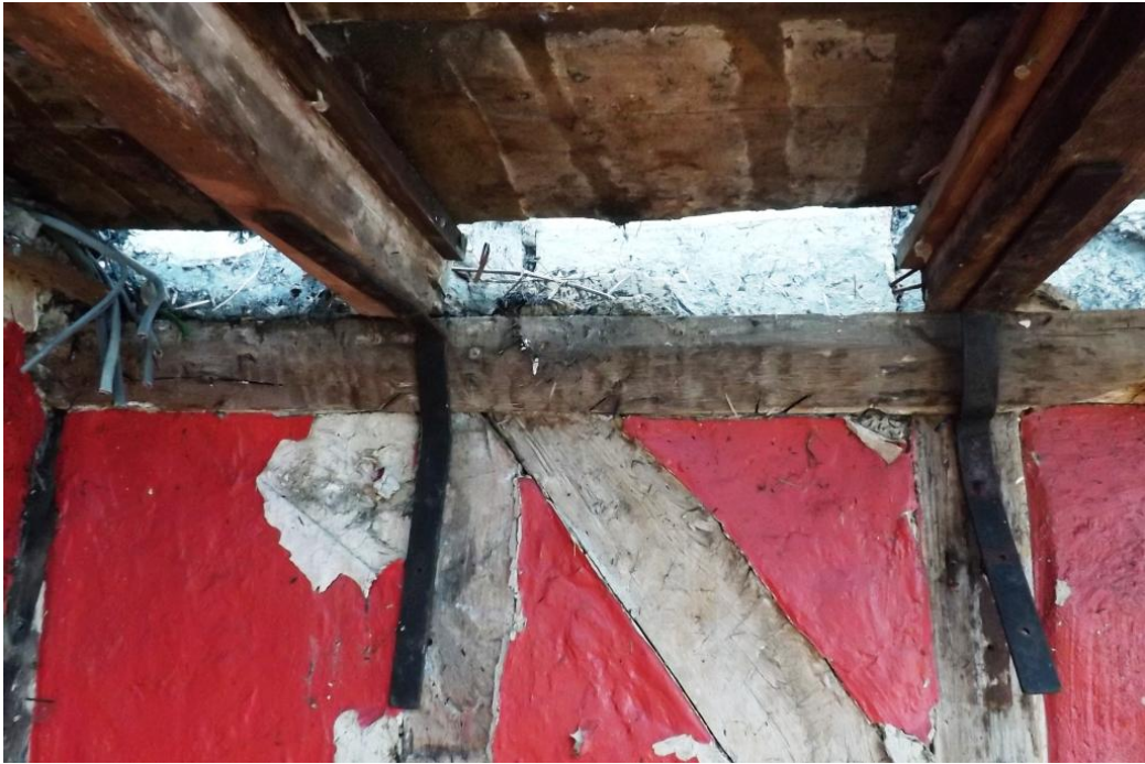
Plate19. Detail of clamp supporting upper floor in parlour gable end wall
