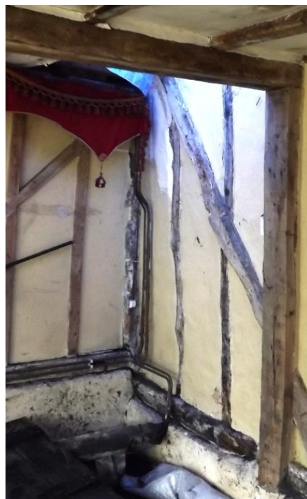
Plate 14. Detail of storey post and joist support at service room division
