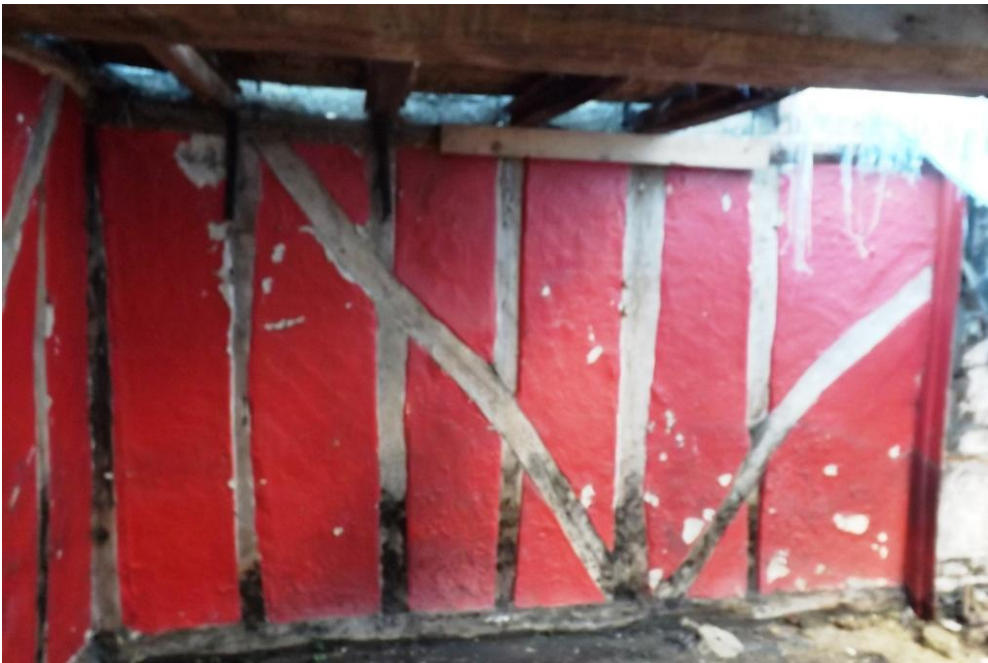
Plate 2. Parlour end gable wall studwork
