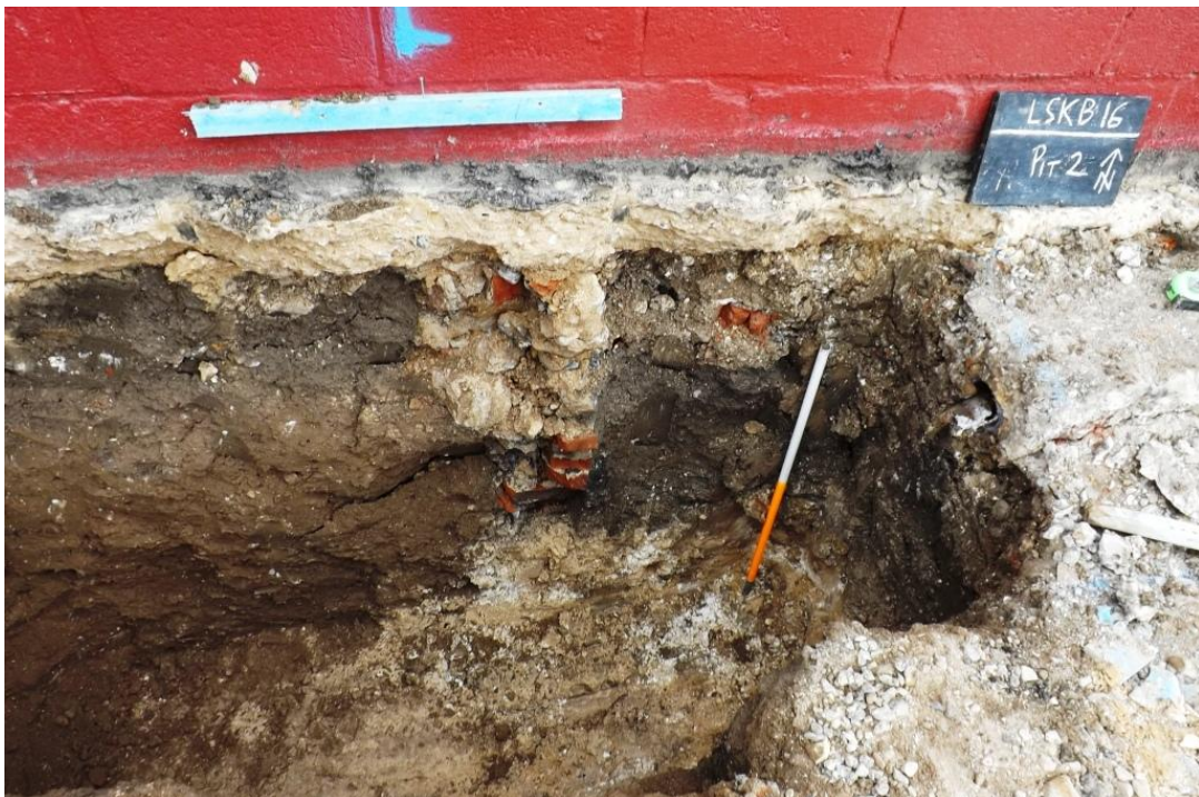
Plate 7. Tr 2. Showing footing (1002) below auction rooms, from the north-east
