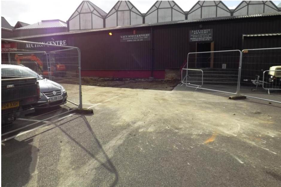
Plate 1. Pre-excavation, general site view from the north
