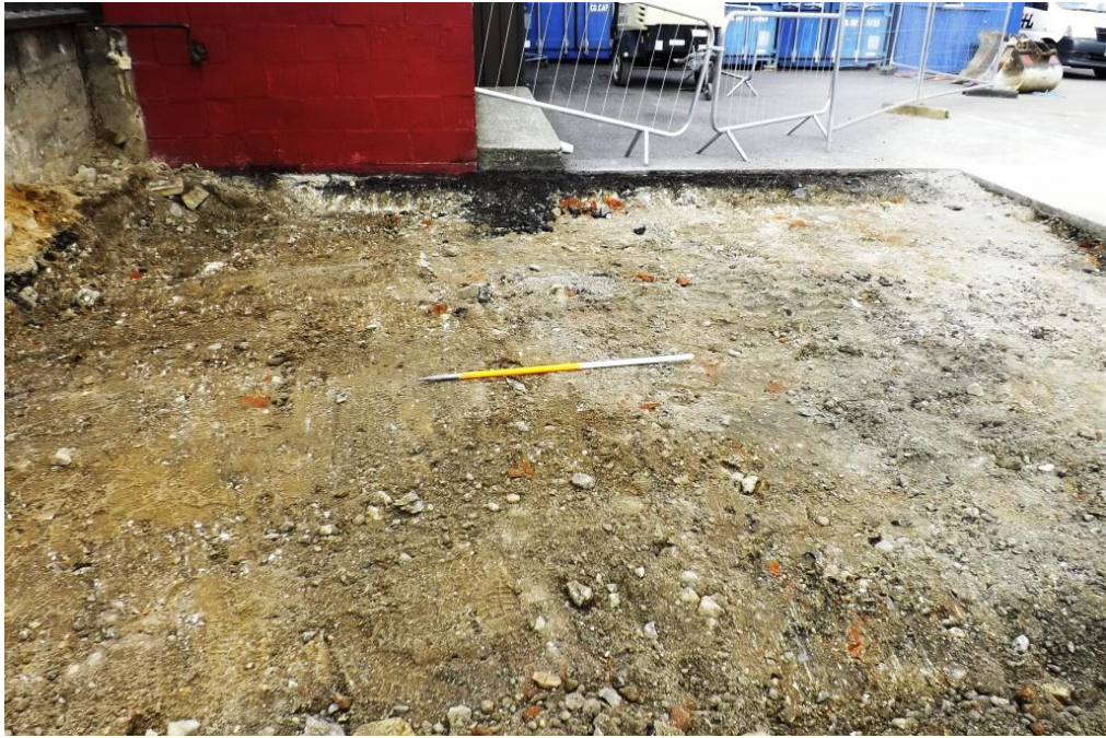
Plate 5. part of development area after surfaces removal
