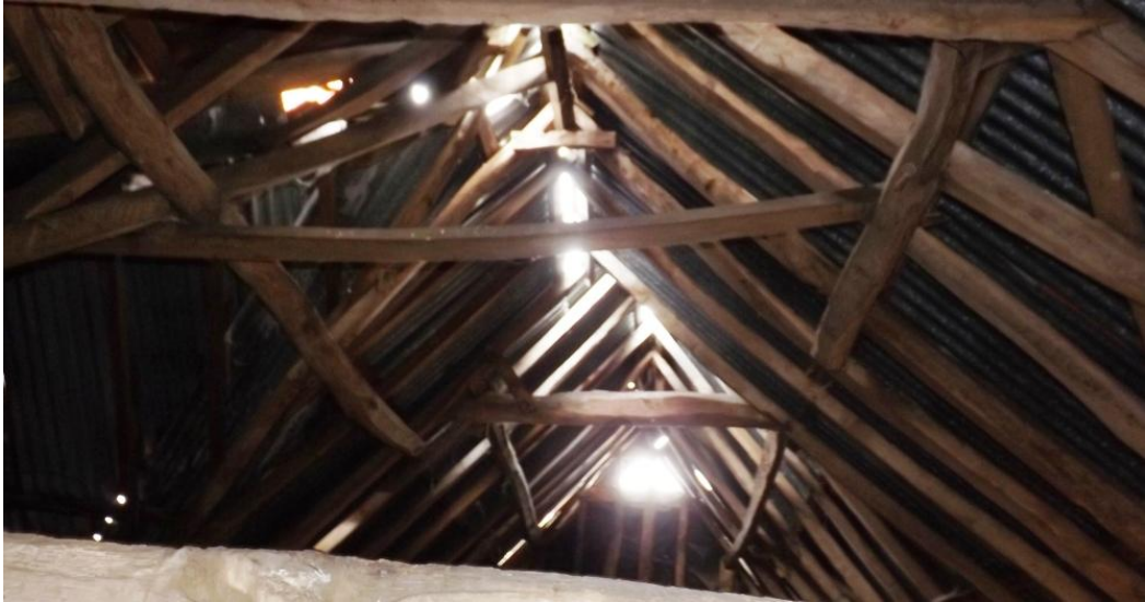
Plate 18. Roof detail under higher section of roof
