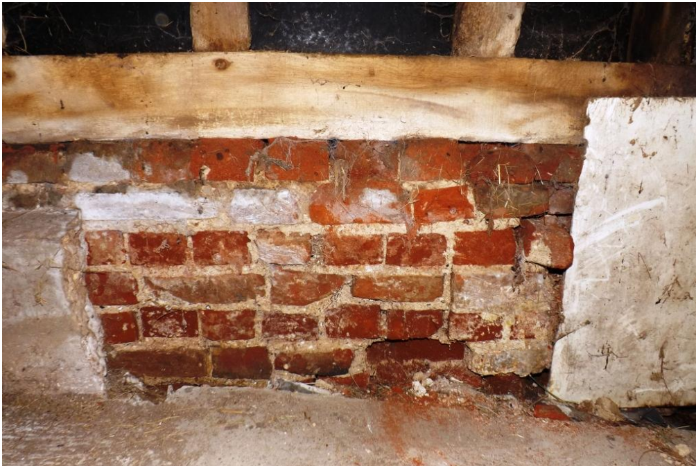
Plate 29. Brick plinth detail showing English Bond coursework in red brick (shot 31)
