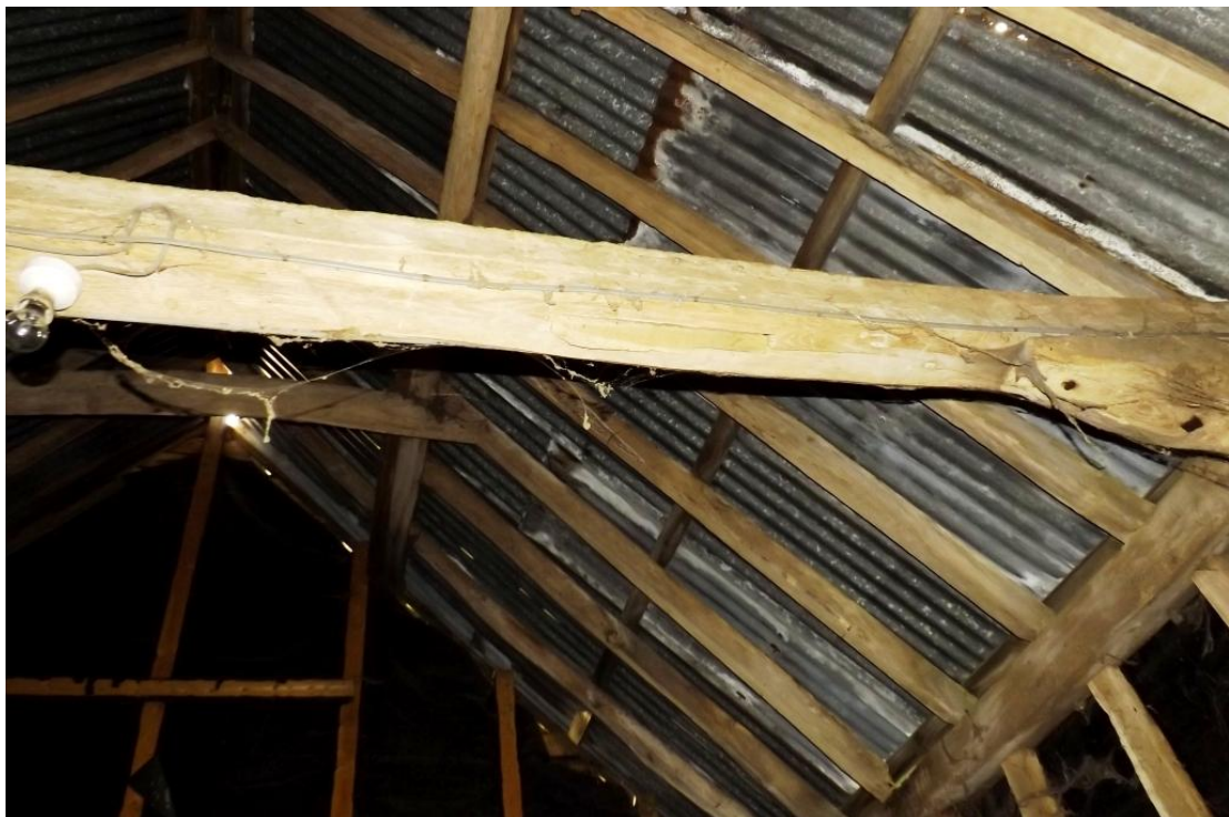
Plate 11. Blind tenon in tie beam for the earlier arched brace
