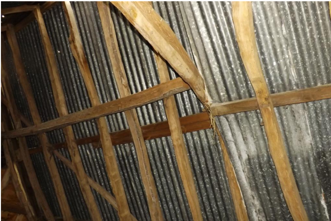
Plate 23. Lowered roof detail at the join with the higher section-west-facing
