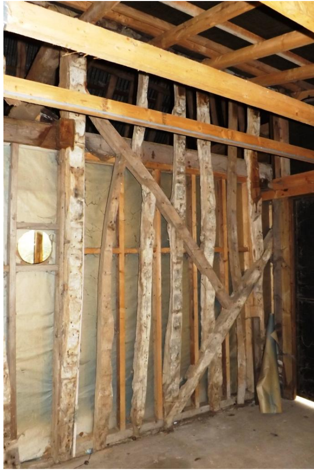
Plate 14. Original studwork to the porch (originally the outer wall)
