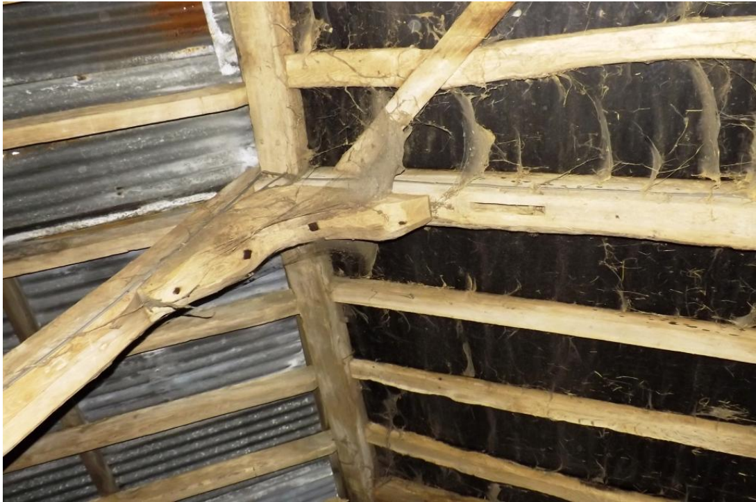
Plate 10. Bolted knee brace (early 19th c.) between bays 1 & 2
