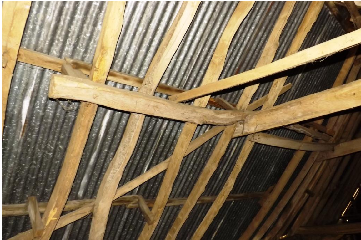
Plate 24. Roof detail under high section of roof (north-west section)
