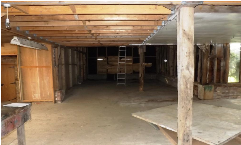
Plate 5. Interior view from the north
