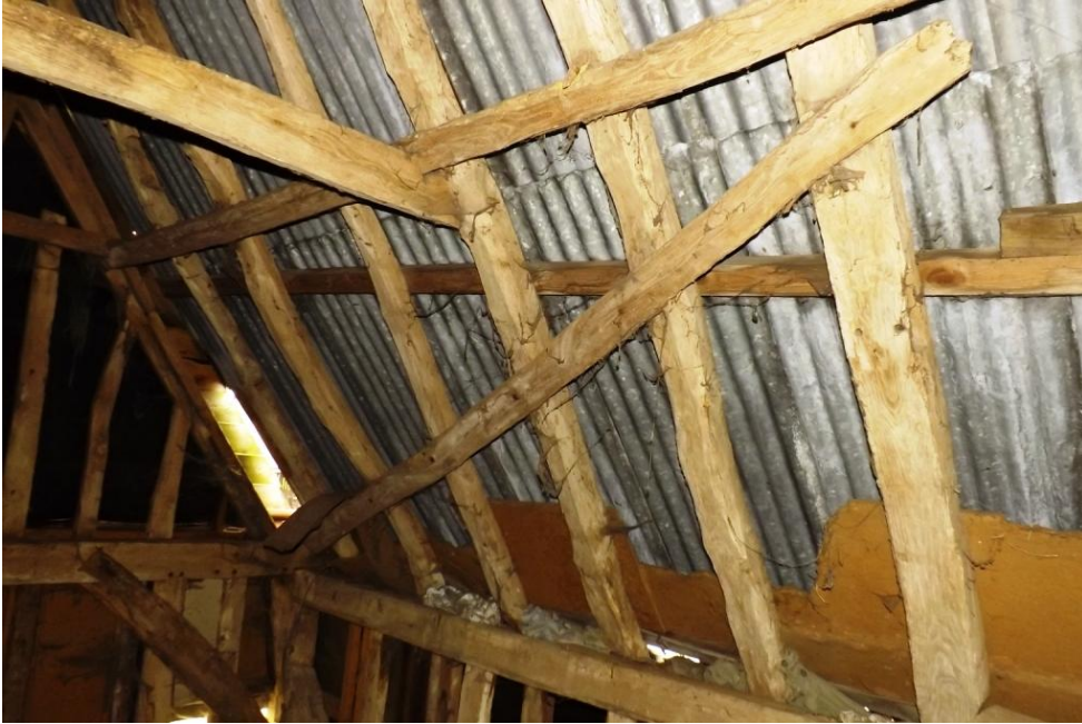
Plate 20. Roof construction showing diagonal wind brace and butt purlins under bay 4
