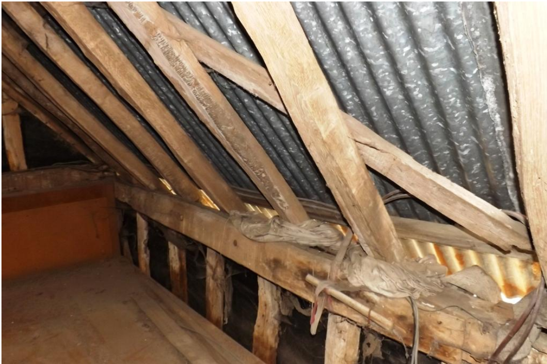
Plate 27, Undisturbed, correctly placed rafters under high section of roof
