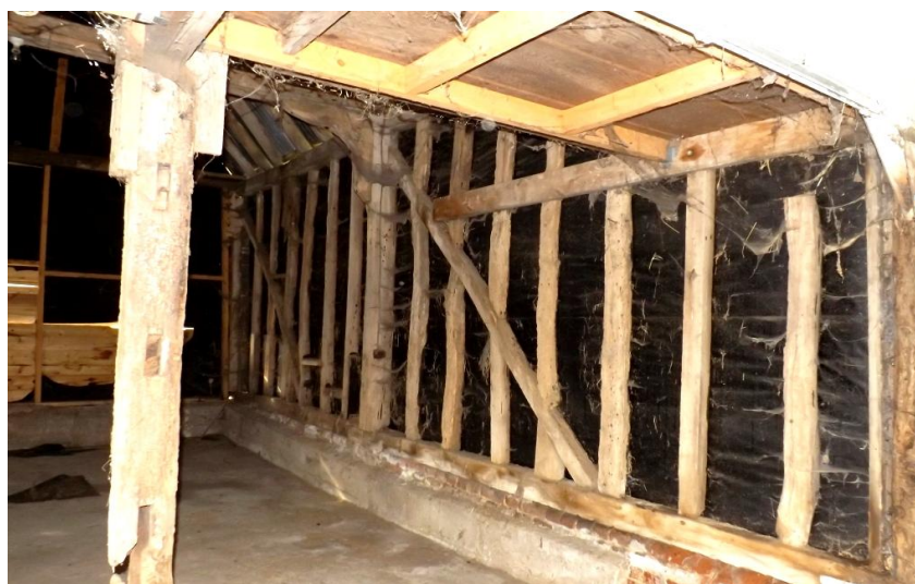
Plate 9. Original studwork on west-facing elevation wall
