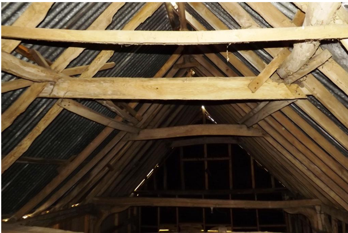
Plate 25. Roof truss detail looking south under lowered section of roof
