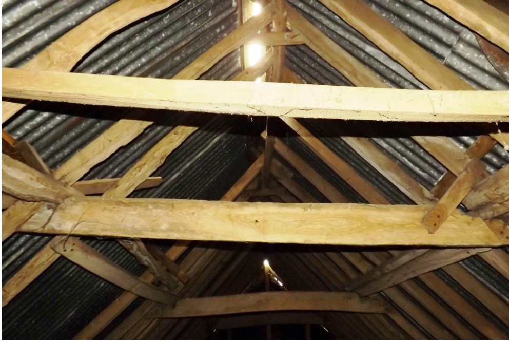
Plate 28. Collars over bays 3-4, peg jointed with nailed strengtheners
