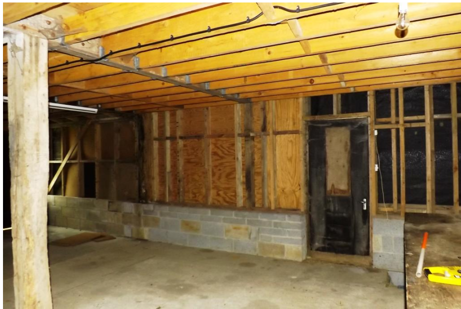
Plate 15. South gable end wall interior (replaced work)
