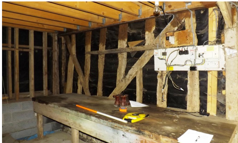
Plate 8. Original studwork on east-facing elevation wall interior
