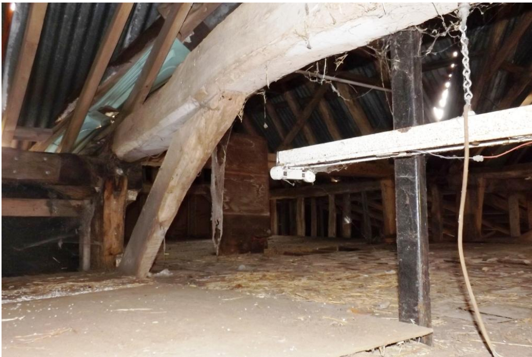
Plate 17. Tie beam and arched brace between bays 2 & 3
