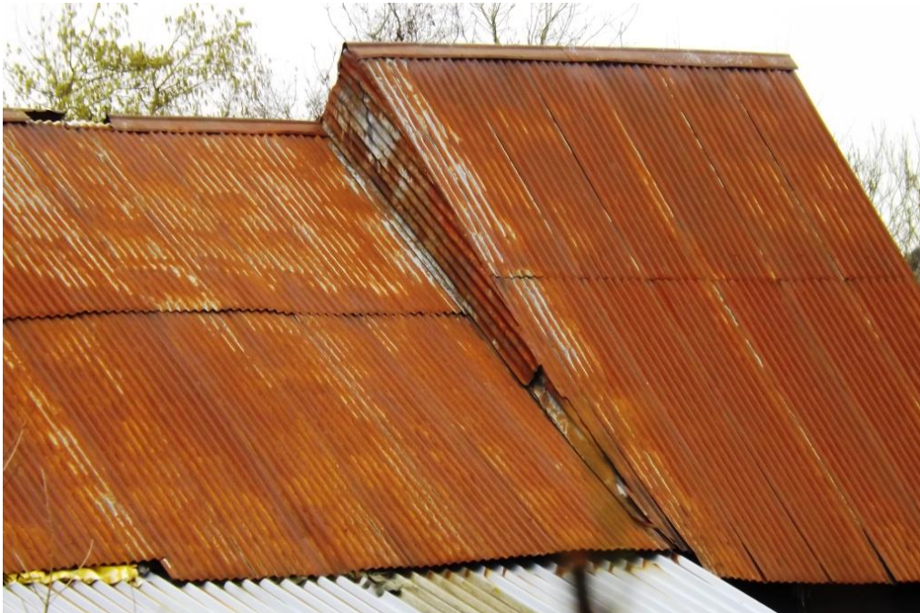
Plate 31 Roof detail showing original height (high end and the altered lower end, from the road (shot 33))
