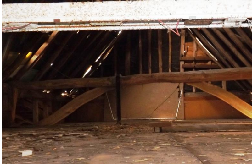
Plate 16. Tie beam with original arched braces between bays 3 & 4
