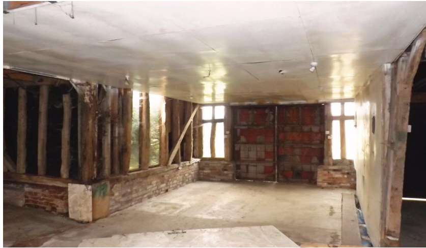
Plate 7. Interior towards the porch from the east
