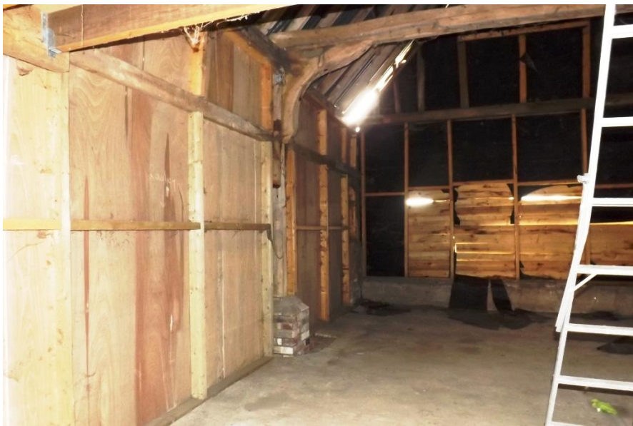
Plate 13. Replaced wall section to east elevation and south gable end
