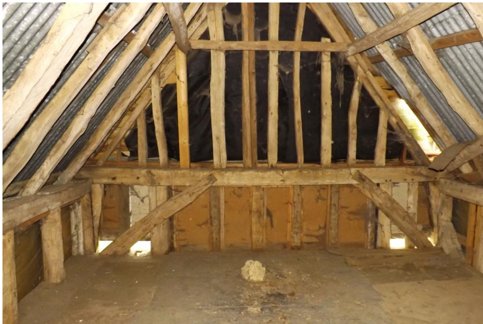
Plate 21. Gable end studwork detail; corner posts with arched bracing
