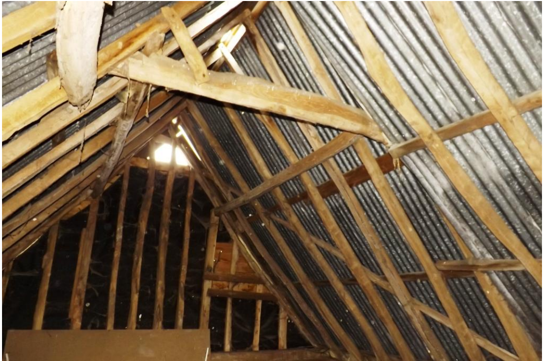
Plate 22. Roof detail between high and low sections, looking north
